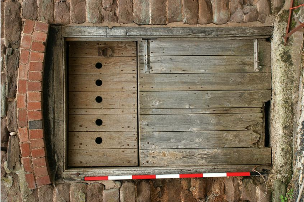
Plate 7 East elevation doorway
