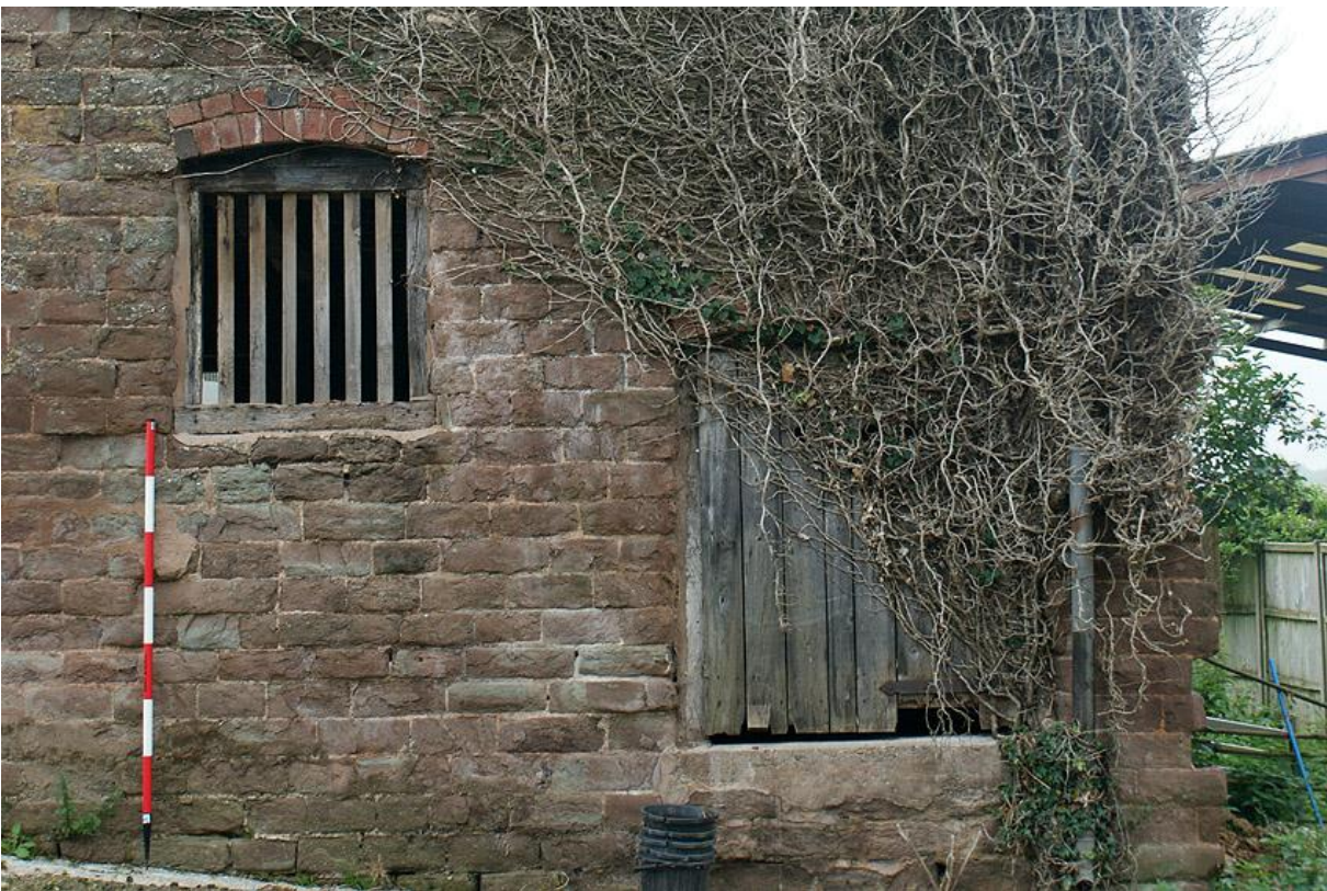
Plate 29 Blocked northern stable door and window on east elevation
