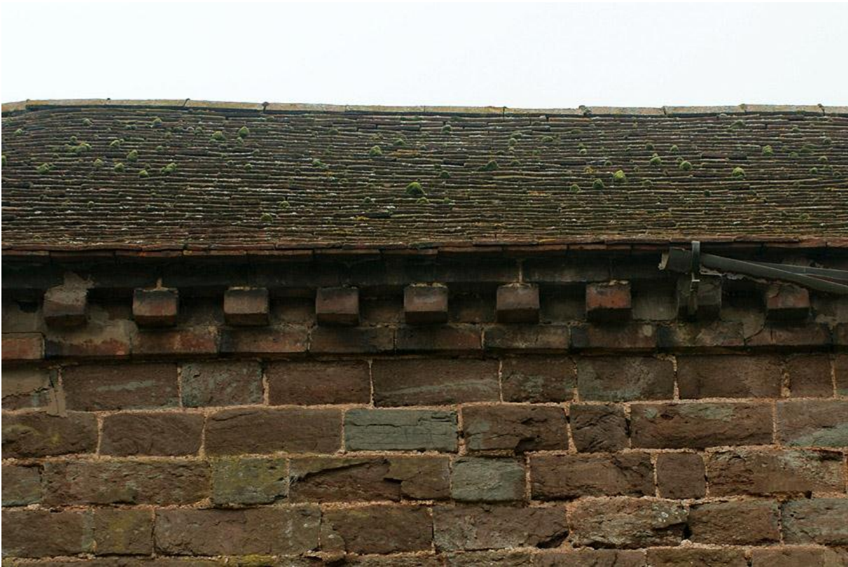
Plate 5 The dentilated brick eaves cornice on the east elevation
