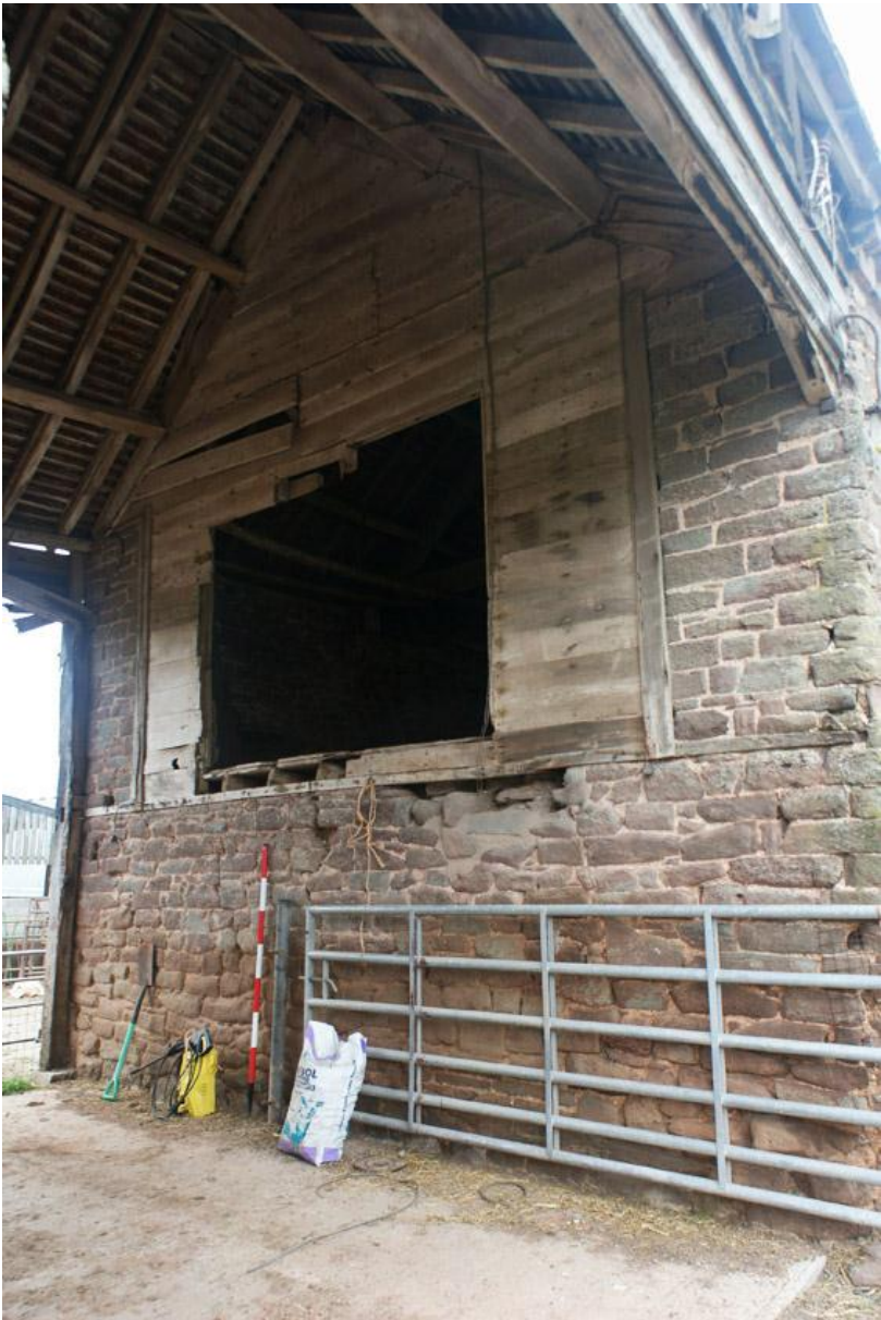
Plate 19 South gable from the south east
