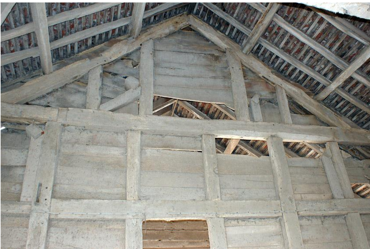
Plate 27 Interior of timber-frame barn where recorded building was attached
