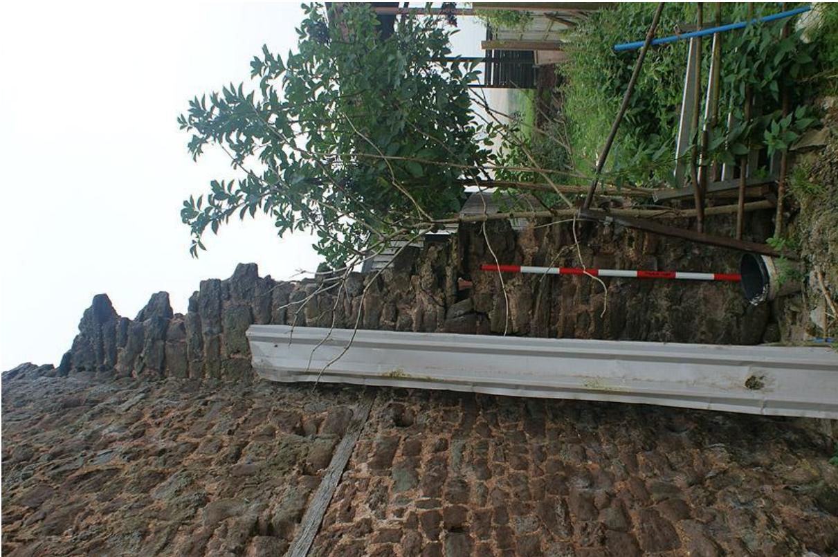
Plate 11 North elevation, west stub wall
