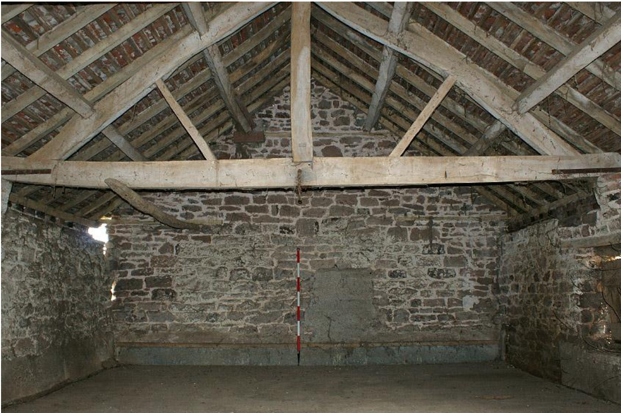
Plate 22 First floor interior
