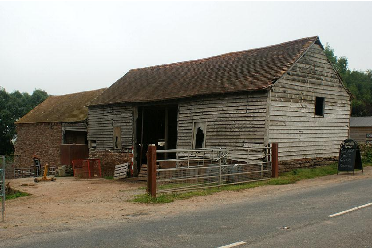
Plate 2 The barn from south west
