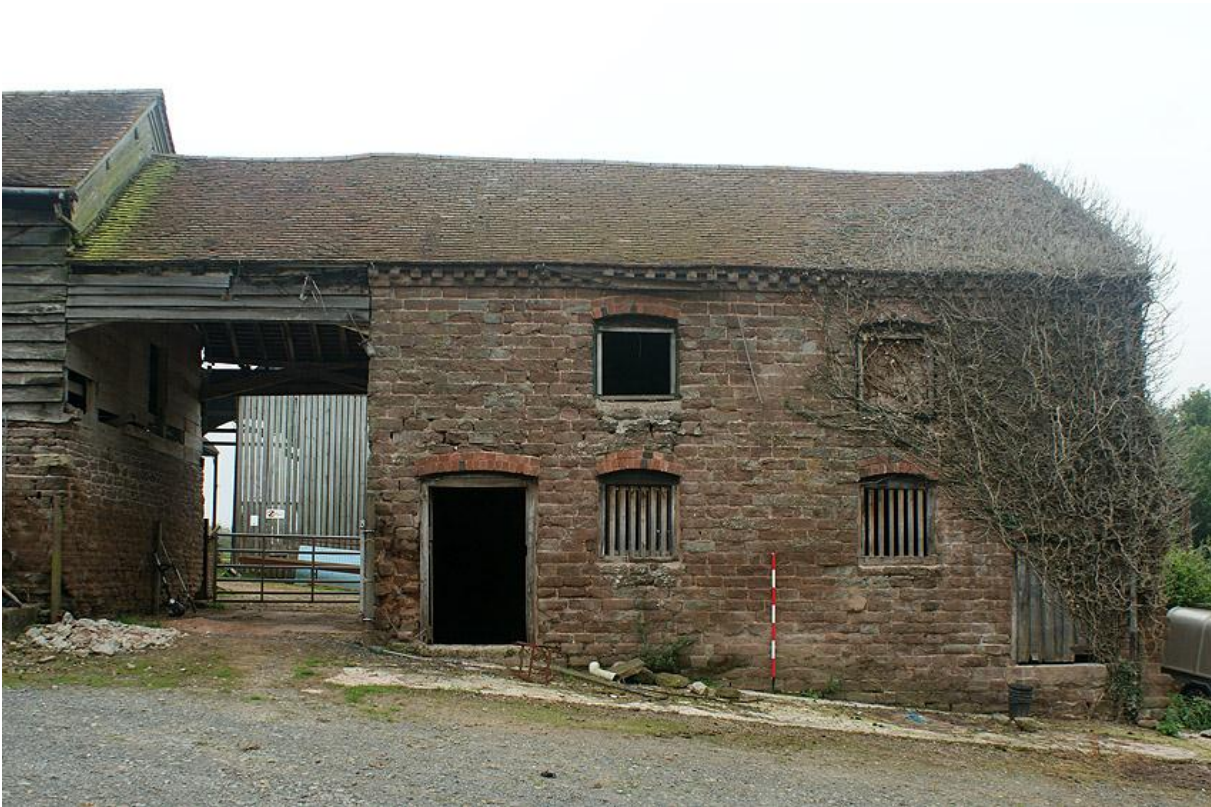
Plate 3 The barn from the east
