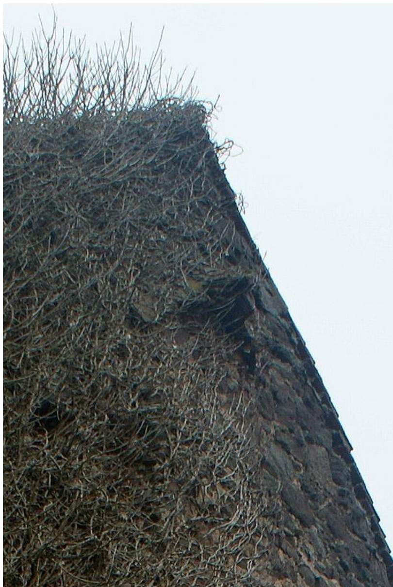
Plate 14 Remains of adjoining roof on north elevation
