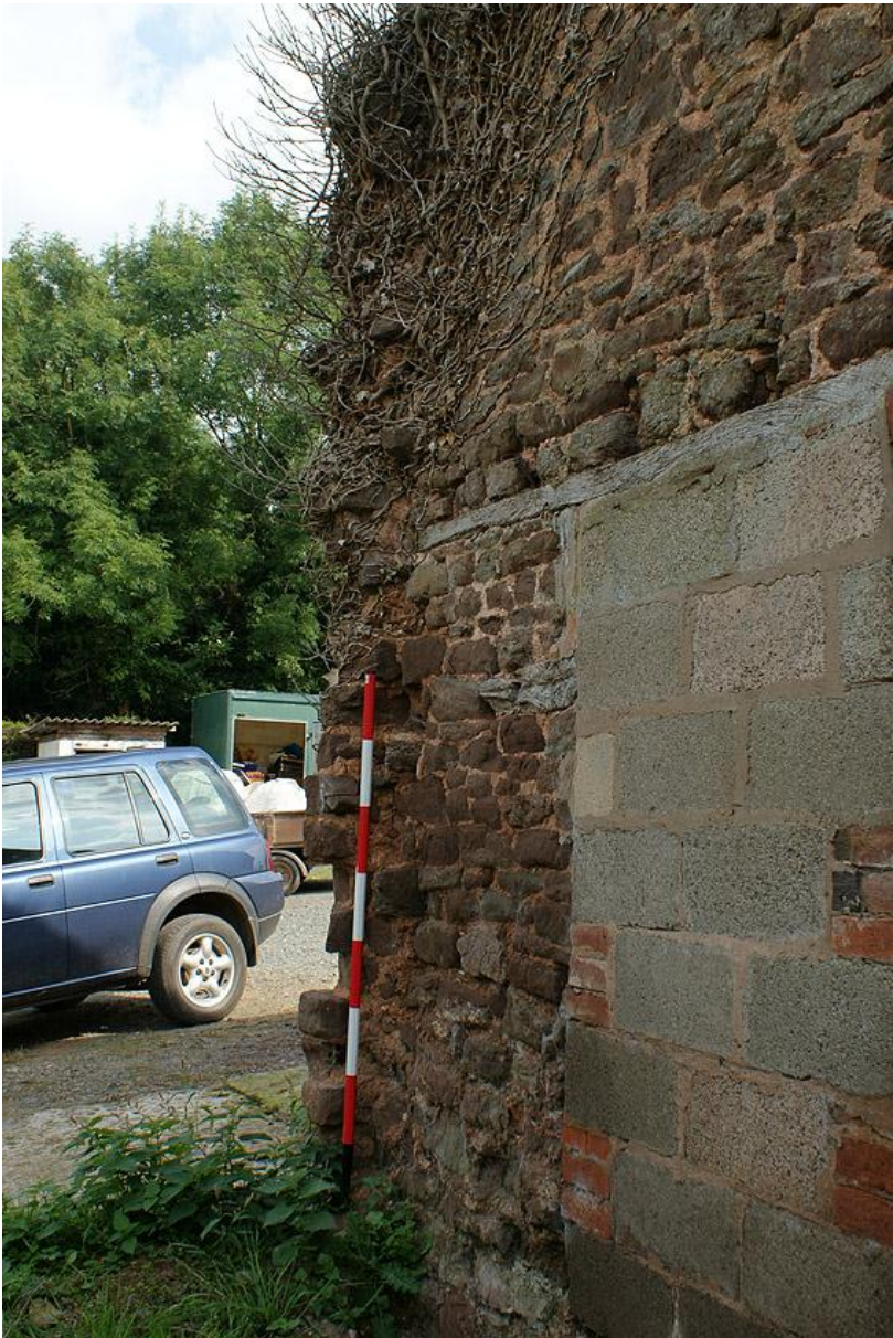
Plate 10 North elevation, east stub wall
