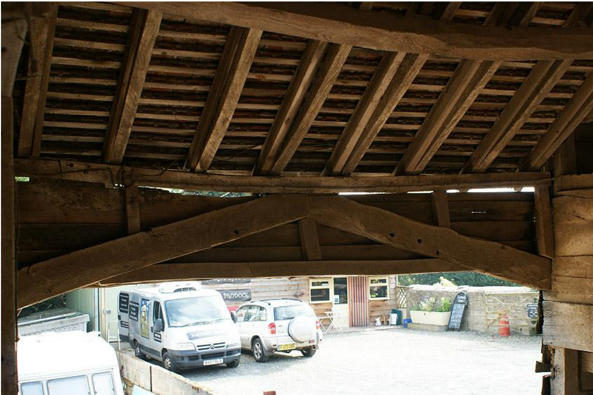
Plate 24 Internal frame of access way
