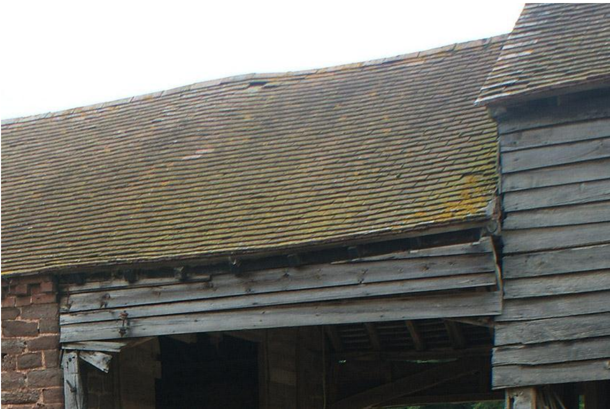
Plate 25 External weather-boarding of access way, west side
