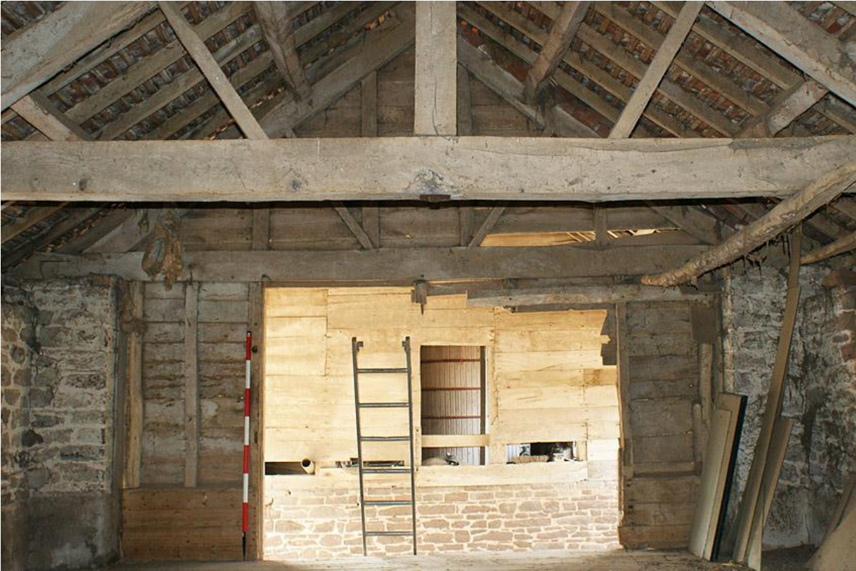
Plate 20 Interior of the south gable from the north
