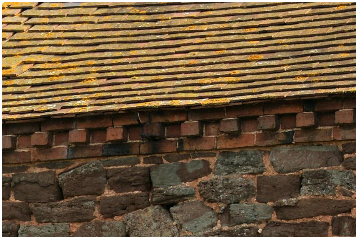
Plate 18 Dentilated cornice on west elevation
