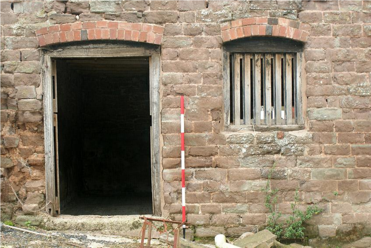
Plate 28 Southern stable door and window on east elevation
