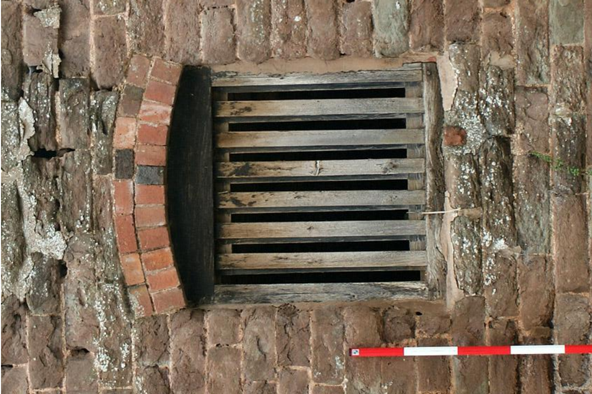
Plate 6 East elevation ground floor windows
