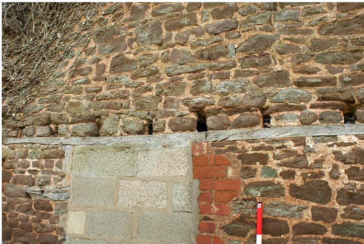
Plate 13 North elevation, holes from former floor joists
