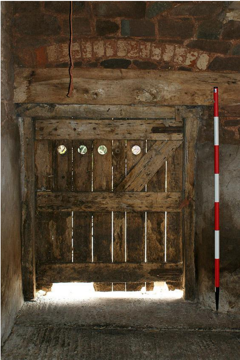
Plate 30 Blocked door interior
