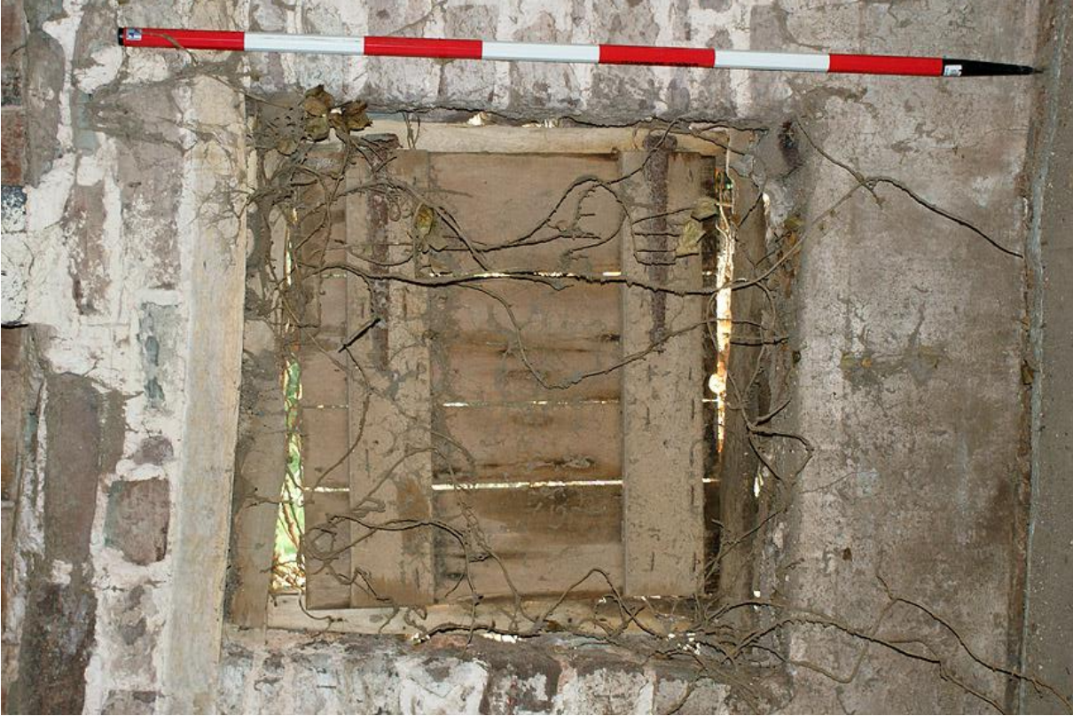
Plate 8 Upper floor window with shutter
