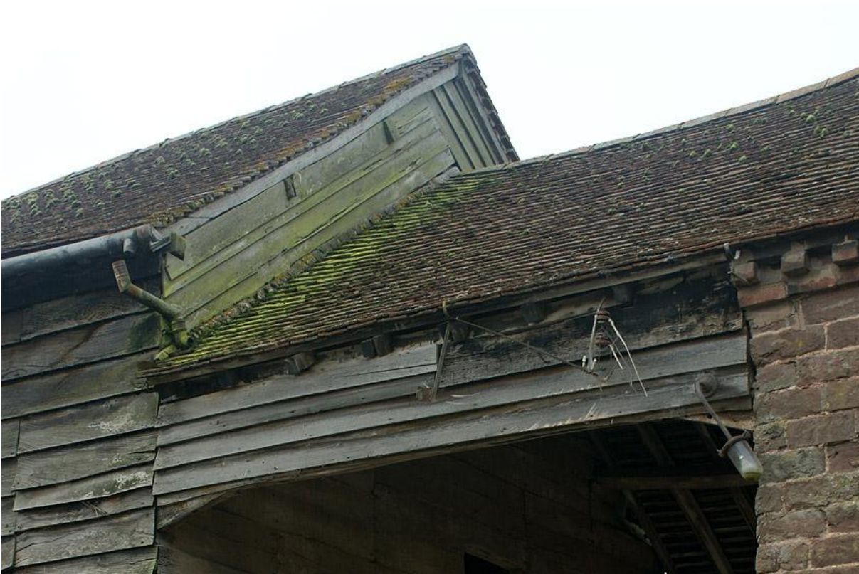
Plate 26 External weather-boarding of access way, east side
