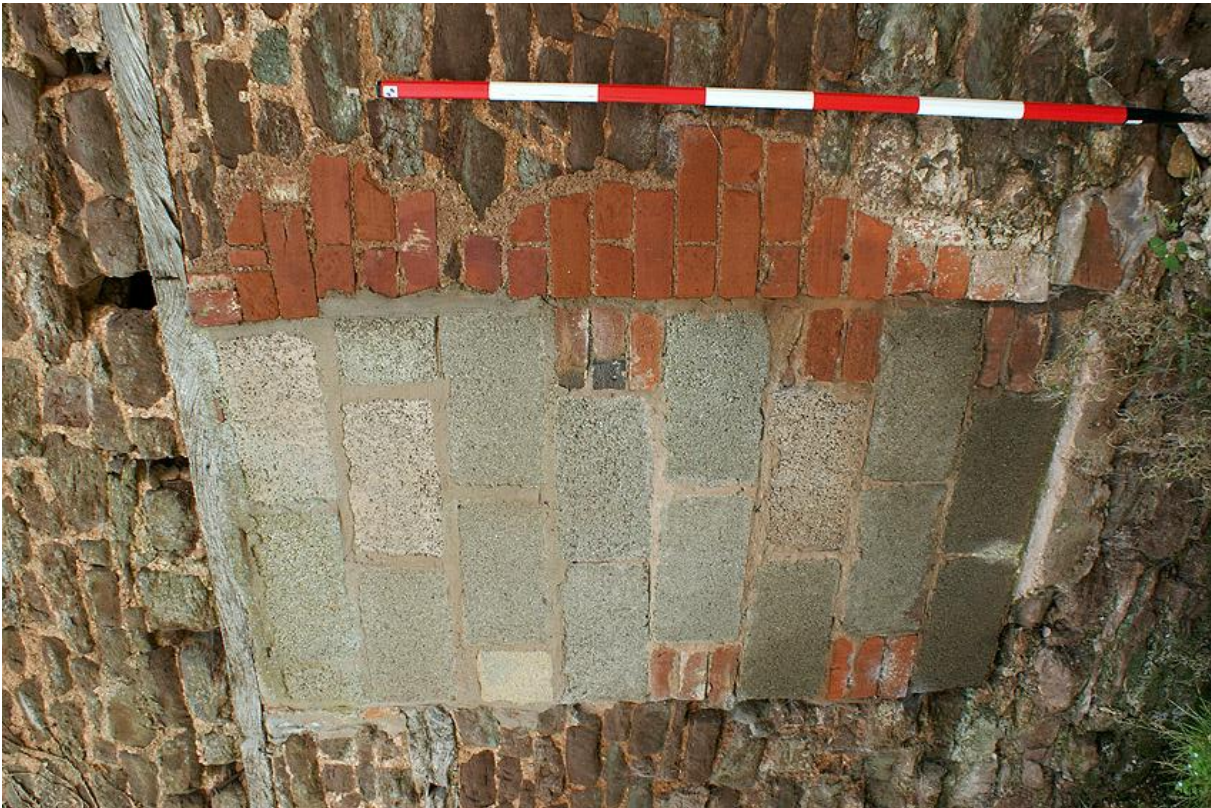
Plate 12 North elevation blocked door
