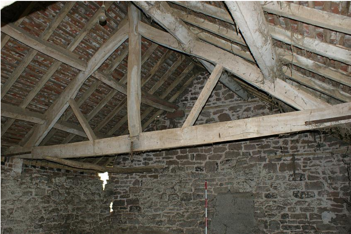
Plate 23 King-post roof truss
