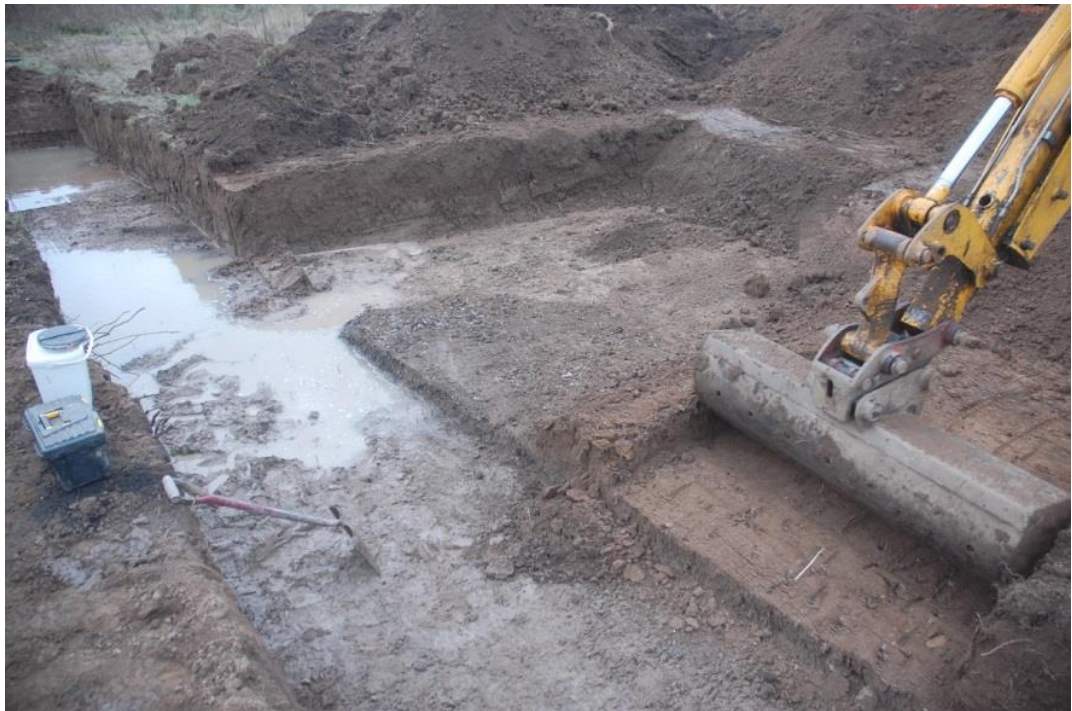
Plate 6: Burnt mound deposit 305 during machining in Trench 3 extension
