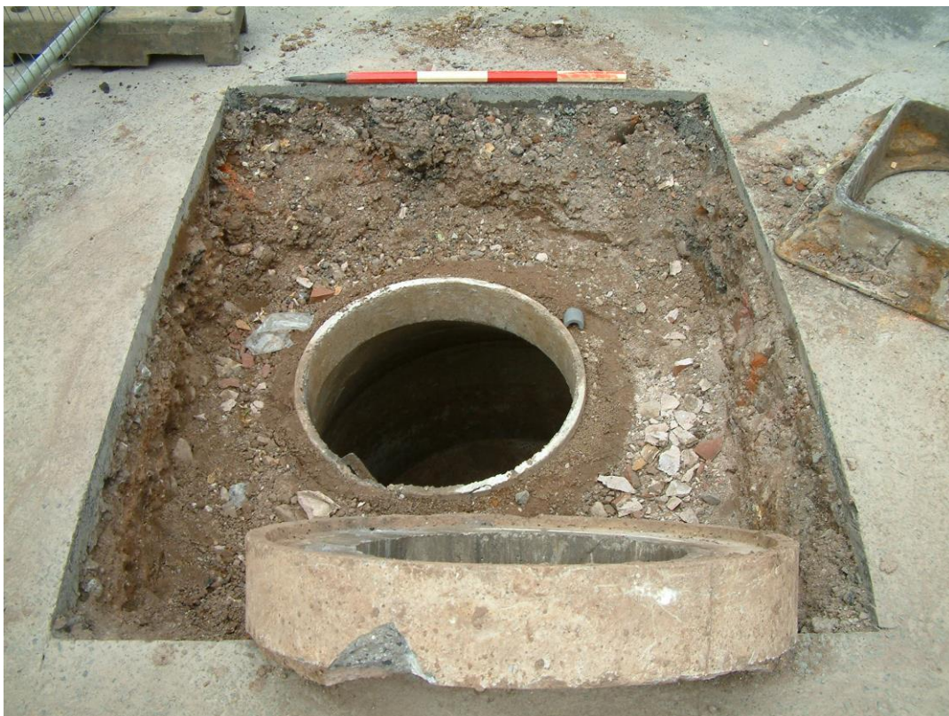
Plate 2: Trench 2, Edgar Street
