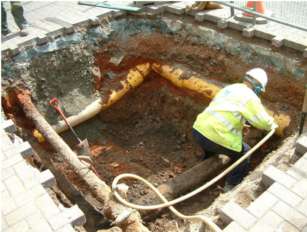
Plate 1: Trench 1, Park Street/Wyld's Lane
