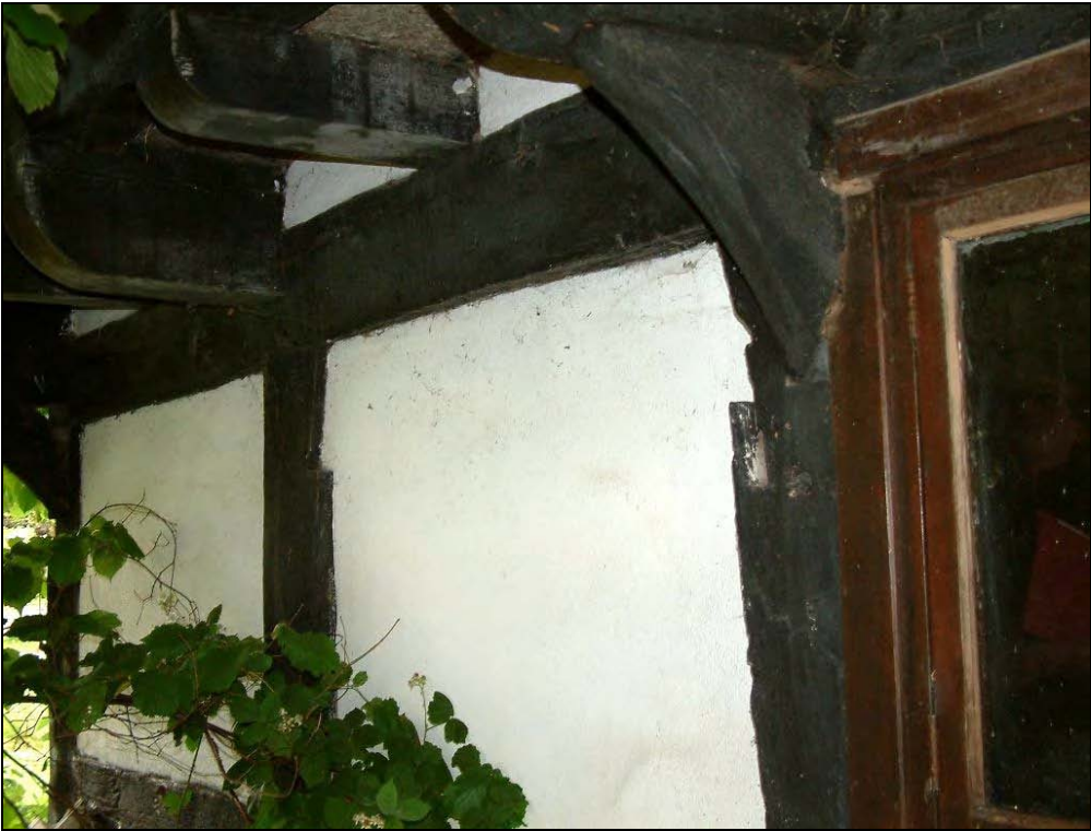
Plate 6: Position of former doorway on north-west elevation of the building
