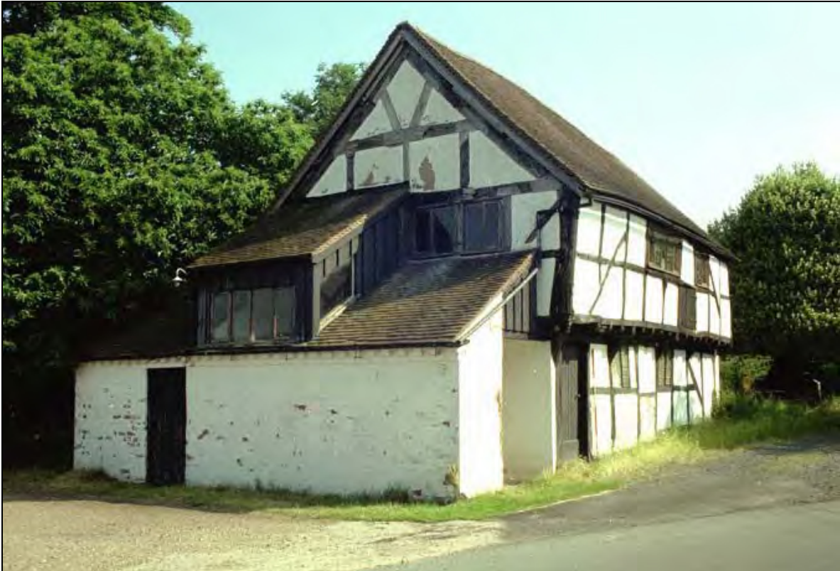
Plate 1: Church House from the south
