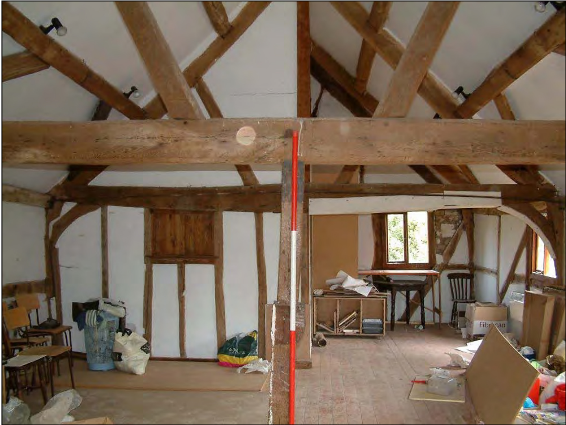
Plate 19: First floor partition
