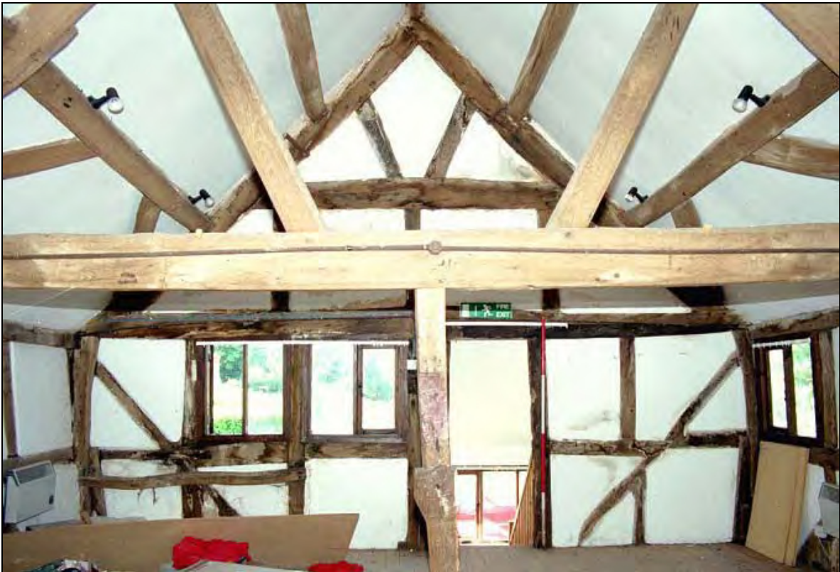
Plate 2: First floor, interior facing south-west
