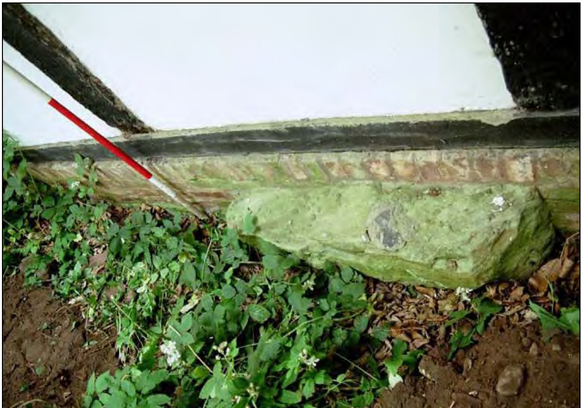
Plate 4: Stone foundation on north-west elevation of building
