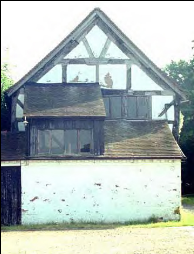
Plate 14: South-west gable of the building with added 1820s extension
