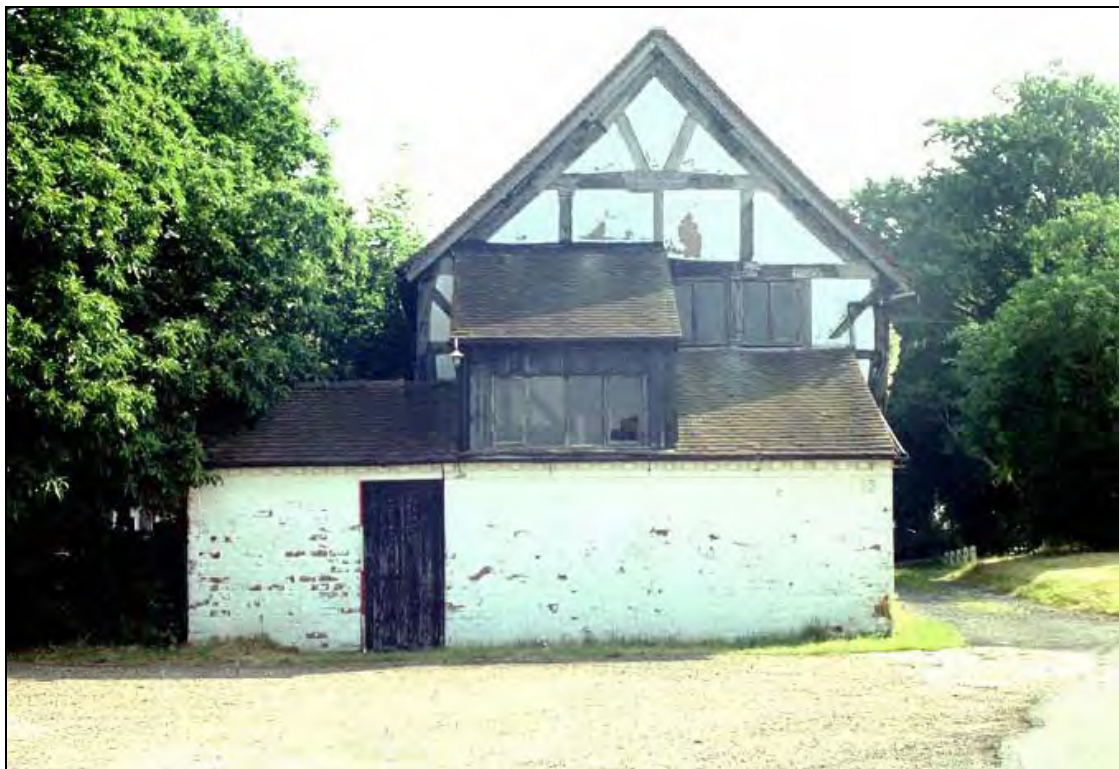
Plate 16: South-west gable with 1890s added extension
