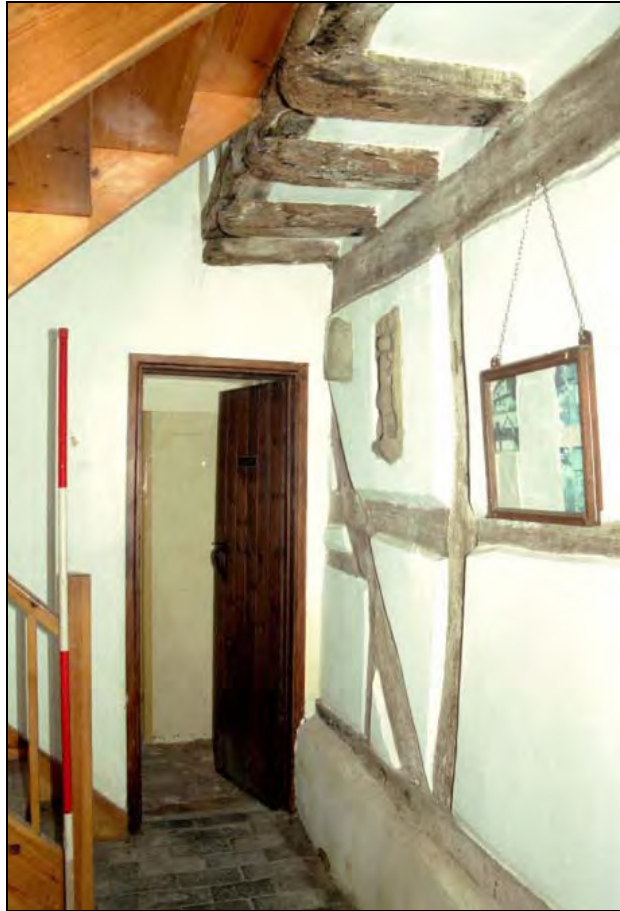
Plate 15: Groom's room (entrance hall) facing north-west
