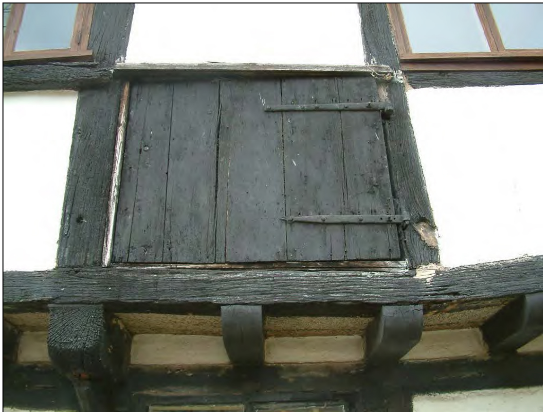
Plate 12: Hayloft door on south-east elevation
