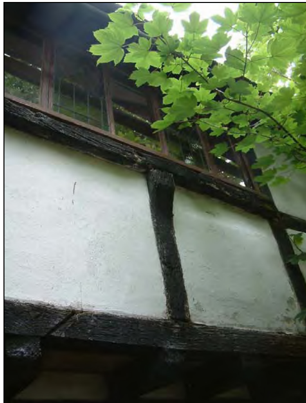
Plate 8: First floor oriel window with cove strut.
