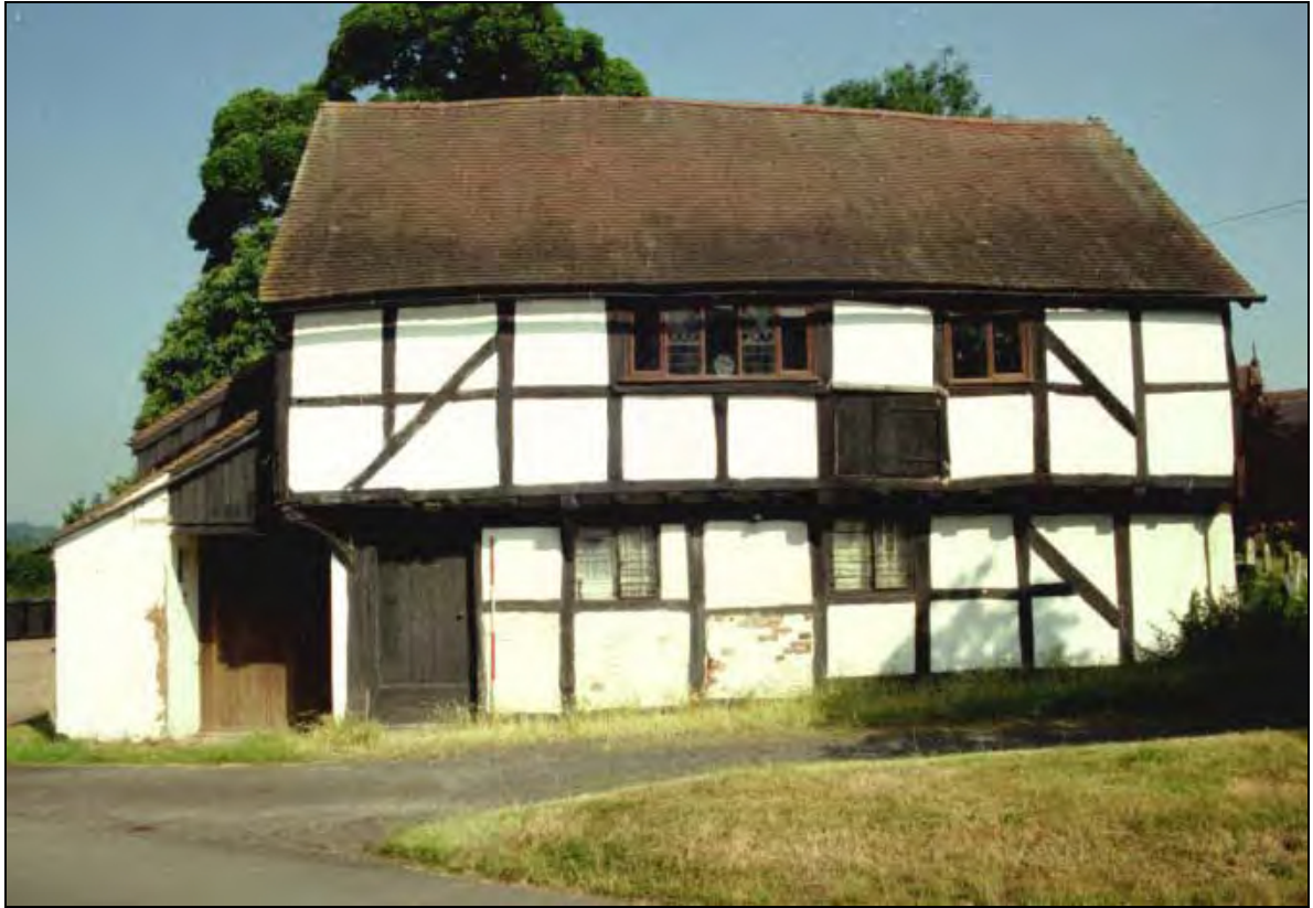
Plate 3: Church House from the south-east
