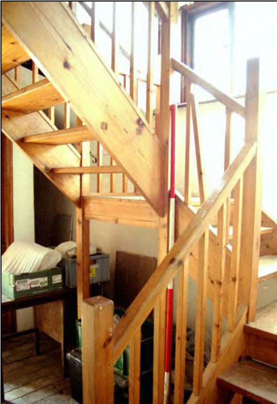
Plate 17: Staircase added to groom's room
