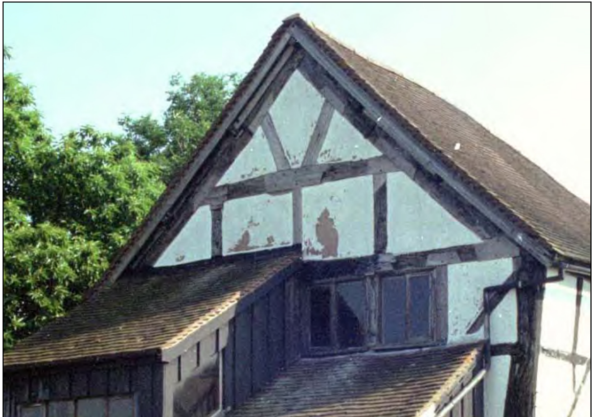
Plate 20: Replaced exterior joints on south-west gable
