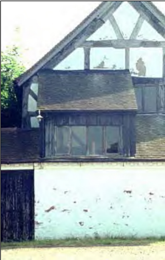
Plate 18: Staircase rising through groom's room roof
