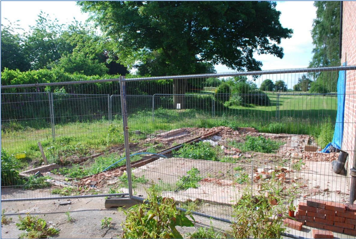
Plate 1 The footings of the previous building looking southeast
