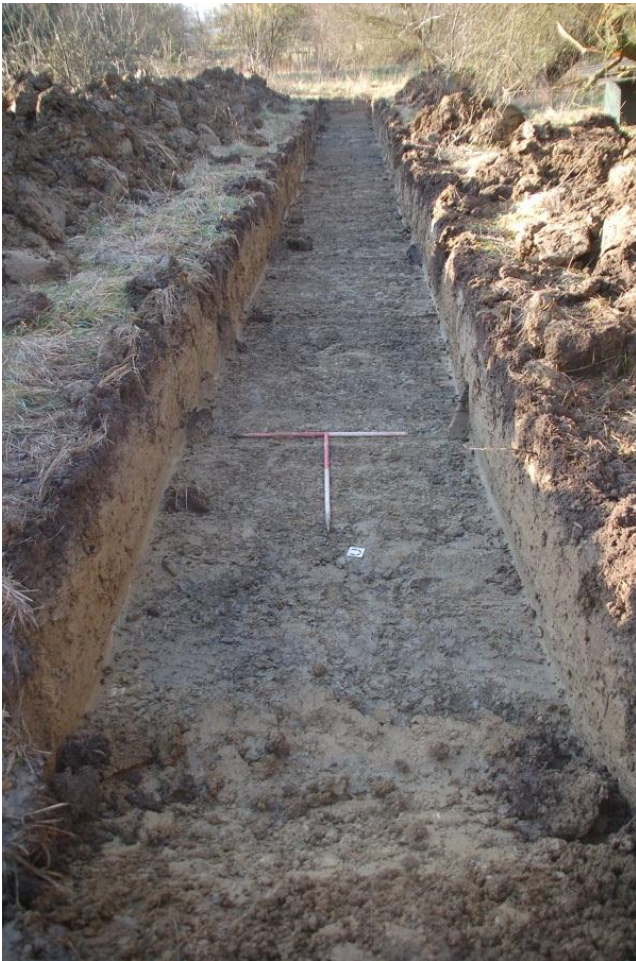
Plate 5: General view of Trench 2, facing east
