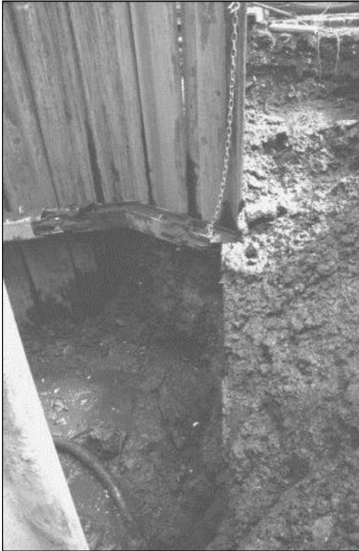
Plate 7: Location of stone wall beneath open south side of shuttering
