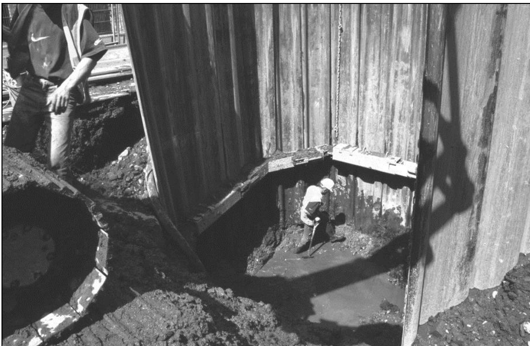
Plate 6: Deep excavations at foot of Dog Lane
