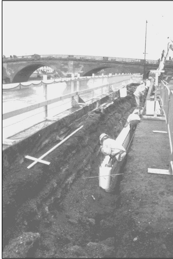
Plate 3: General view of guide trench showing dumped gravels in west-facing section
