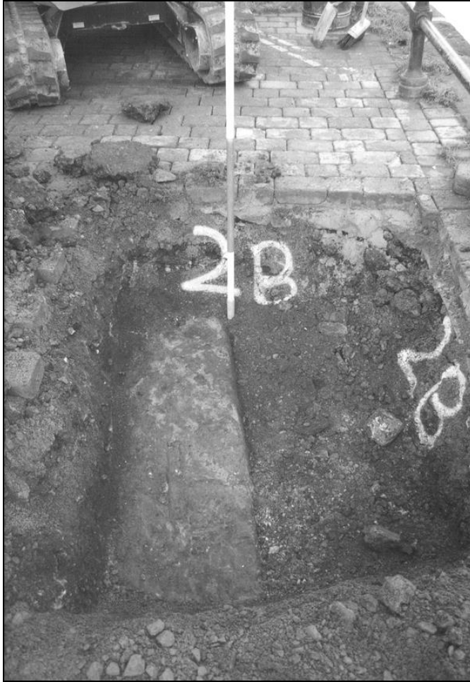
Plate 1: Top of former quayside wall exposed in test-pit 10
