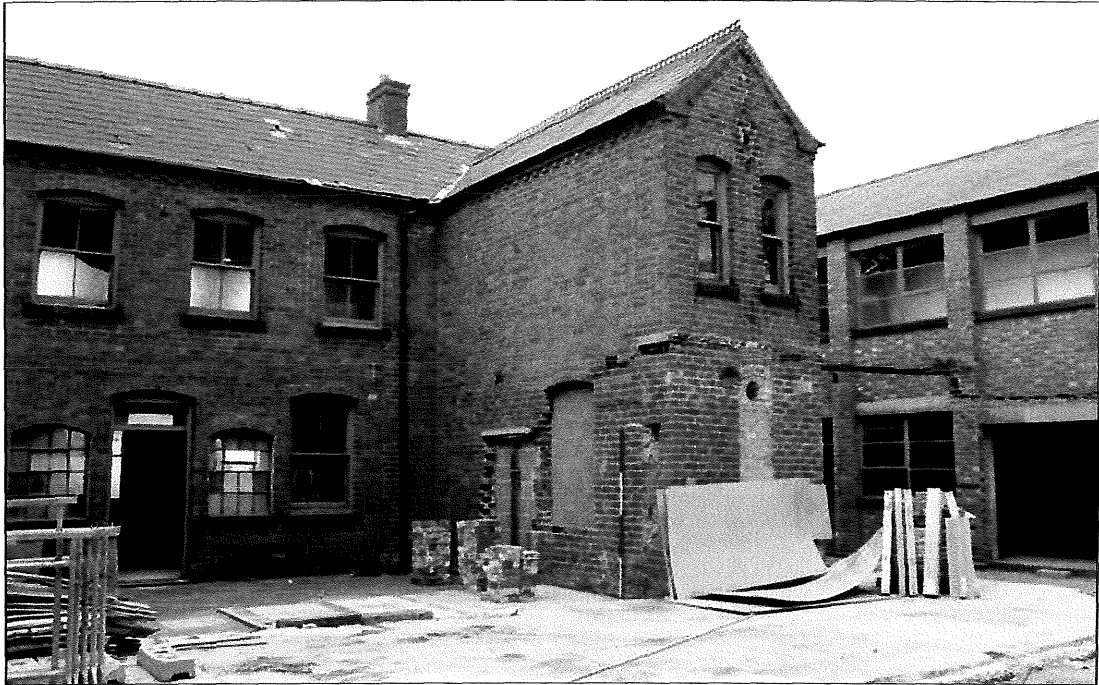
Plate 7: Northern range courtyard facing elevation
