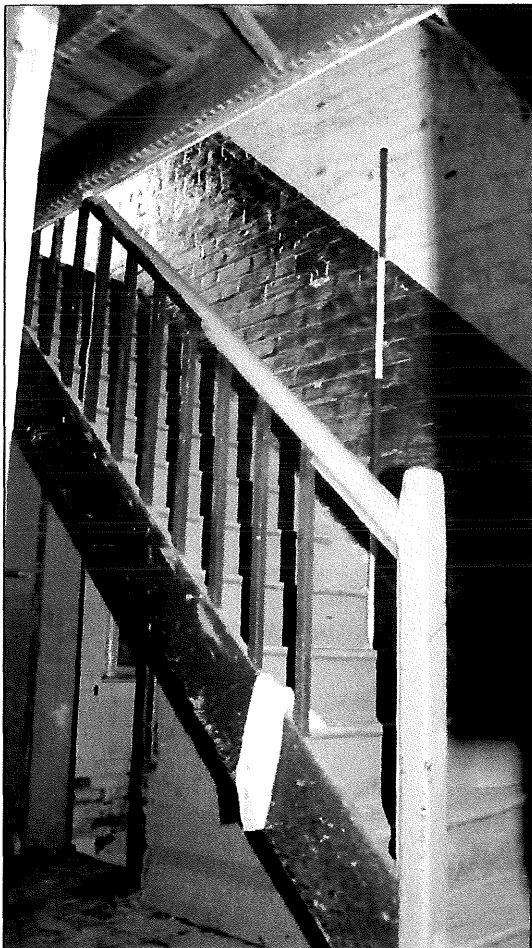
Plate 12: Main staircase from the Crescent Works inserted against the original external wall of the Walton Works. The plinth below the stairs is an indicator that this wall was external when built
