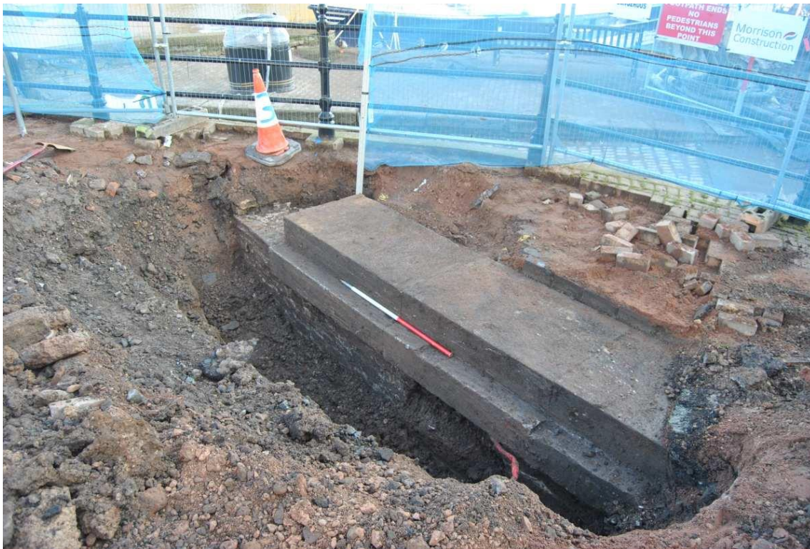
Plate 6: Granite running block (8171) capping the eastern, downstream drawbridge wall; 1m scale; view north-east
