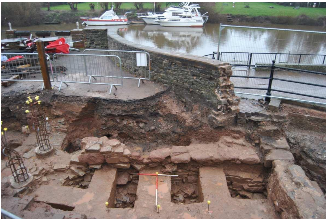
Plate 4: The post-medieval bridge; wall 8106 to the left, wall footing 8157 to the centre; later wall 8146 above; drawbridge wall 8158 to the right; the curved wall for the swing bridge still upstanding above; 1m scales; view north (Figs 10 and 11)
