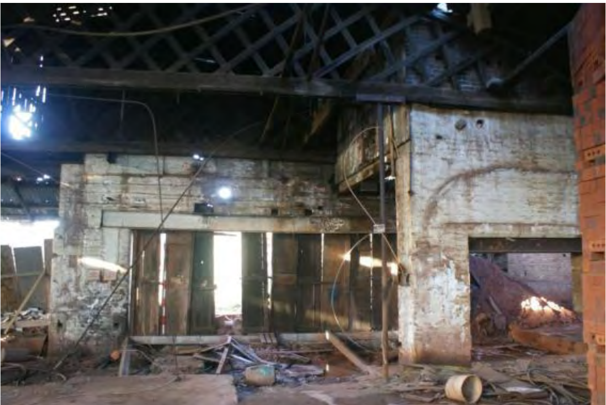
Plate 56 Structure 8, looking west
