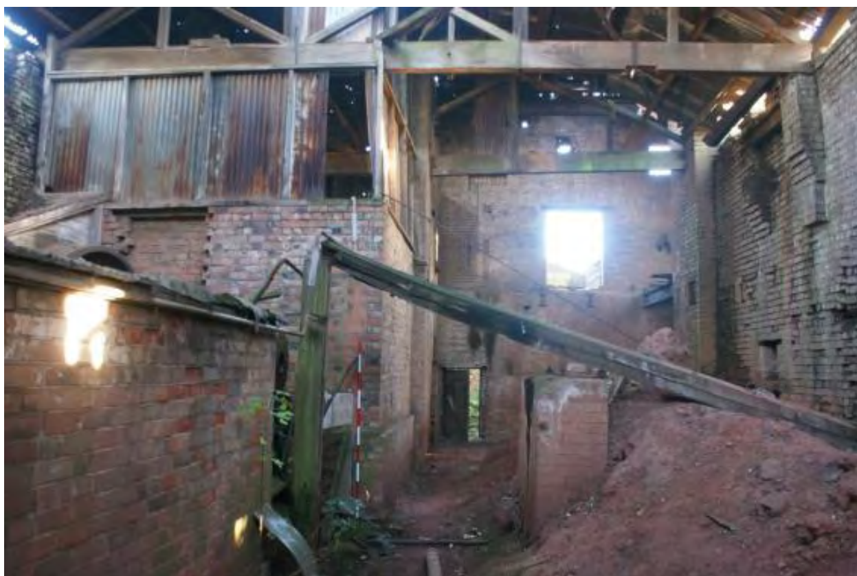
Plate 40 Structure 10, looking east
