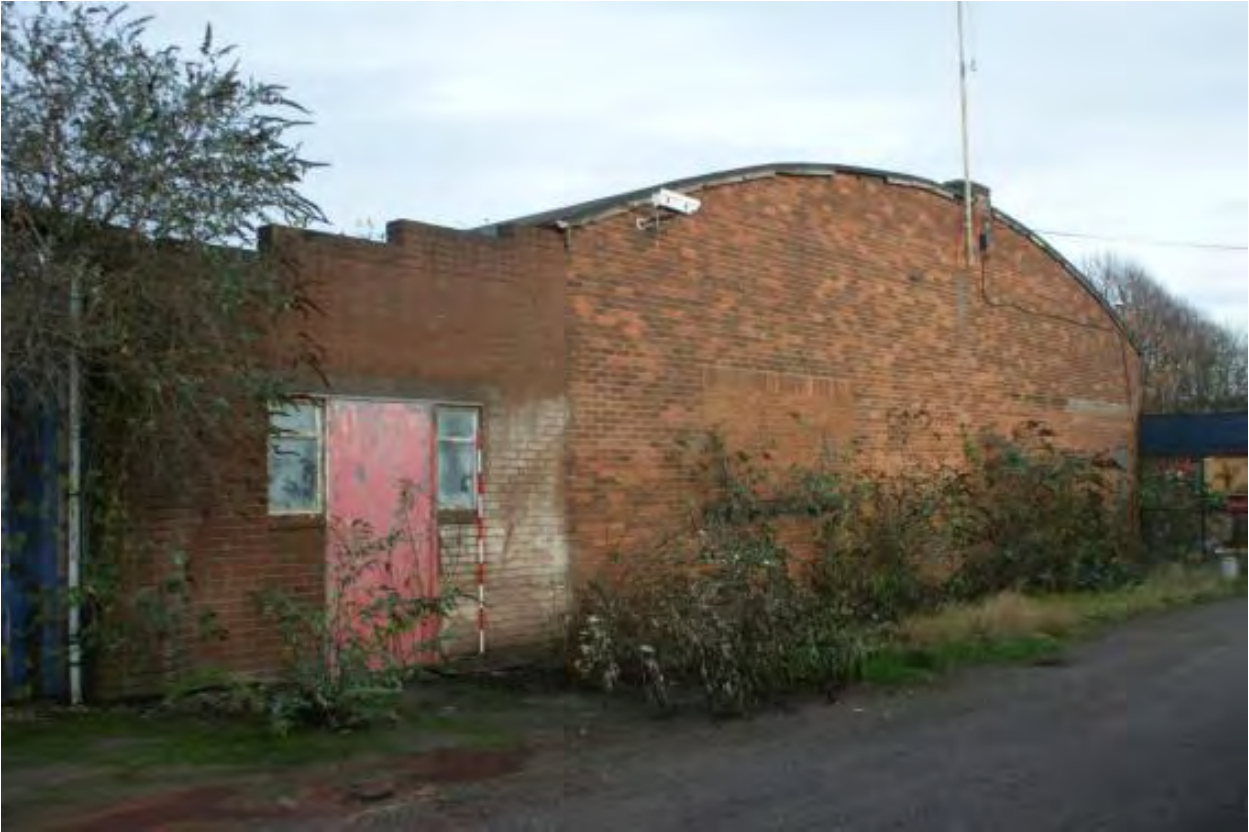
Plate 68 Structure 22, looking north-east
