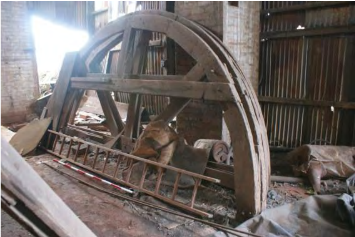
Plate 14 Structure 1 arch former, looking north-west
