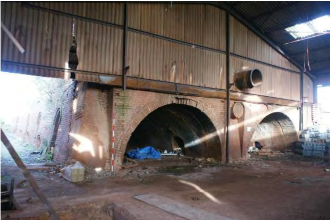
Plate 9 Structure 1, looking north-east
