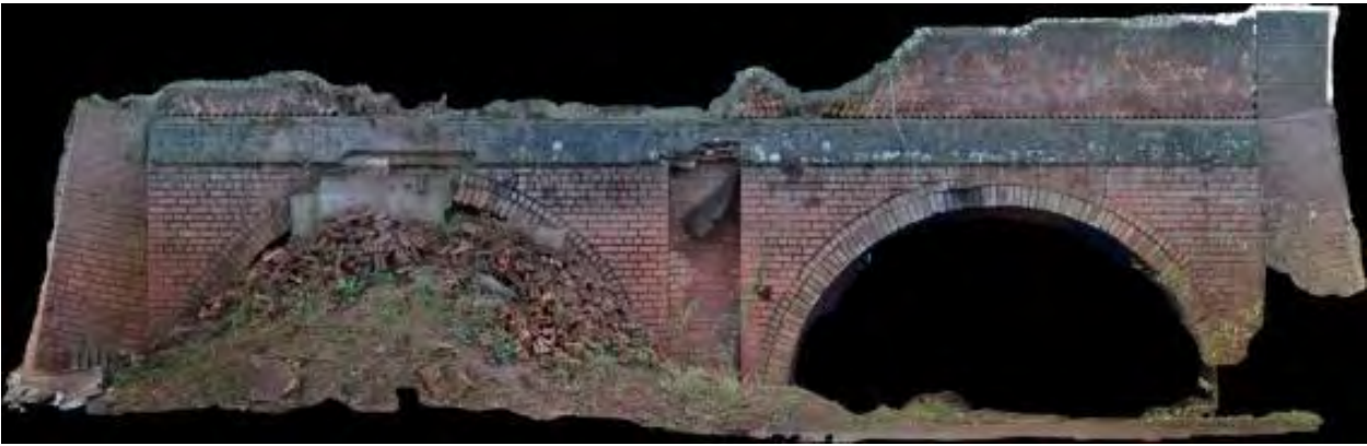
Plate 11 Structure 1, looking south
