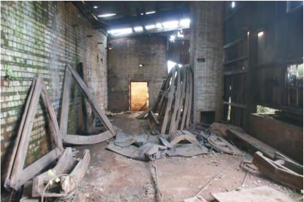
Plate 77 Structure 21, looking west
