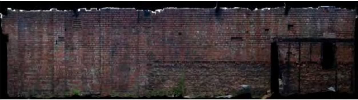
Plate 23 Structure 9, looking west
