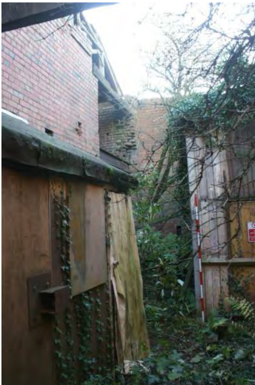
Plate 63 Structure 17, looking south-east
