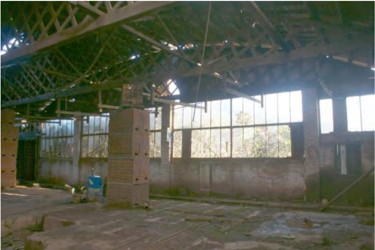
Plate 57 Structure 8, looking north-east
