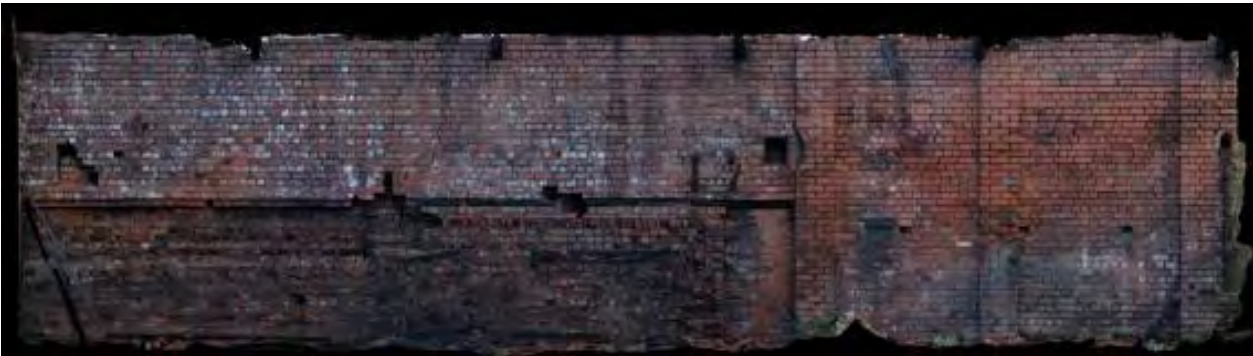
Plate 22 Structure 9, looking east
