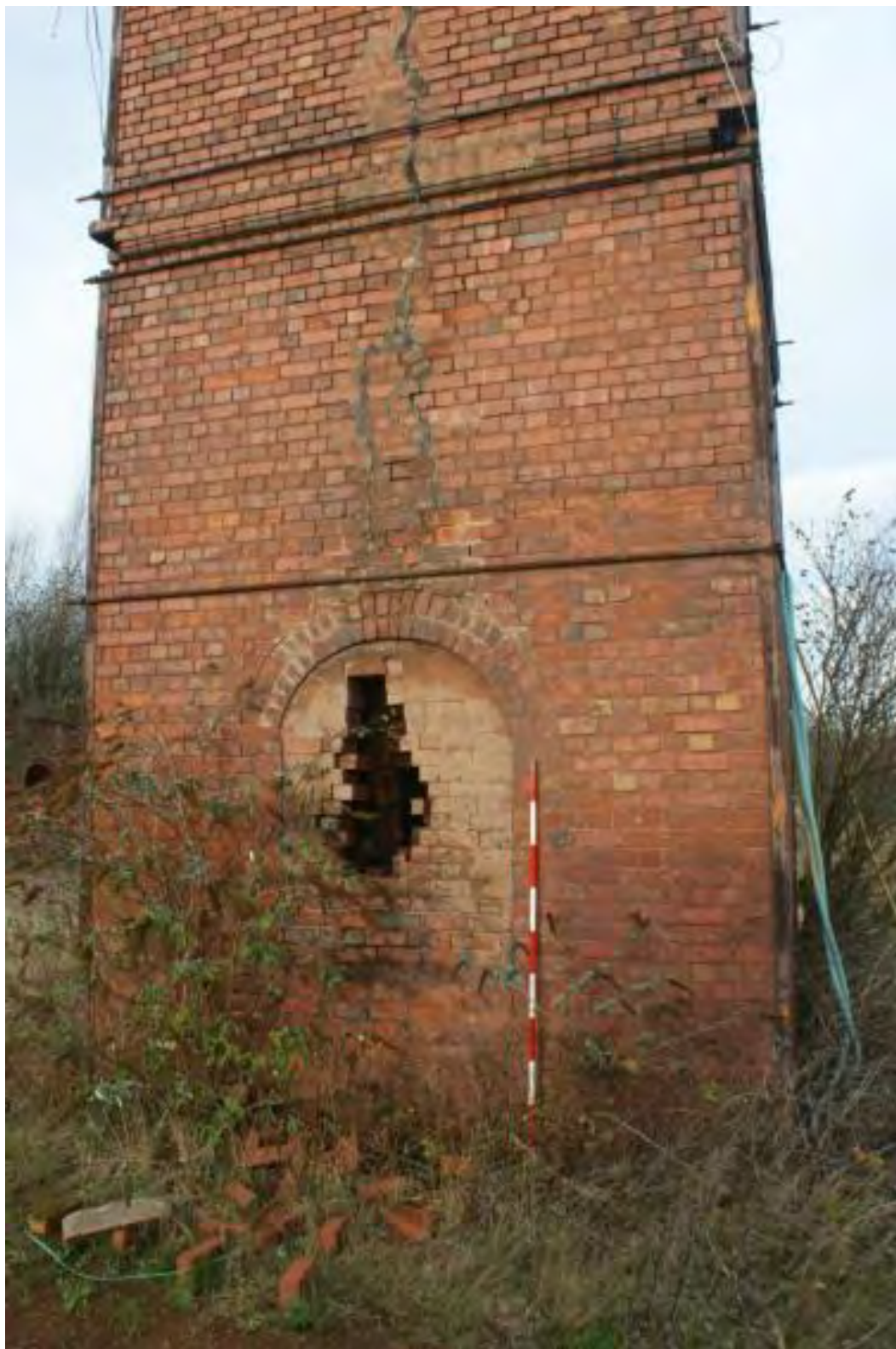
Plate 19 Structure 2, looking north
