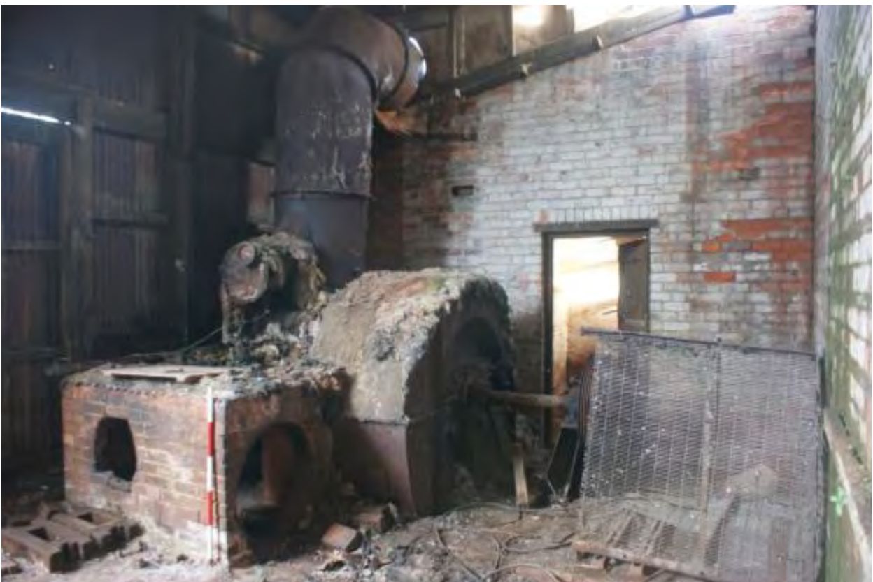
Plate 78 Structure 21, looking north-east
