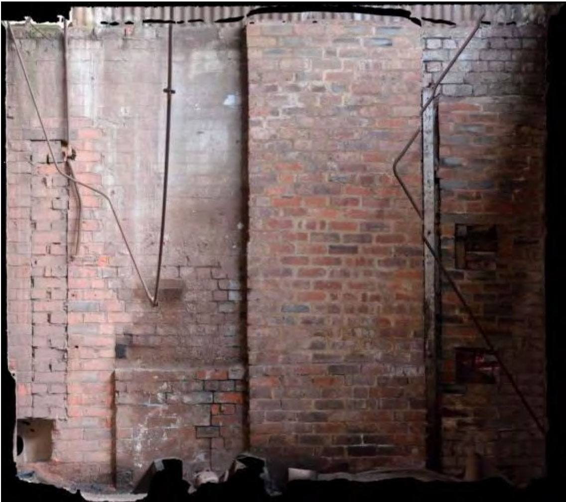
Plate 47 Structure 10, looking west
