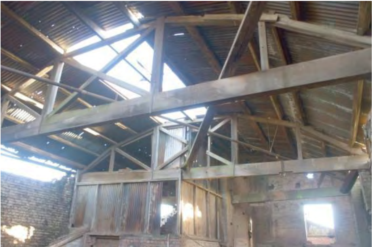
Plate 29 Structure 13, looking north-east
