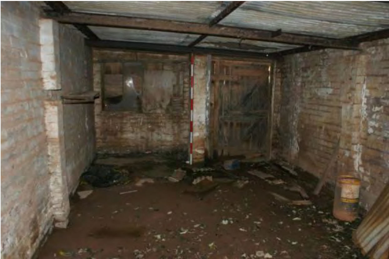
Plate 65 Structure 6, looking south
