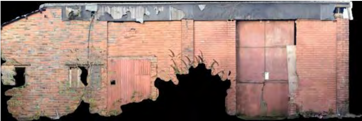
Plate 52 Structure 8, looking north
