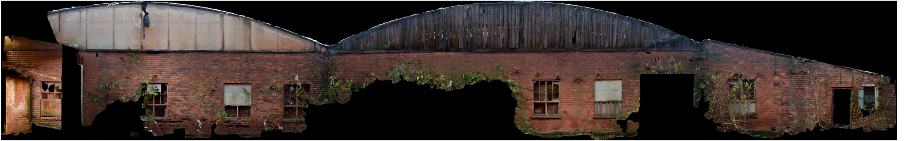
Rectified photograph of Structure 4 exterior elevation
