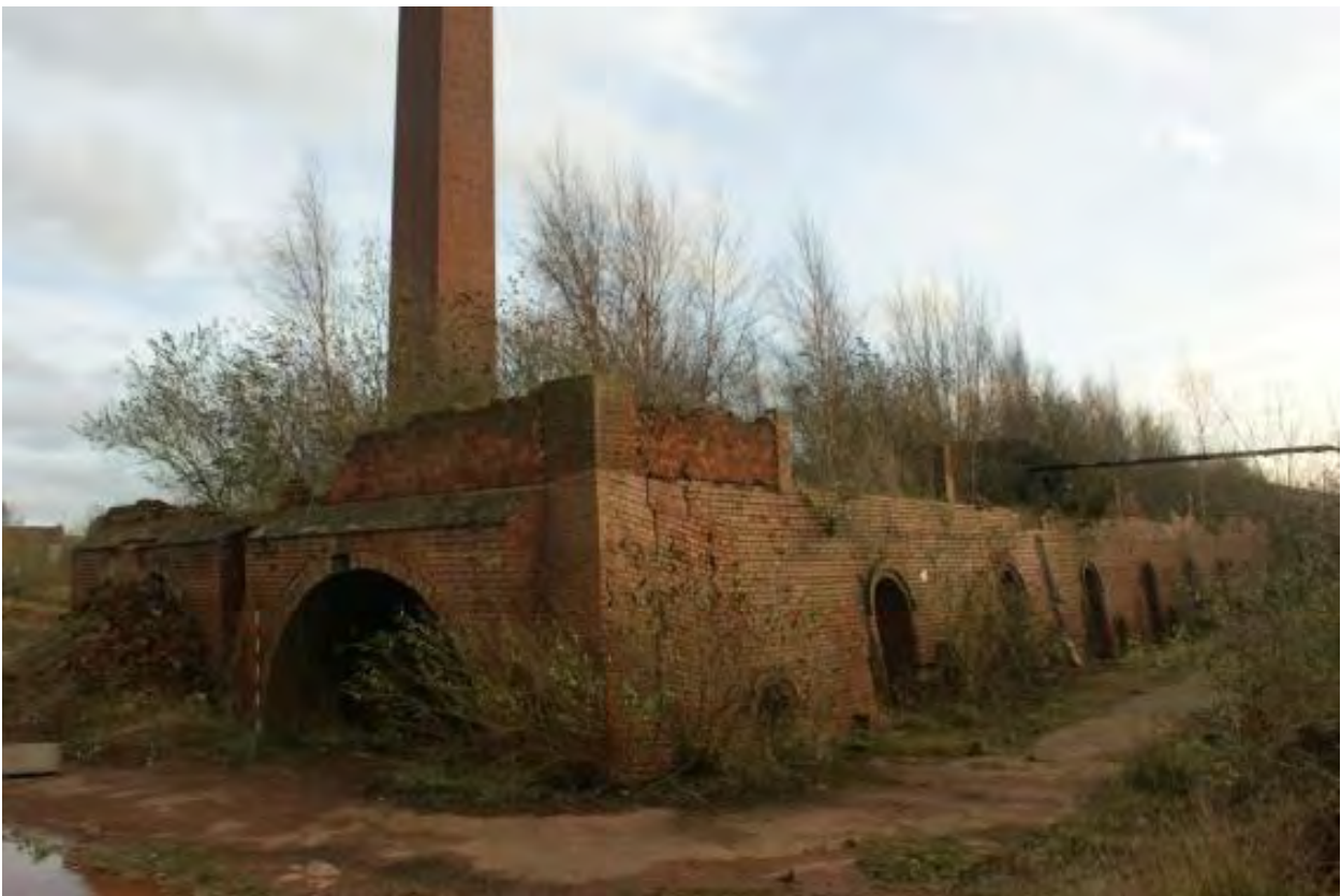
Plate 8 Structure 1, looking south-east
