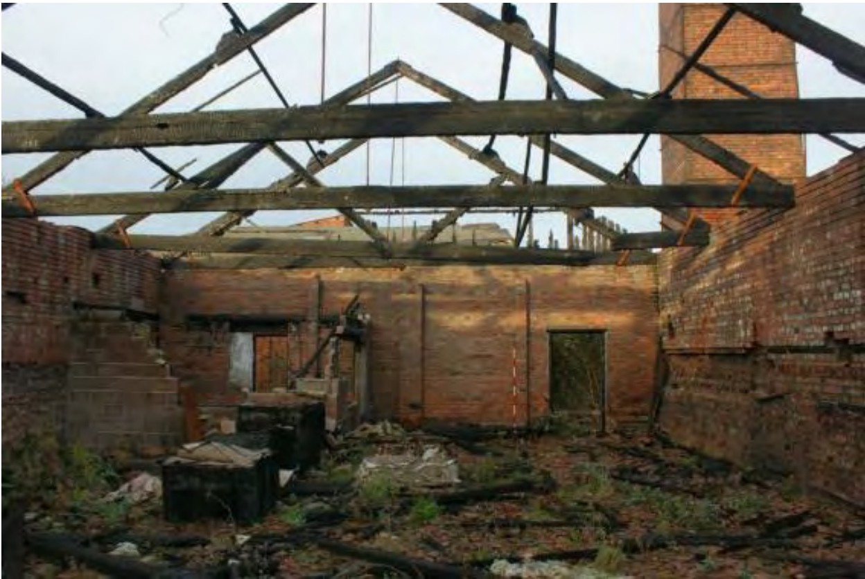
Plate 21 Structure 9, looking north
