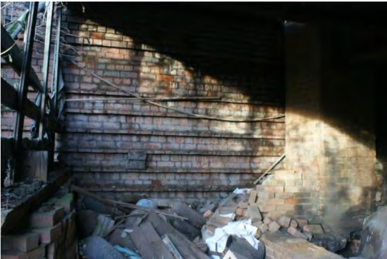
Plate 37 Structure 3, looking north
