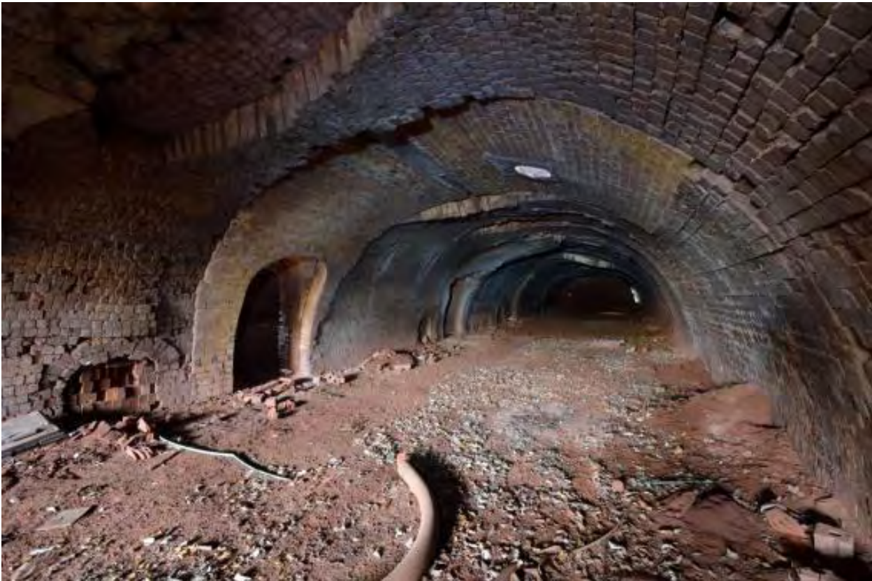
Plate 13 Structure 1, looking north
