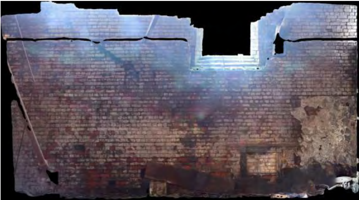
Plate 27 Structure 13, looking north
