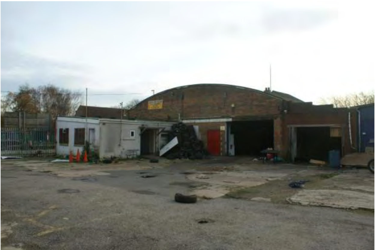
Plate 67 Structure 22, looking south
