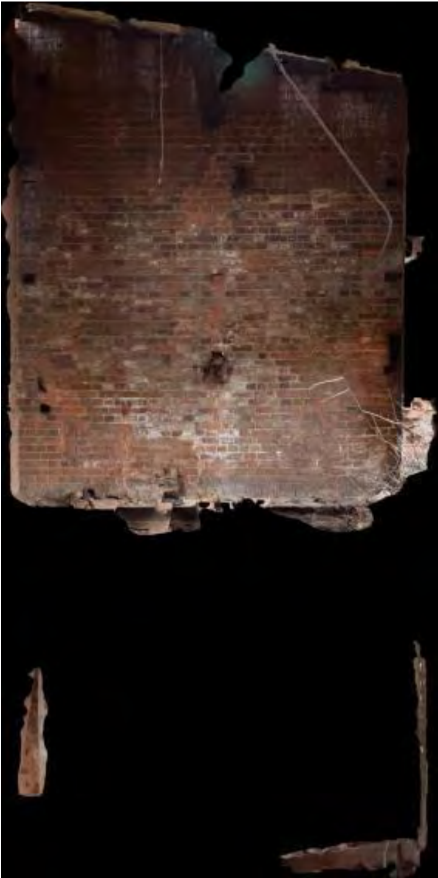
Plate 42 Structure 10, looking south
