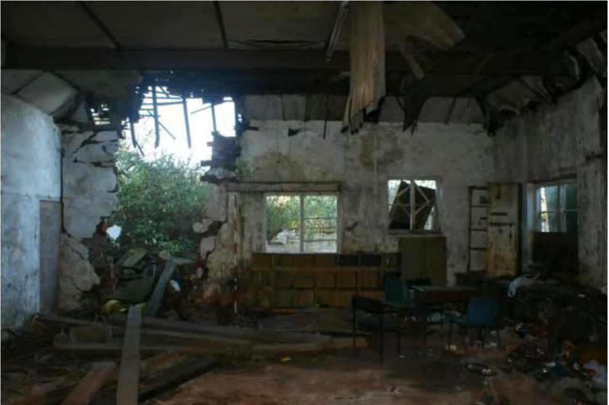
Plate 75 Structure 5, looking west
