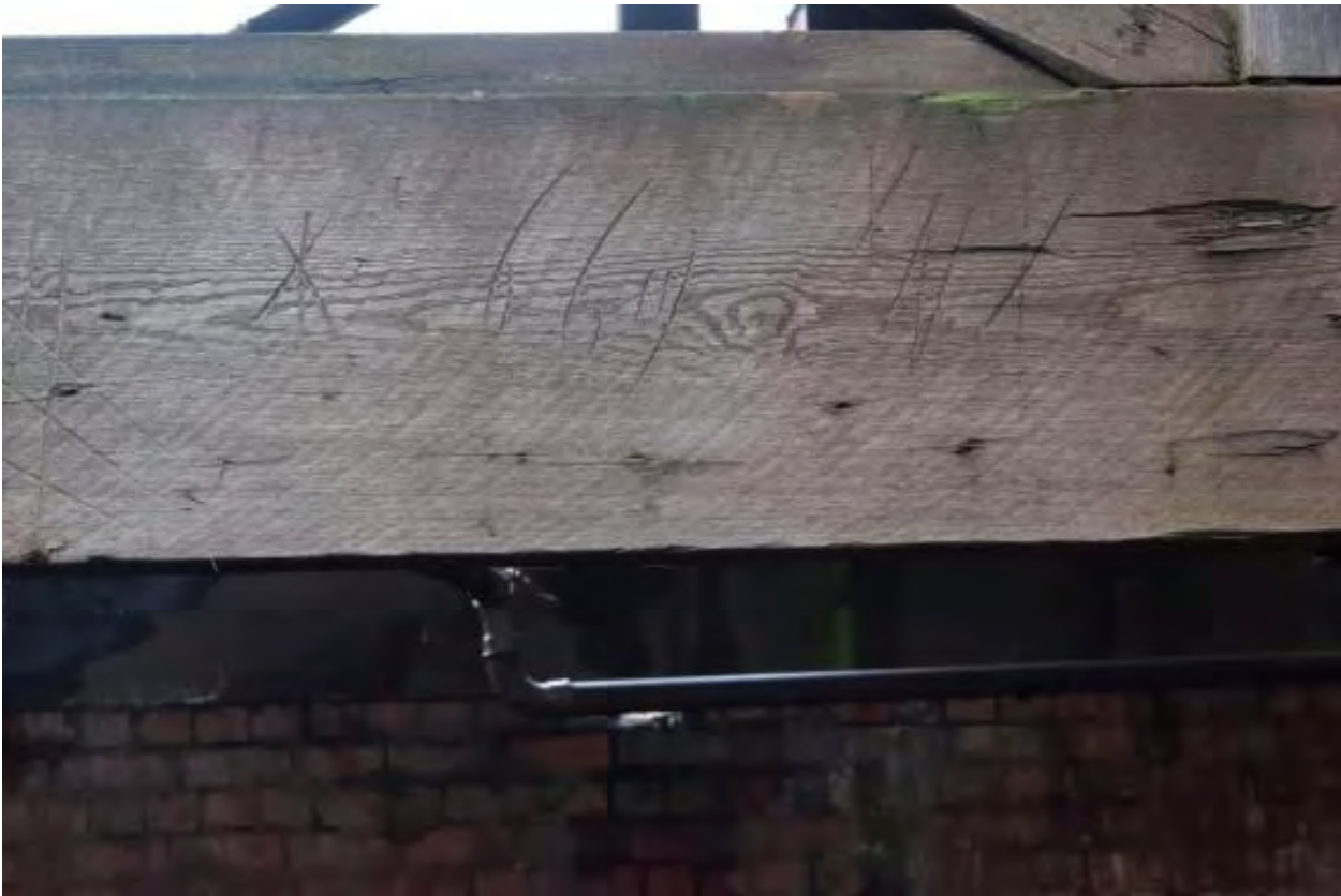
Plate 30 Structure 13, looking west
