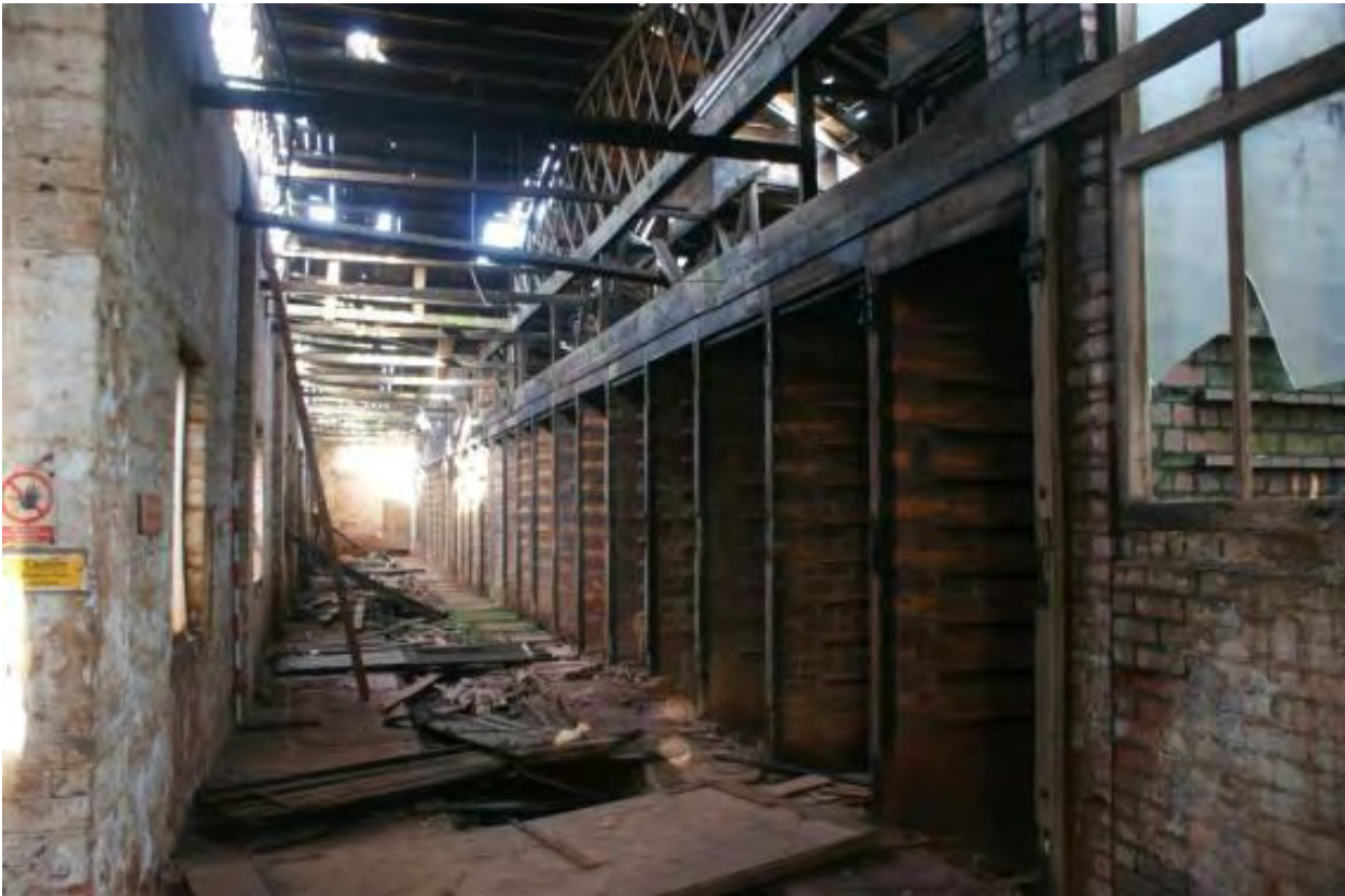
Plate 34 Structure 3, looking north
