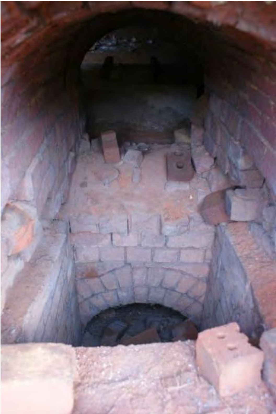
Plate 18 Structure 1, looking east
