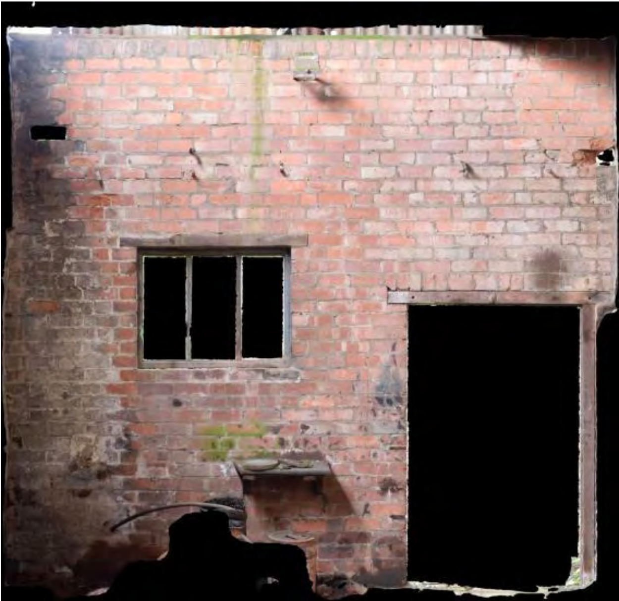
Plate 45 Structure 14, looking east
