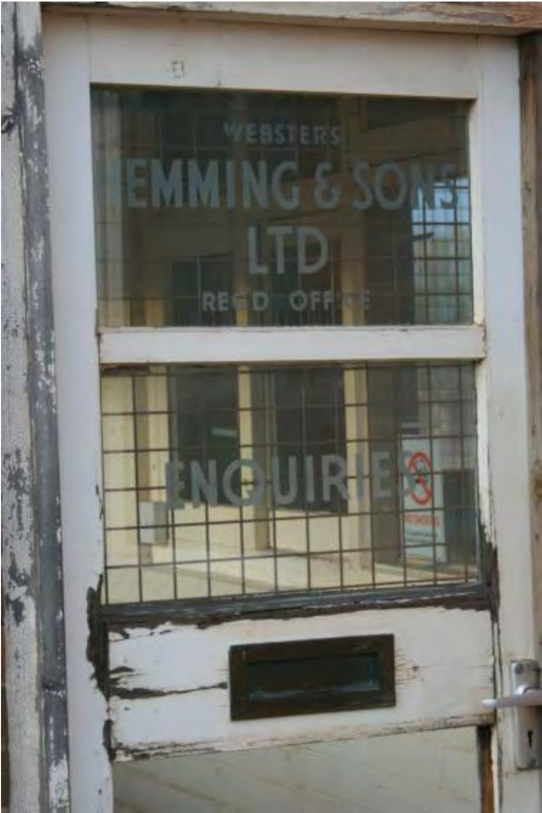
Plate 72 Structure 23, looking west
