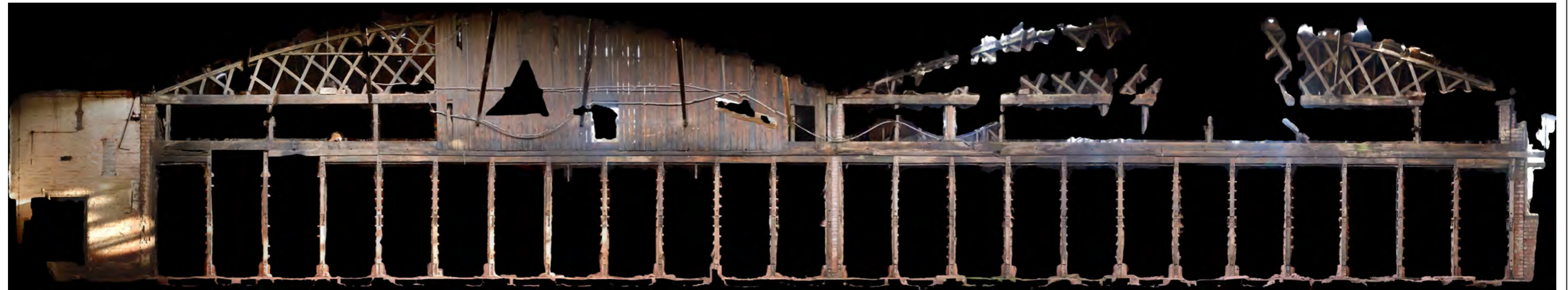
Rectified photograph of Structure 3 western elevation with later Belfast trusses above
