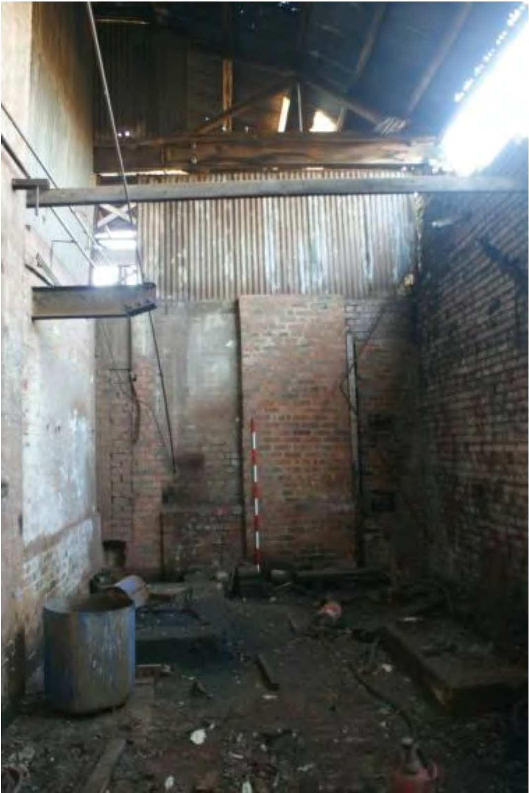
Plate 43 Structure 10, looking west
