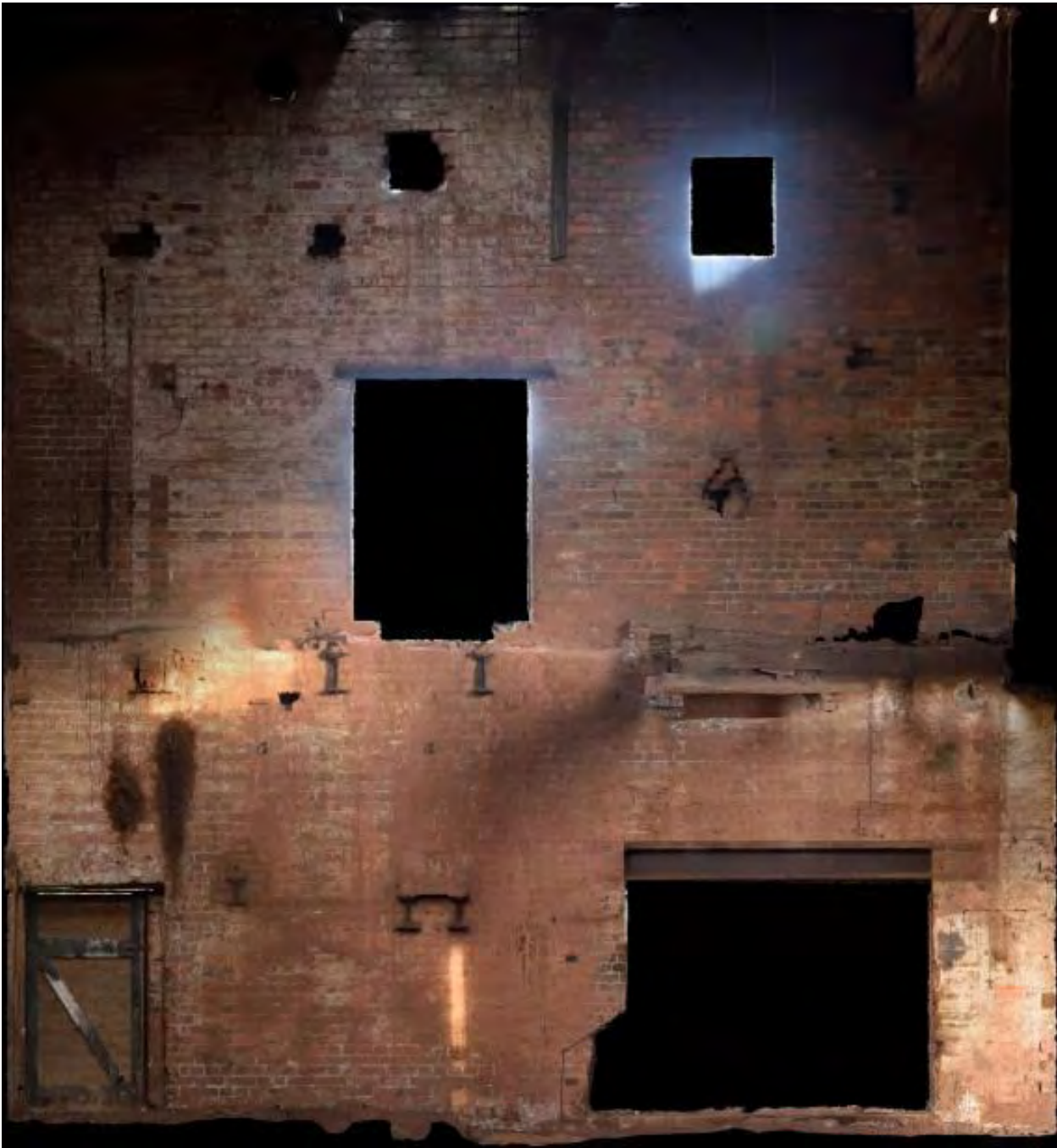
Plate 41 Structure 10, looking east
