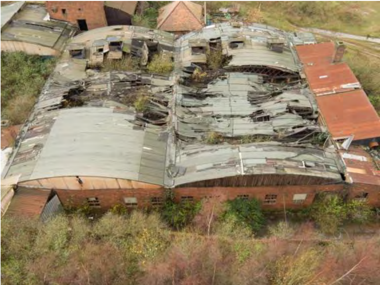
Plate 39 Structure 3 chimneys, looking west
