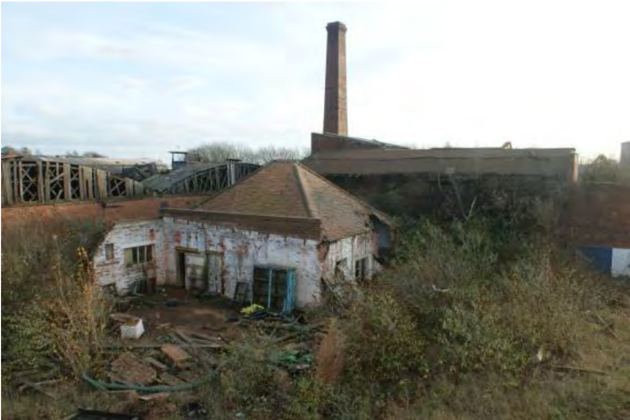
Plate 73 Structure 5, looking south-east
