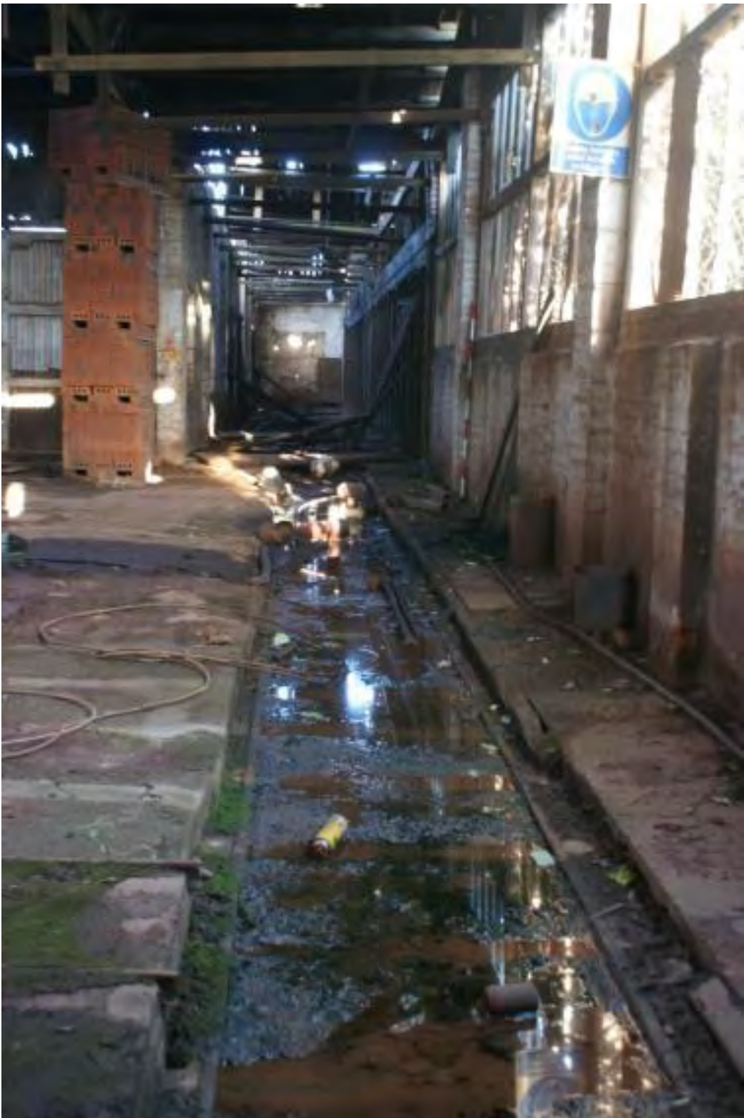
Plate 54 Structure 8, looking north
