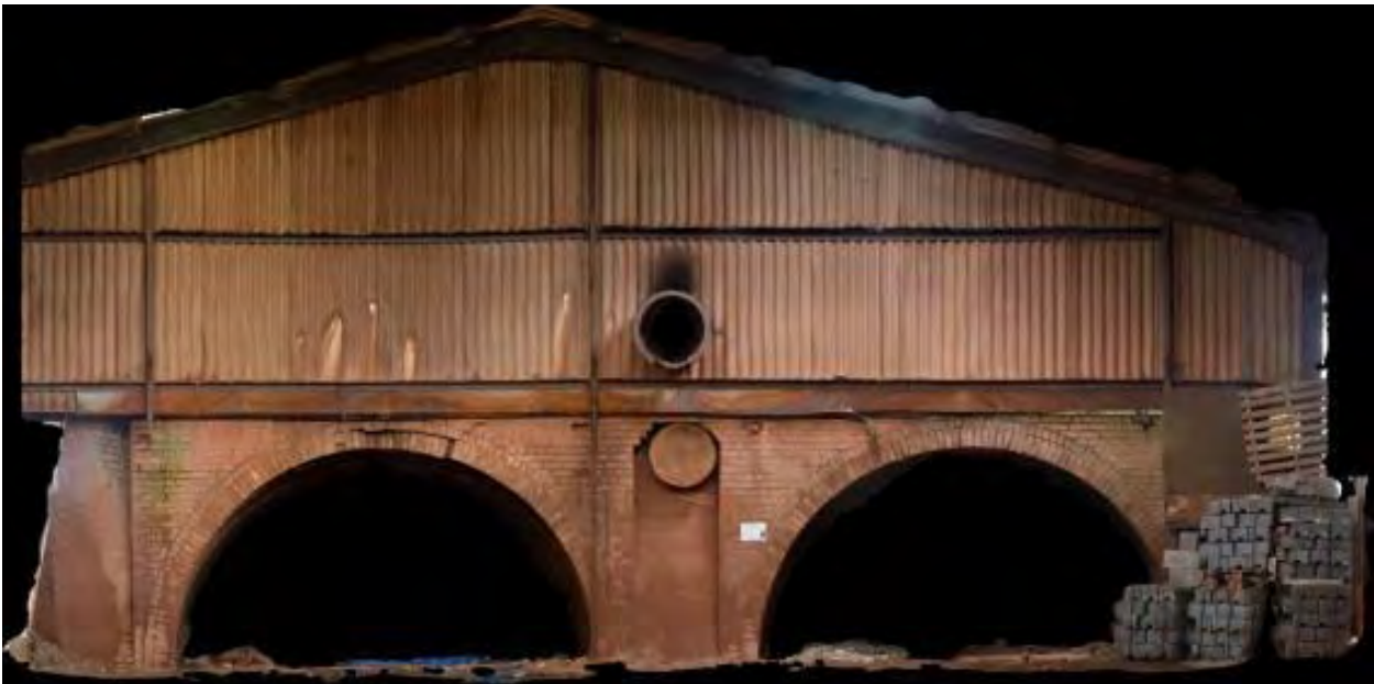
Plate 10 Structure 1, looking north
