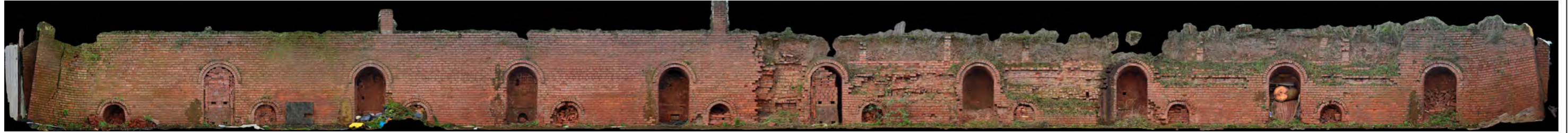
Structure 1 eastern elevation
