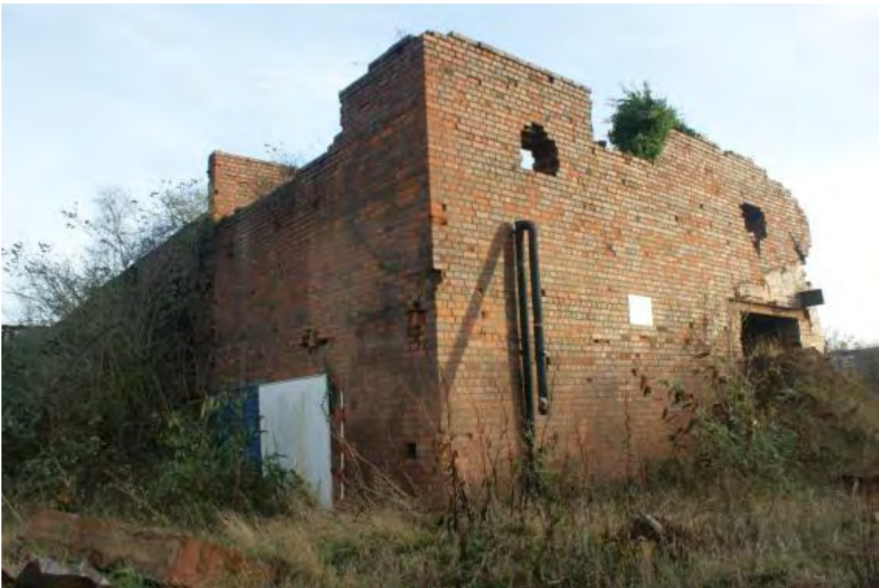
Plate 62 Structure 17, looking south-east
