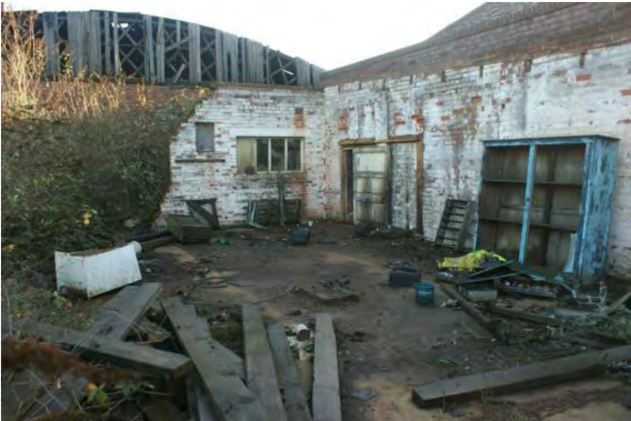
Plate 74 Structure 5, looking south-east
