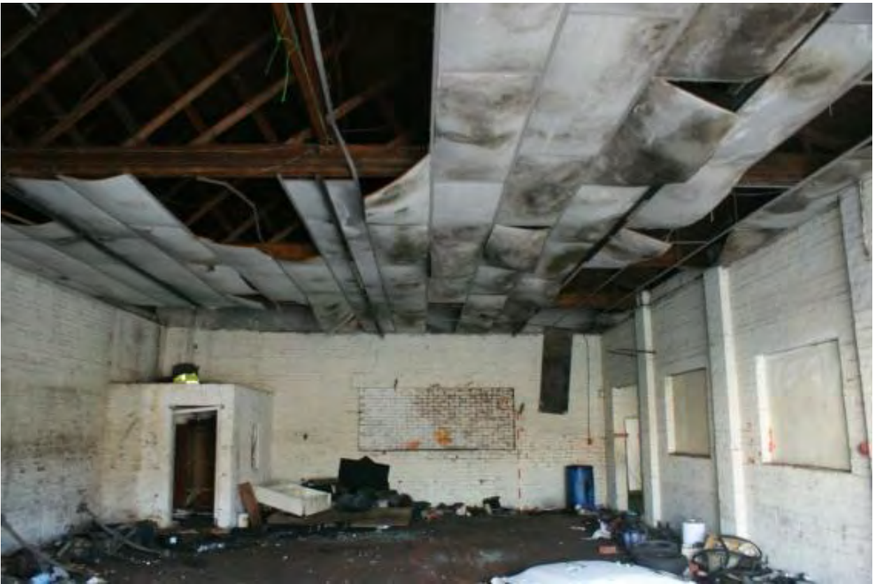
Plate 69 Structure 22, looking south
