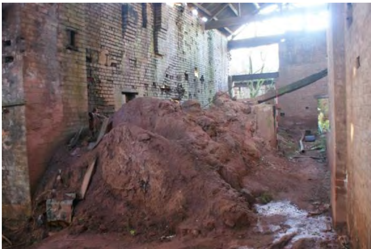
Plate 32 Structure 13, looking west
