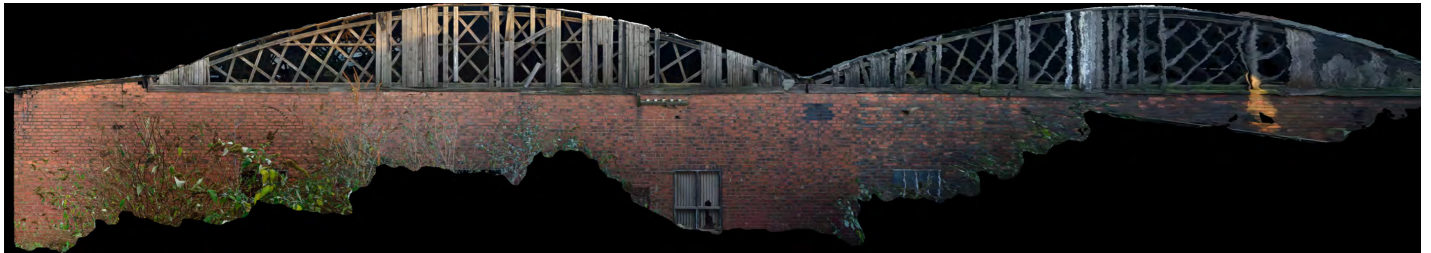
Rectified photograph of Structure 5 exterior elevation
