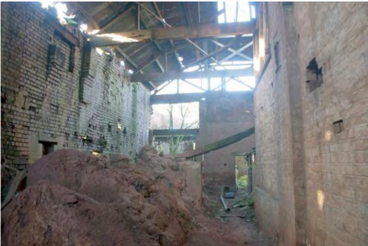
Plate 59 Structure 15, looking west
