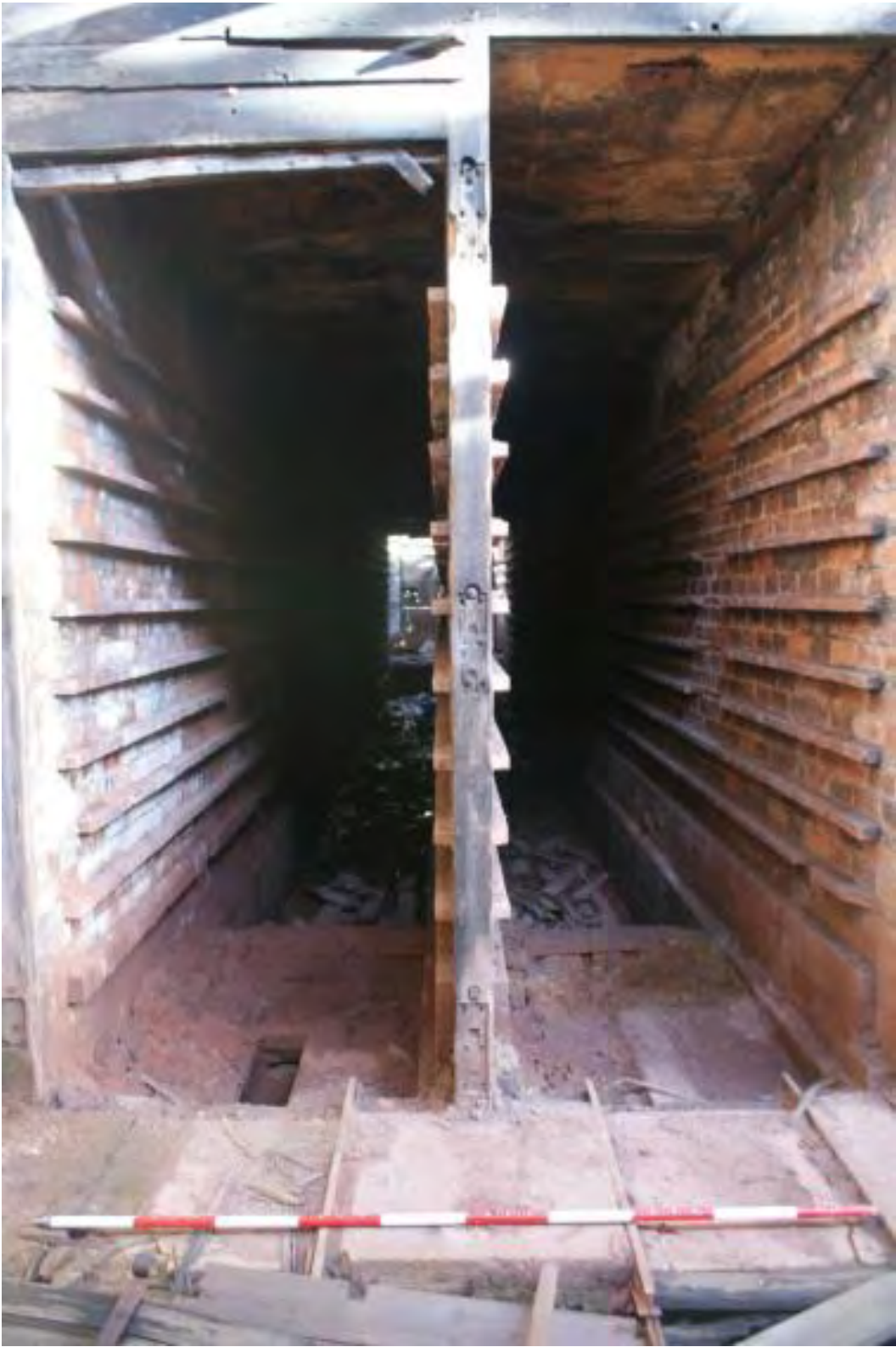
Plate 35 Structure 3, looking west
