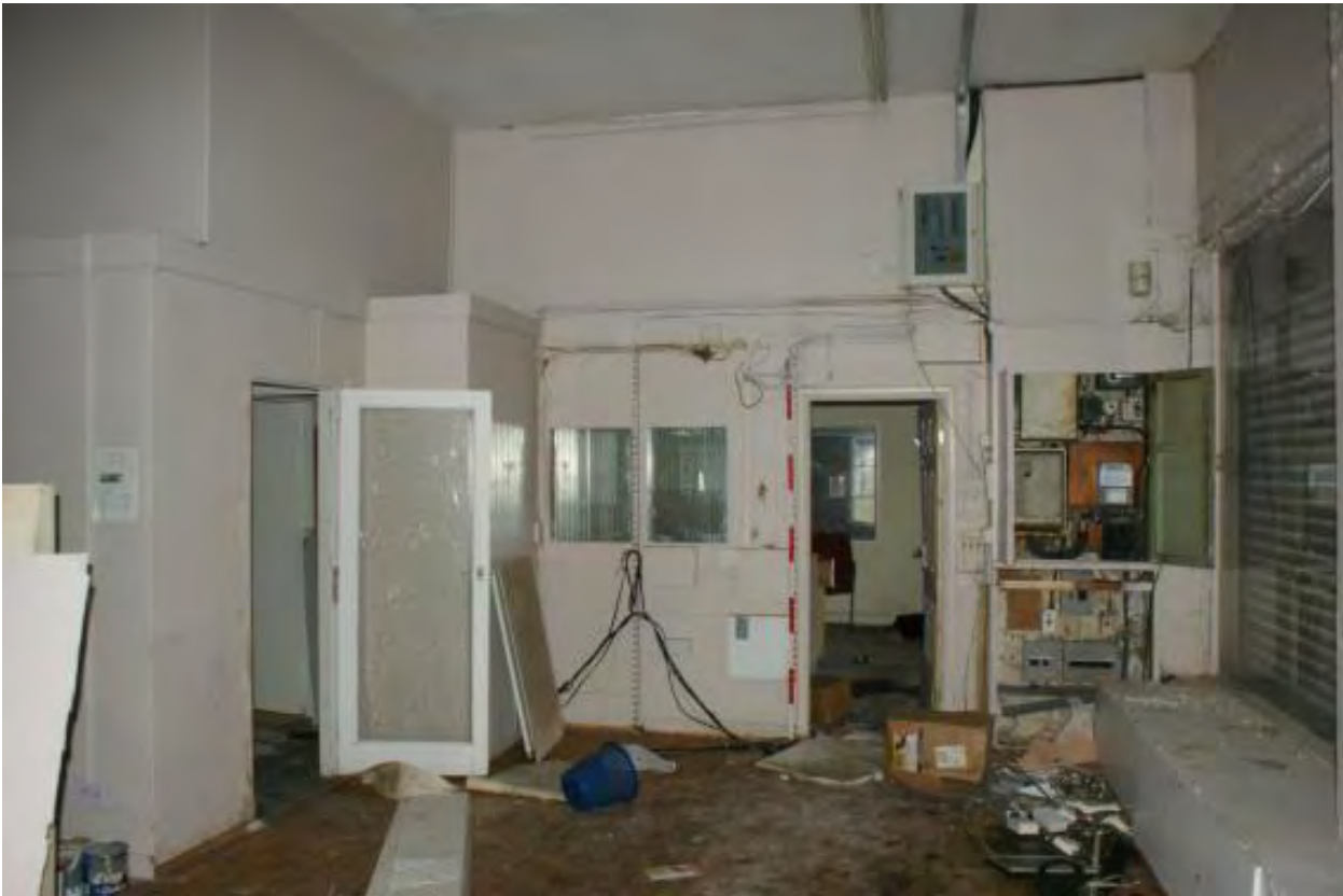
Plate 70 Structure 22, looking east
