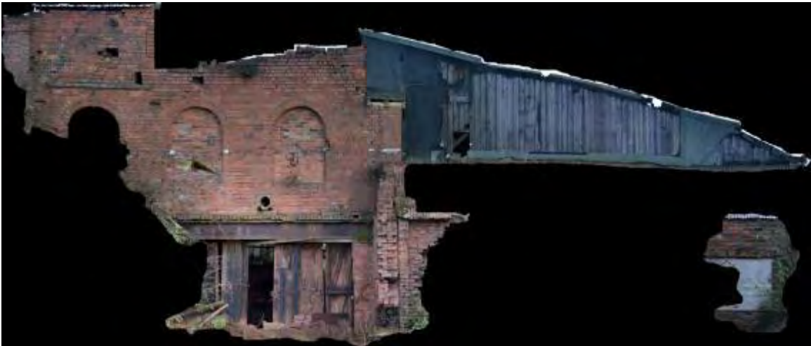
Plate 25 Structure 11/12, looking east
