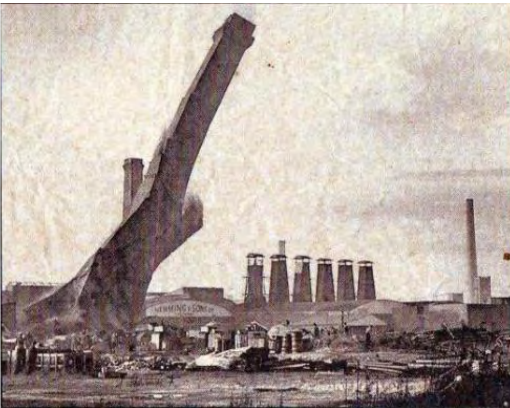
Plate 2 Destruction of a chimney, possibly 1960s (Historic Coventry Forum 2016)
