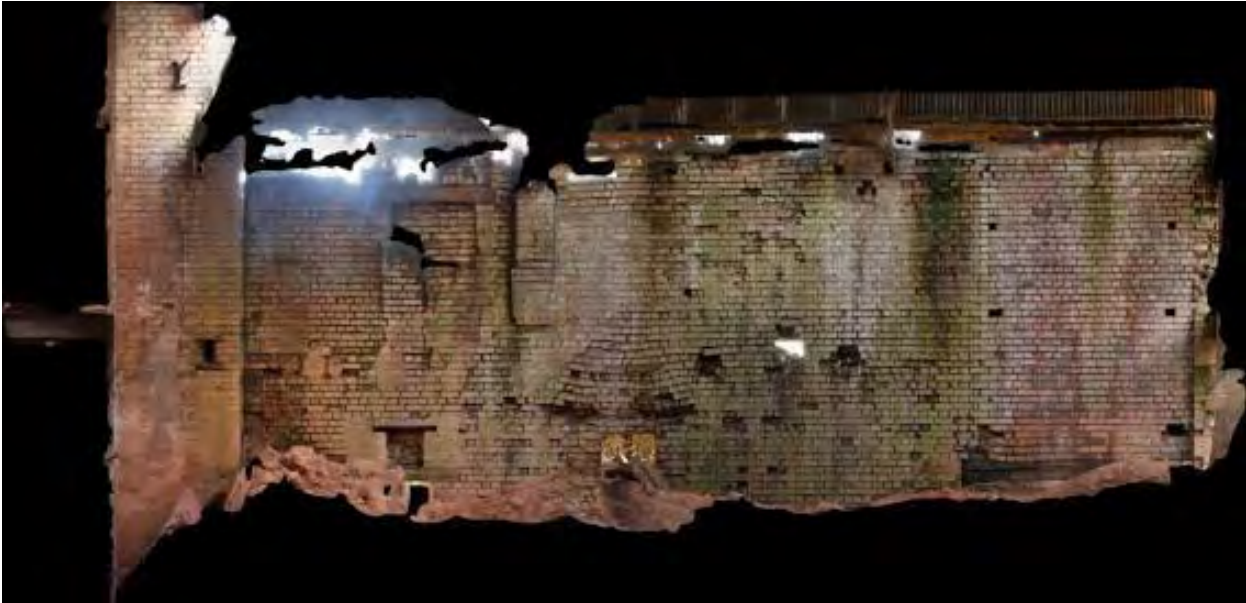
Plate 28 Structure 12, looking south
