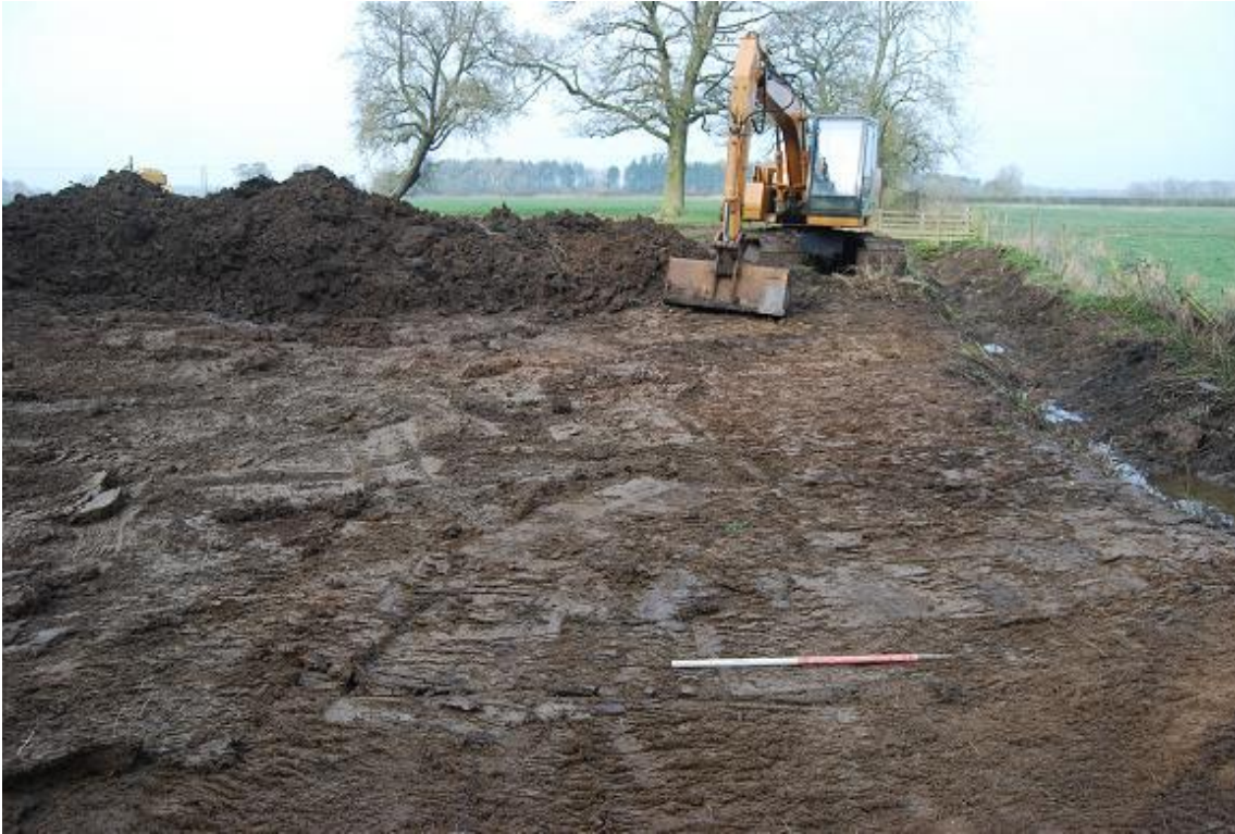
Plate 5 Trench 5 (soil strip), looking west
