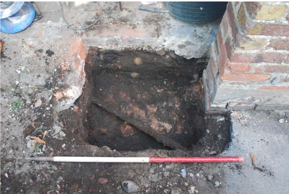
Plate 4 Trench 5 showing metal service pipe, wall footing and made ground; view north, scale 1m
