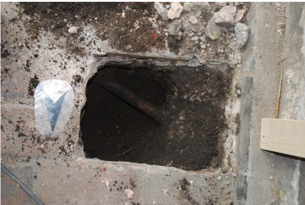
Plate 2 Trench 2 with concrete and brick floor and metal service pipe
