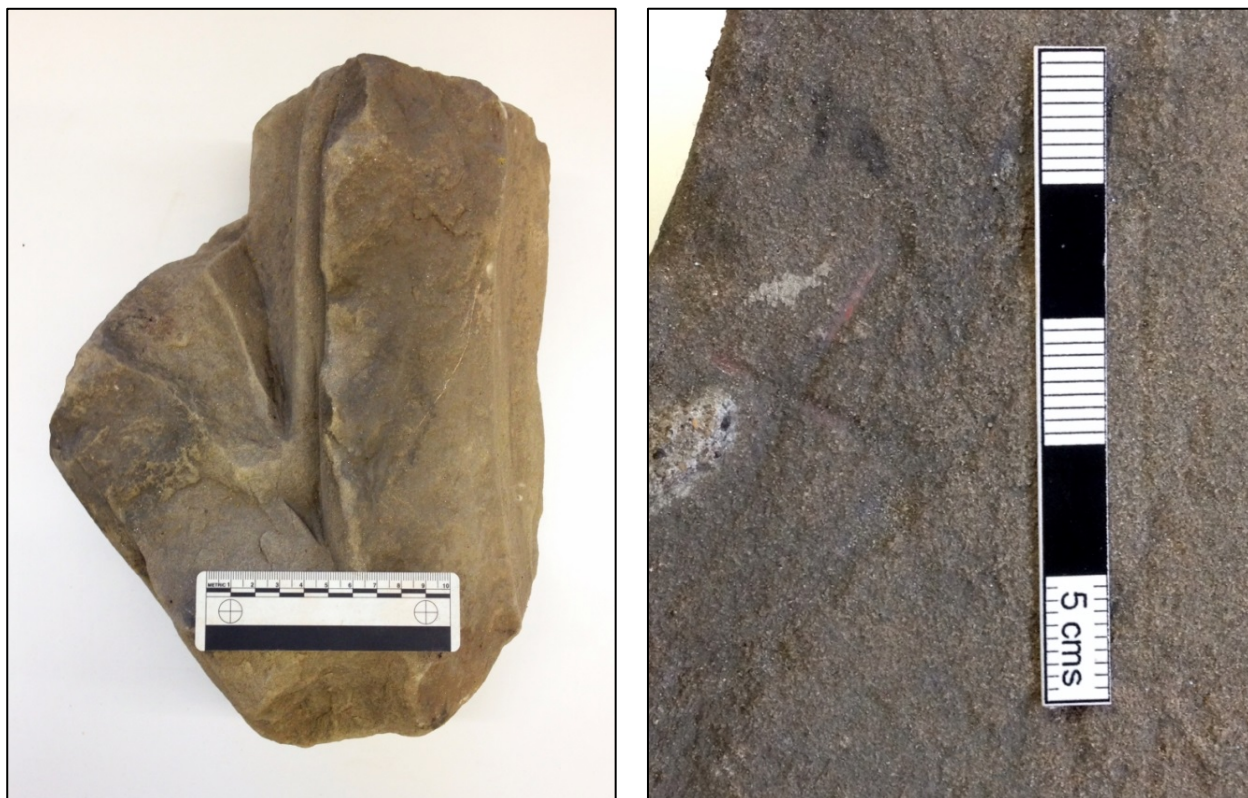
Plate 47 (left): Well-weathered green sandstone tracery, probably from late 15th century South Clerestory
