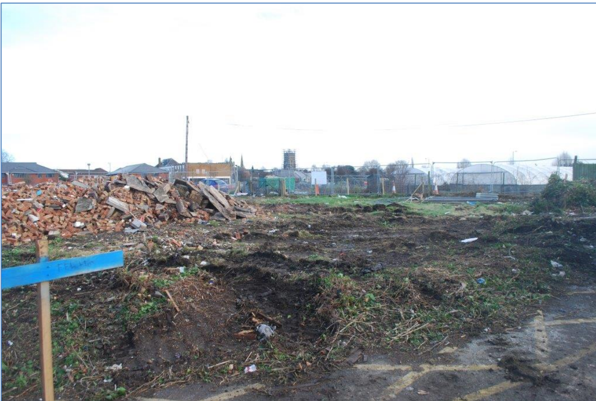
Plate 2: Area 2 during demolition phase, prior to excavation; view north-east
