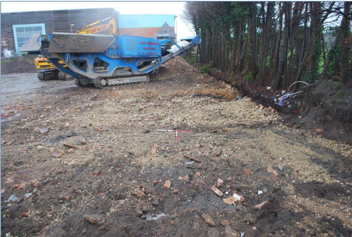
Plate 3: Area 1 with hardstanding removed, to finished depth; view west
