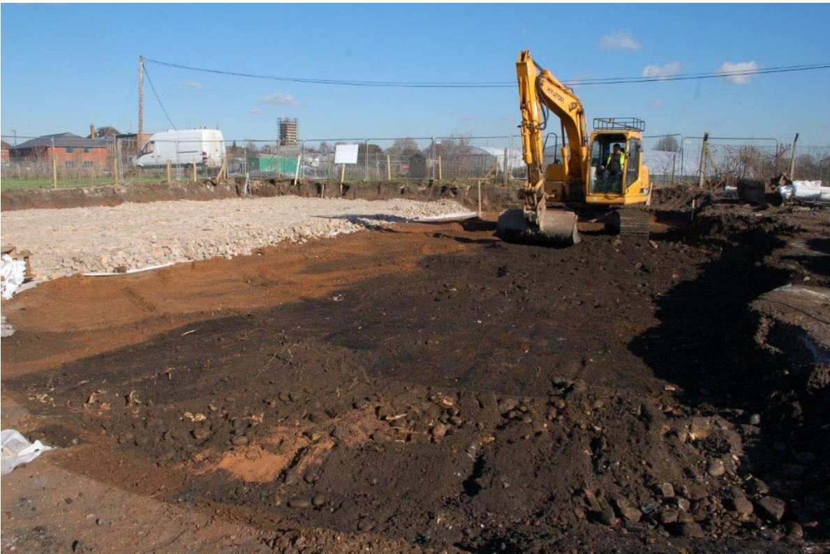
Plate 8: Made ground deposit in southern extent of Area 2; view north-east
