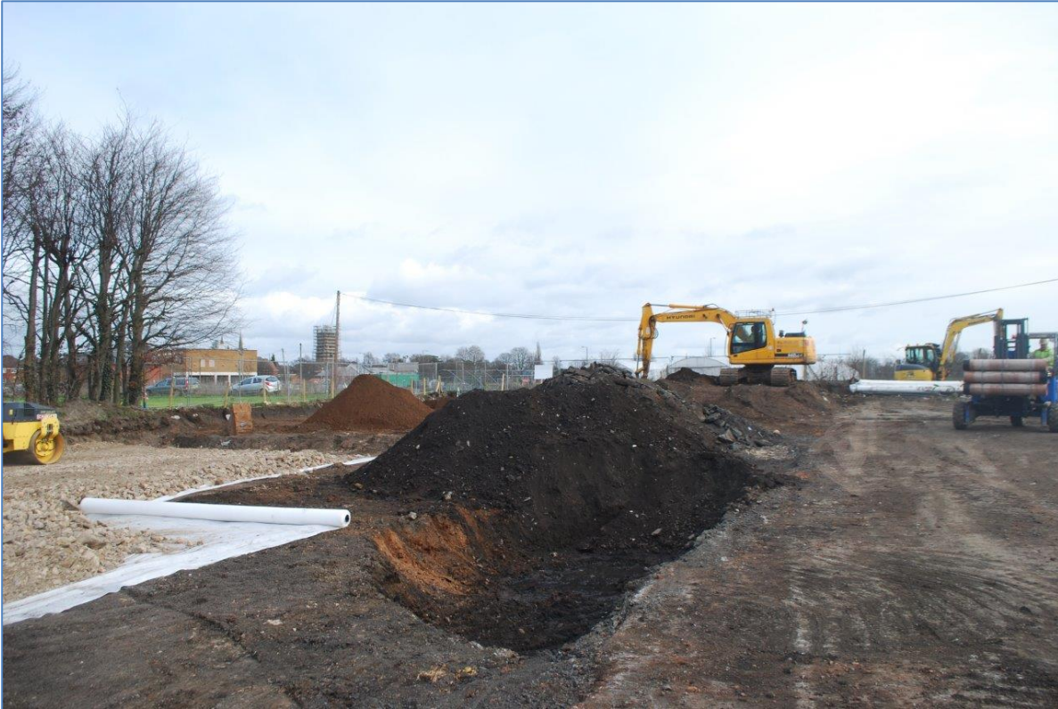
Plate 5: Pit 104 excavated to final depth; view north-east
