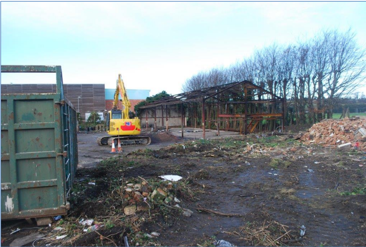
Plate 1: Area 1 during demolition phase prior to excavation; view north-west
