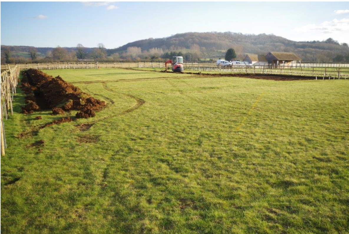
Plate 5 The site showing open trenches, looking south
