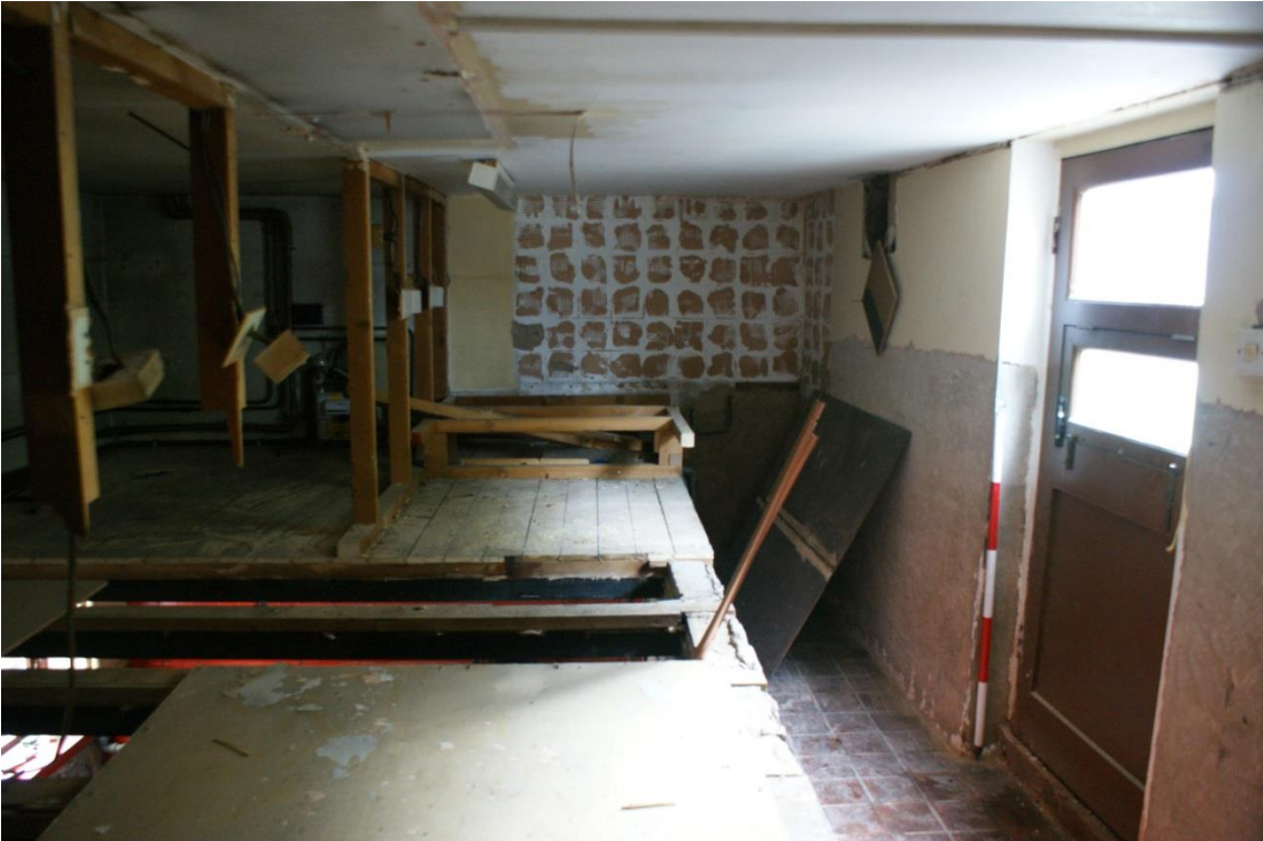
Plate 37 Phase 6 Structure 2, looking east
