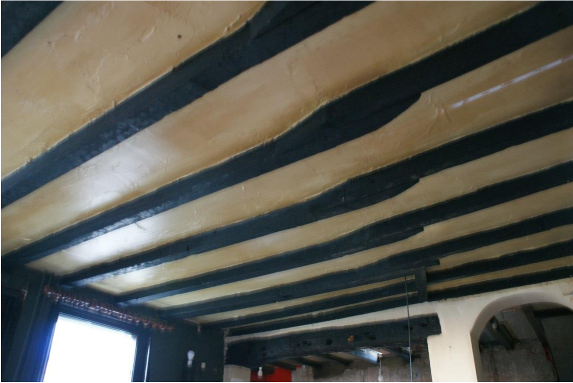
Plate 14 Phase 3 Structure 1, looking south-east
