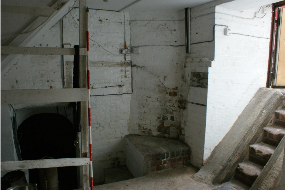
Plate 6 Phase 1 Structure 9, looking south-east
