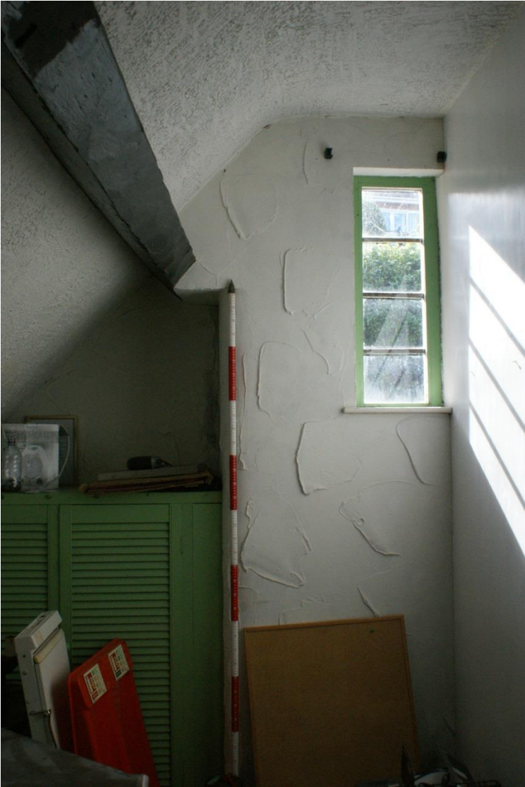
Plate 44 Phase 8 Structure 11, looking south
