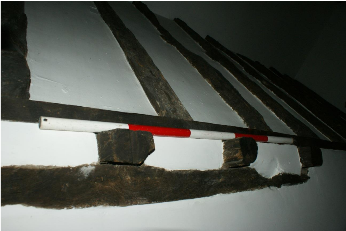
Plate 8 Phase 2 Structure 12, looking south-west
