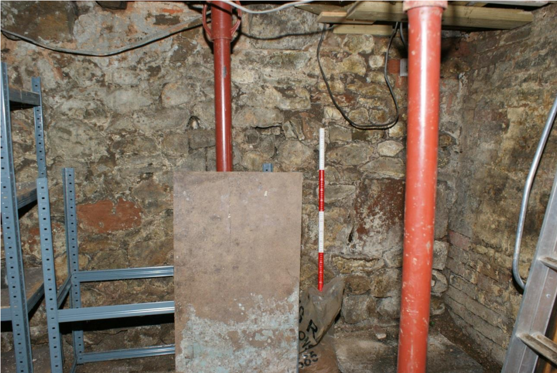
Plate 21 Phase 4 Structure 3, looking south
