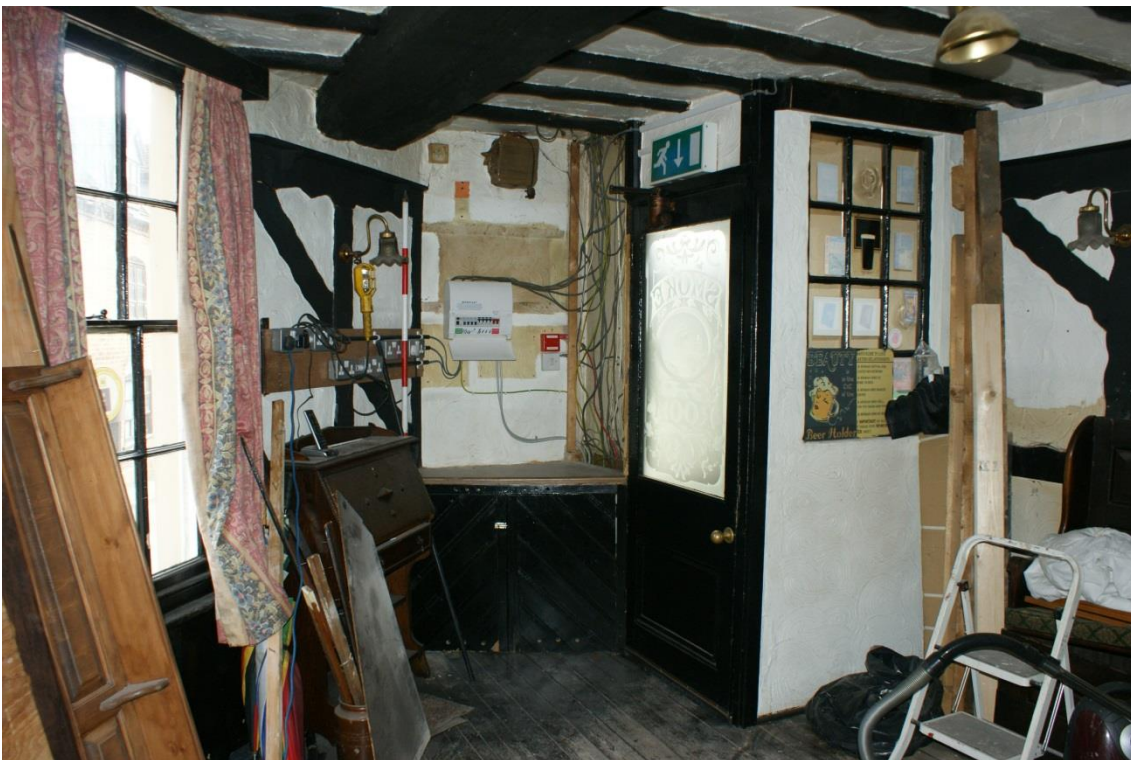
Plate 18 Phase 4 Structure 3, looking south-east
