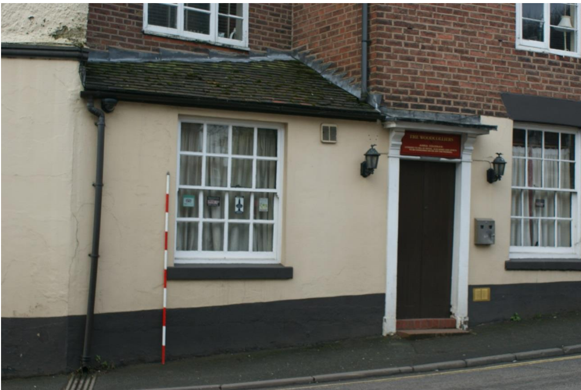
Plate 33 Phase 5 Structure 5, looking south
