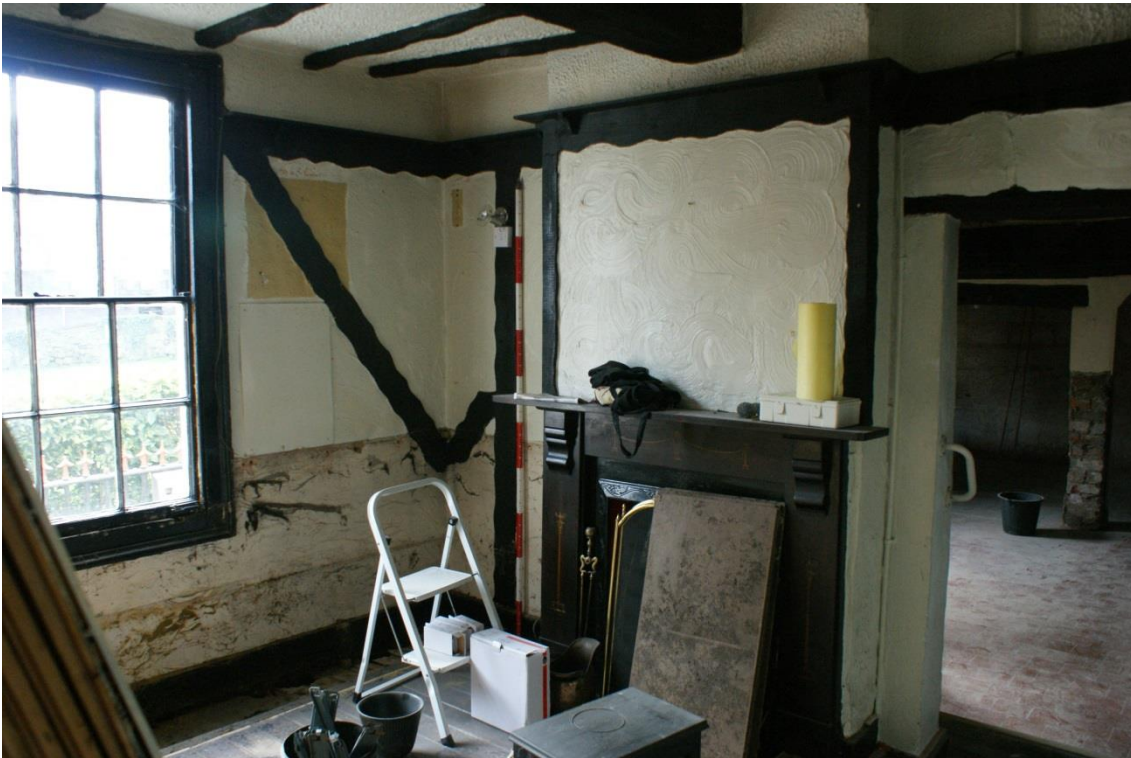
Plate 19 Phase 4 Structure 3, looking south-east
