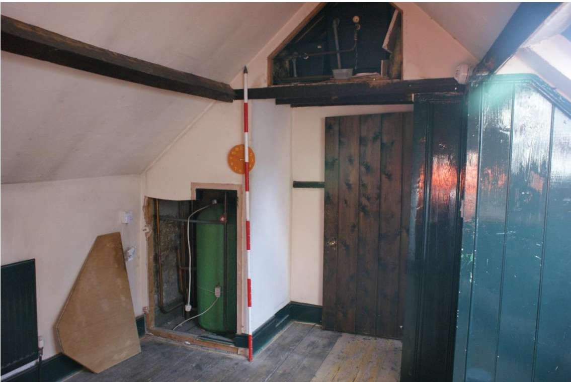
Plate 16 Phase 3 Structure 1, looking sout
