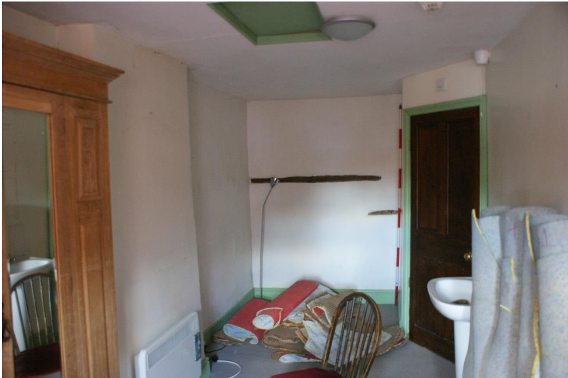
Plate 24 Phase 5 Structure 7, looking south
