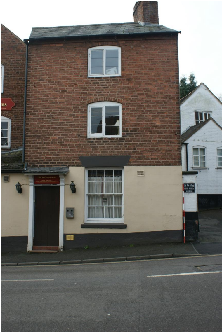
Plate 29 Phase 5 Structure 6, looking south
