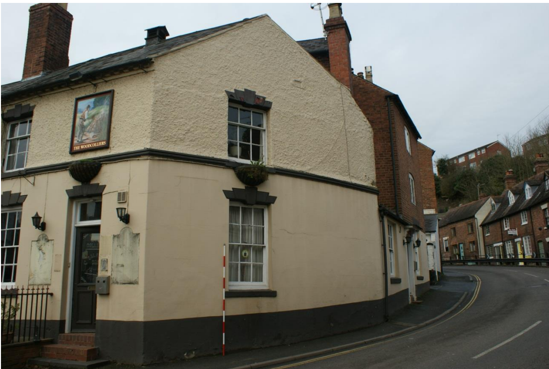
Plate 39 Phase 7 Structure 4, looking south-west
