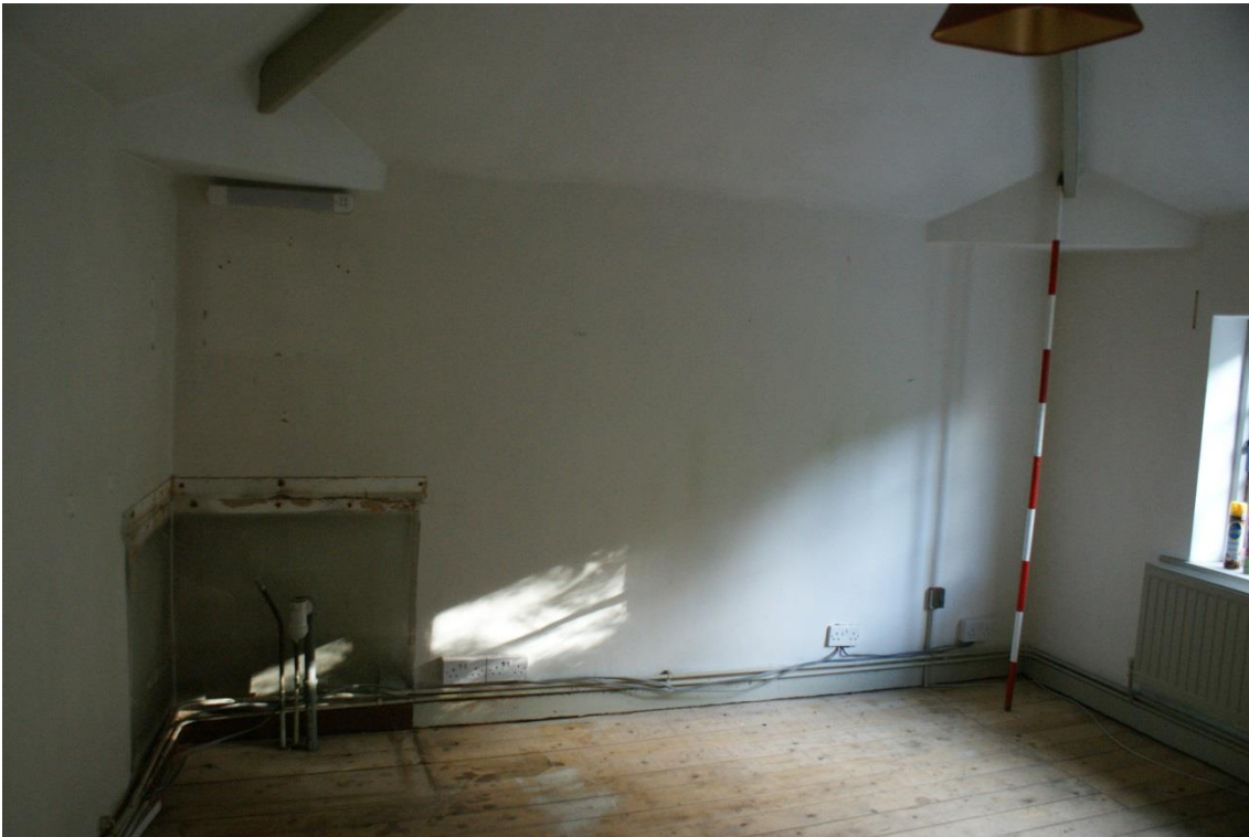
Plate 38 Phase 6 Structure 2, looking east
