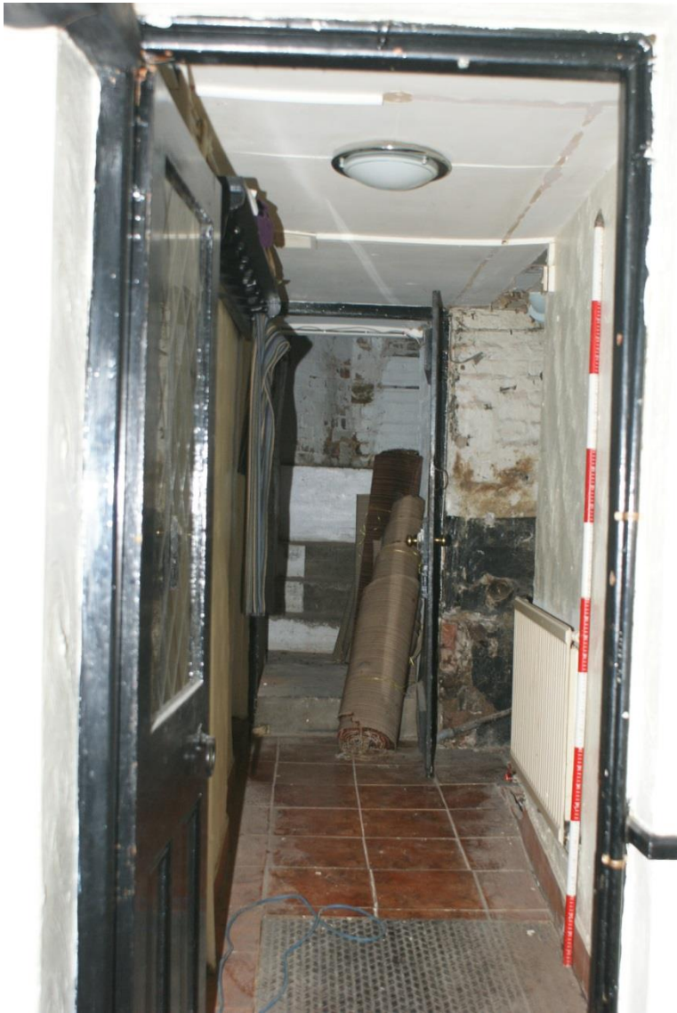
Plate 45 Phase 9 1980s toilet block, looking south
