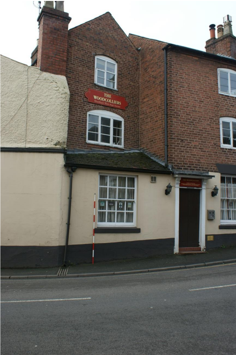
Plate 23 Phase 5 Structure 7, looking south-west
