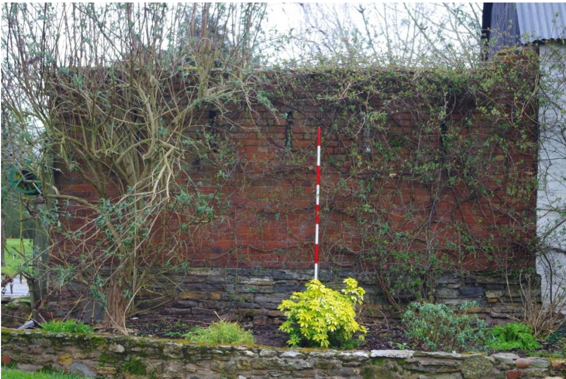
Plate 4 Phase 1 barn, looking east
