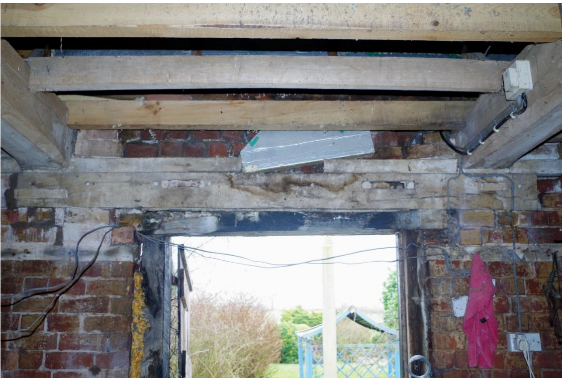
Plate 16 Phase 2 stabling, looking south
