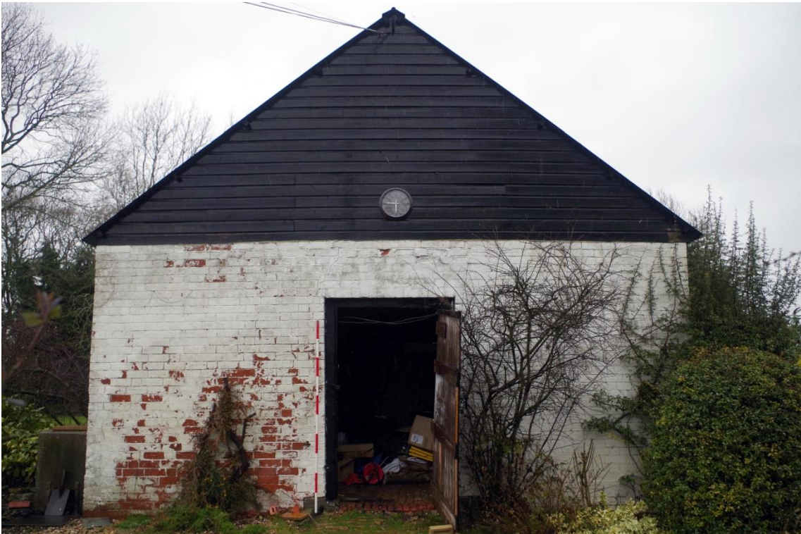
Plate 11 Phase 2 stabling, looking north
