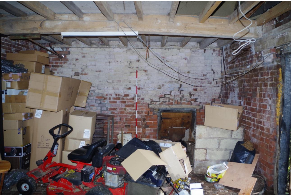
Plate 15 Phase 2 stabling, looking east
