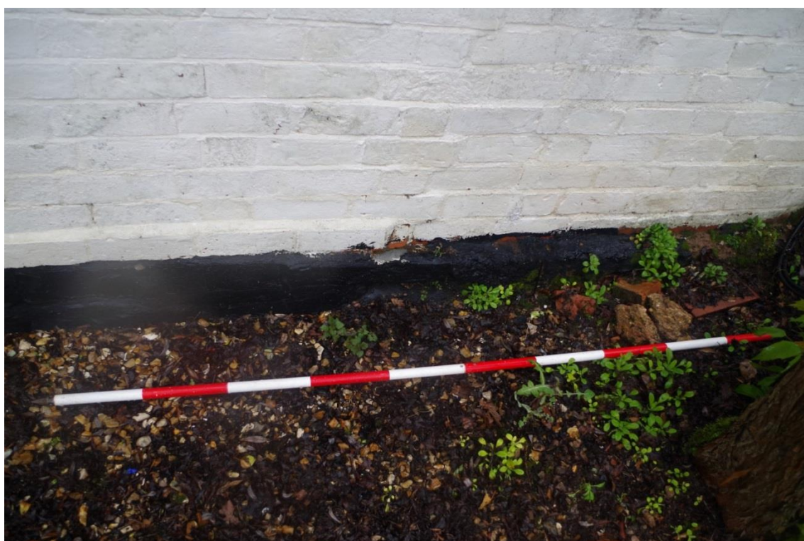
Plate 8 Phase 2 stabling foundation, looking north-west
