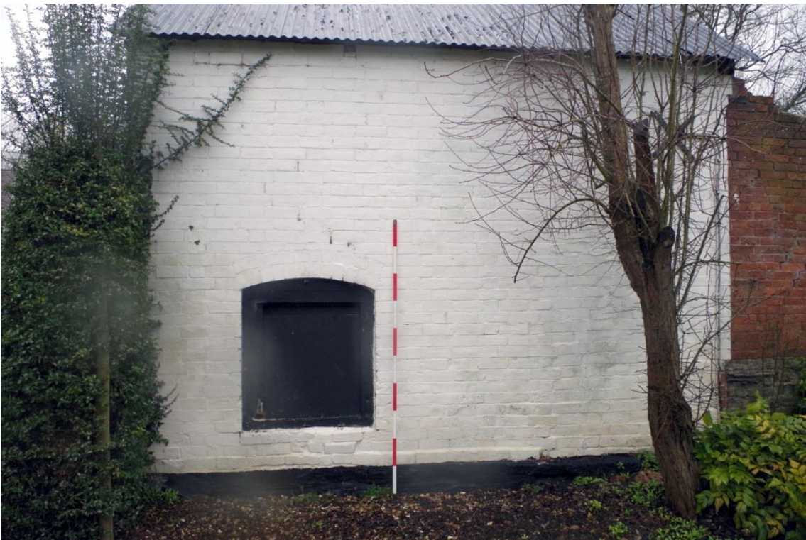
Plate 10 Phase 2 stabling, looking west
