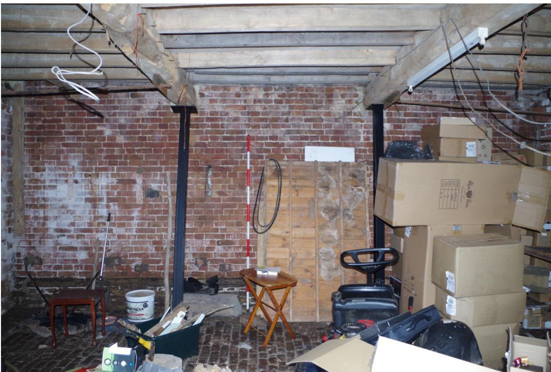
Plate 14 Phase 2 stabling, looking north
