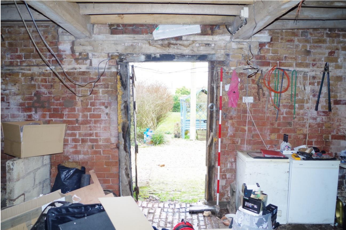
Plate 12 Phase 2 stabling, looking south
