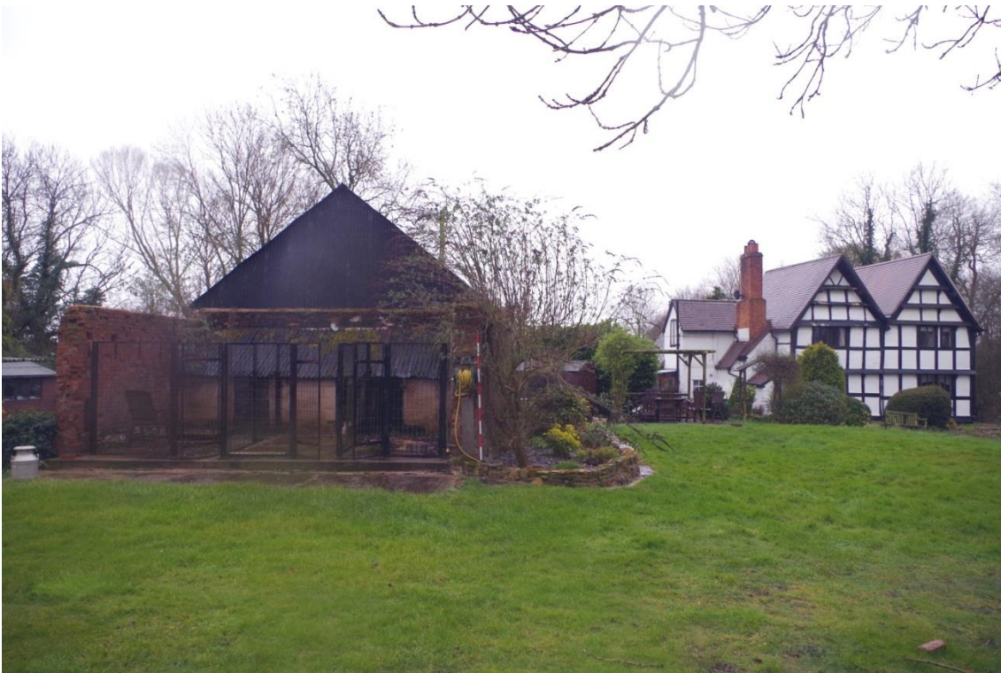
Plate 1 The building and house, looking south
