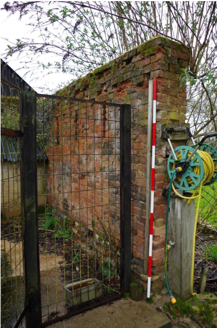
Plate 6 Phase 1 barn former entrance, looking south-west
