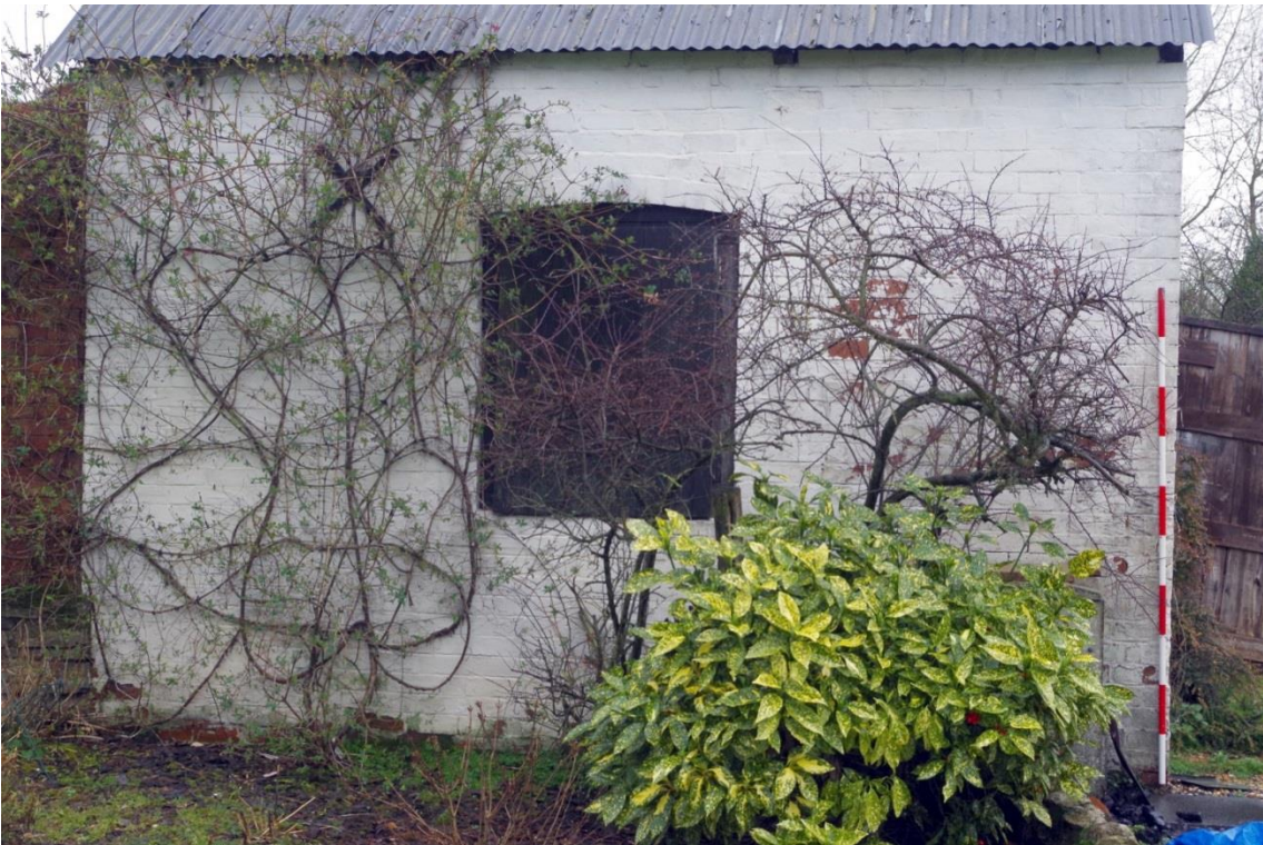
Plate 9 Phase 2 stabling, looking east
