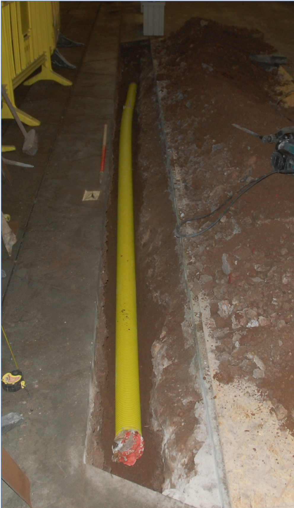
Plate 4 southern c7m stretch of Trench 1, scale 1m, view north
