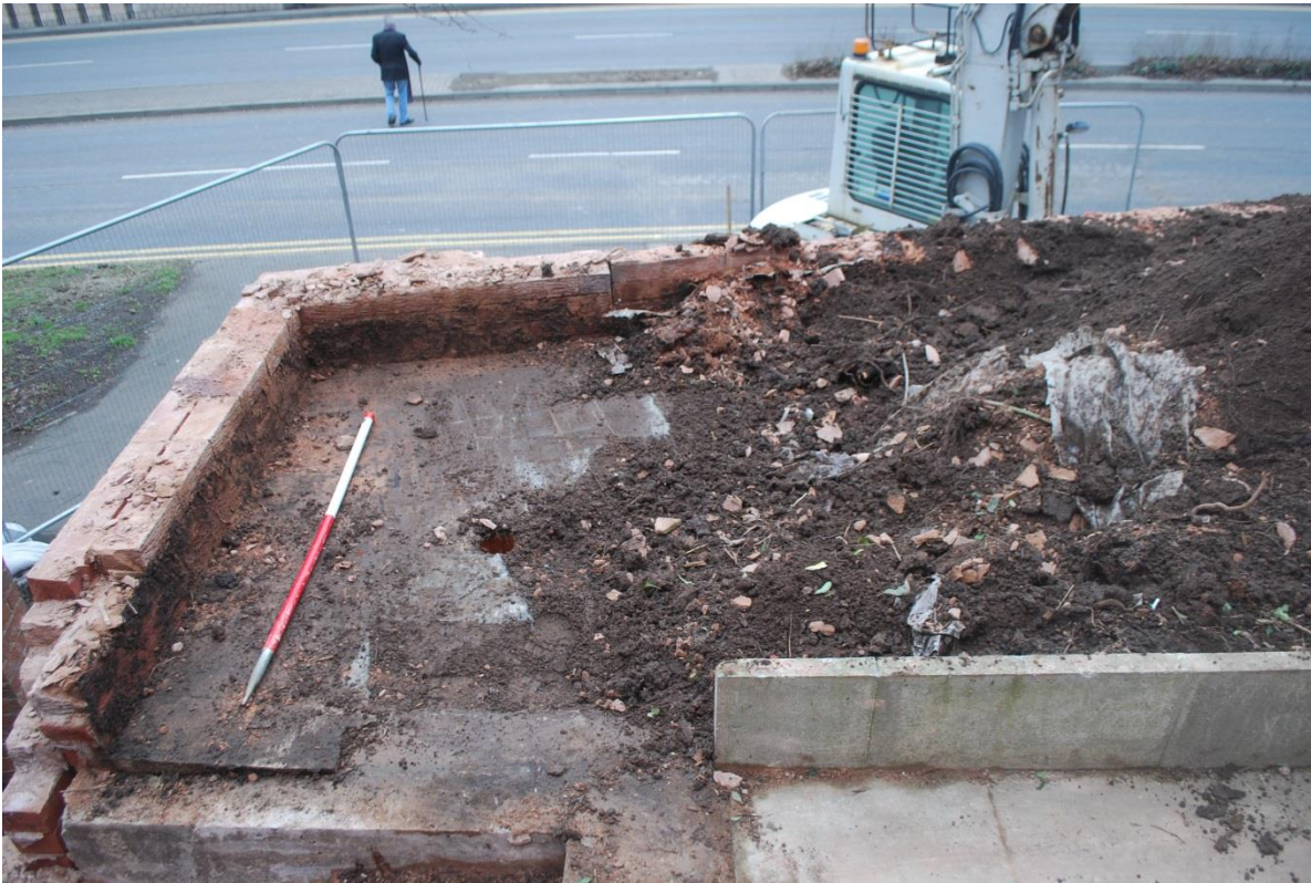
Plate 3: The concrete pad and drain beneath the flowerbed topsoil. View east.
