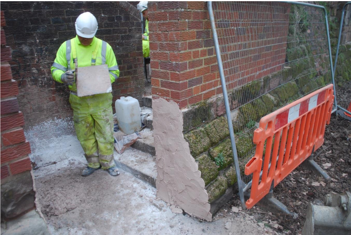
Plate 10: Sandstone wall covered by lime mortar fillet prior to concreting stairwell.
