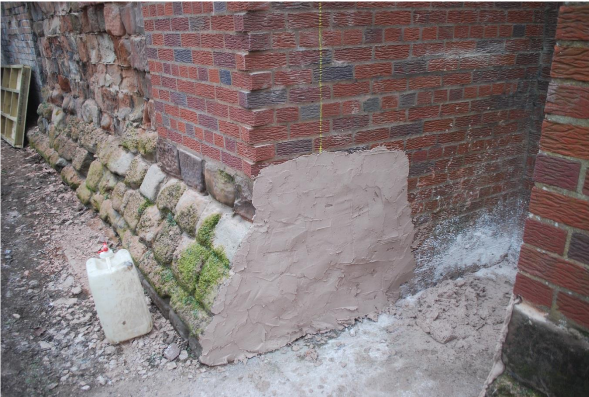
Plate 9: Sandstone wall covered by lime mortar fillet prior to concreting stairwell.
