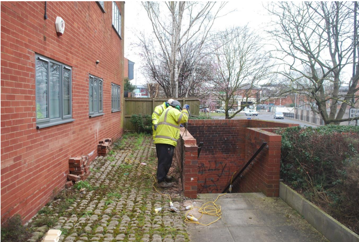
Plate 1: Beginning reduction of the brick stairwell, parapet
