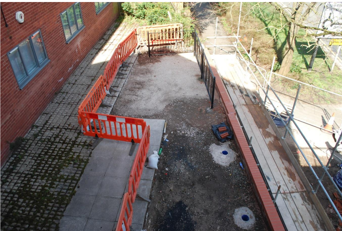
Plate 14: Fencing installed at North end of City Wall.
