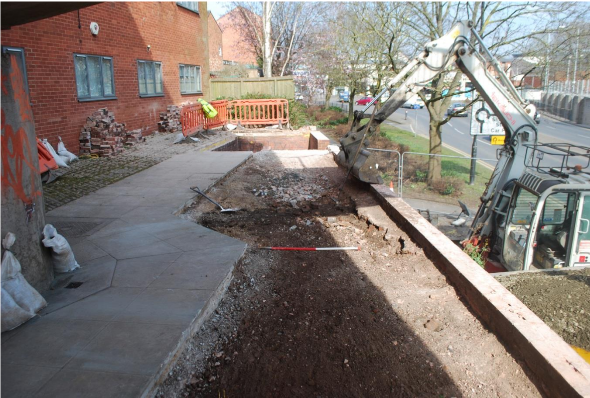
Plate 5: Trench 1 after reductions completed. View north.
