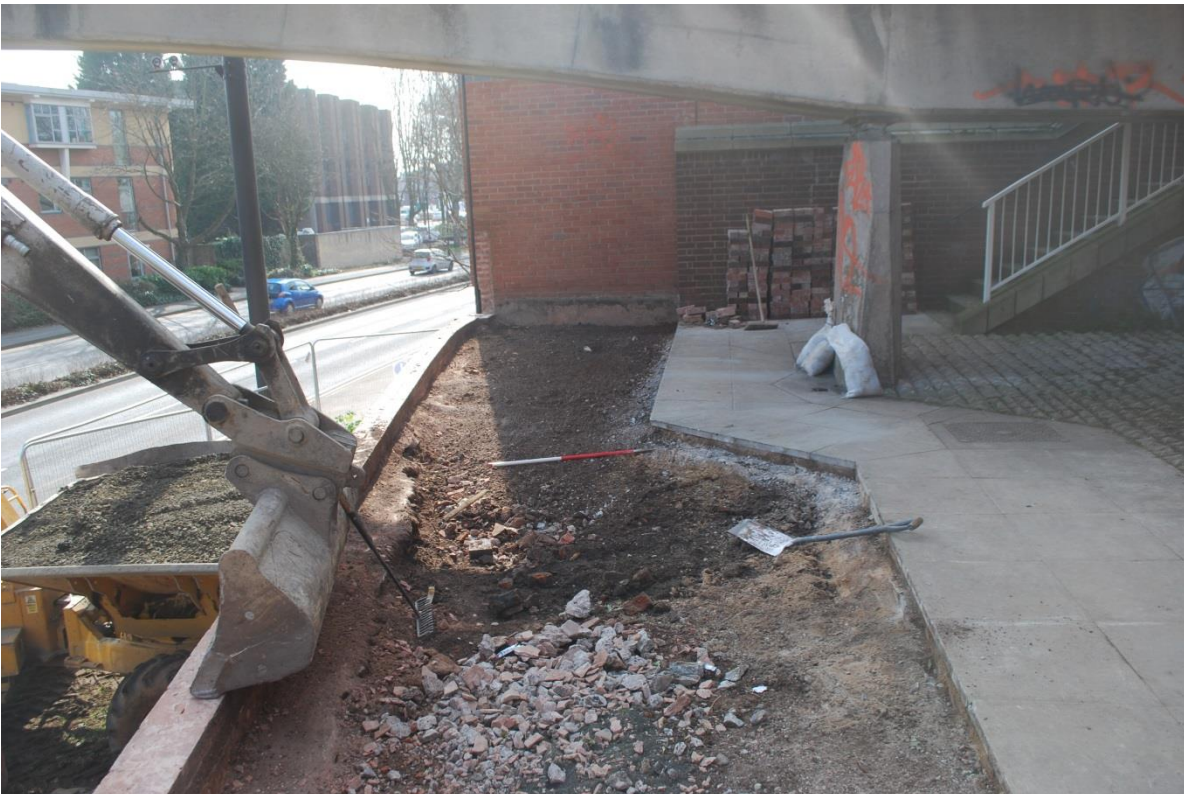
Plate 6: Trench 1 following reduction: View south.
