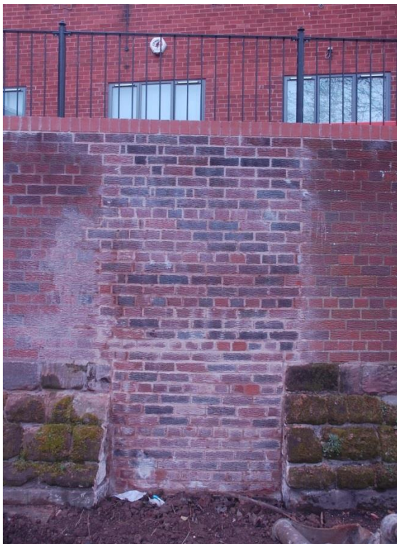
Plate 16: Completed blocked passageway
