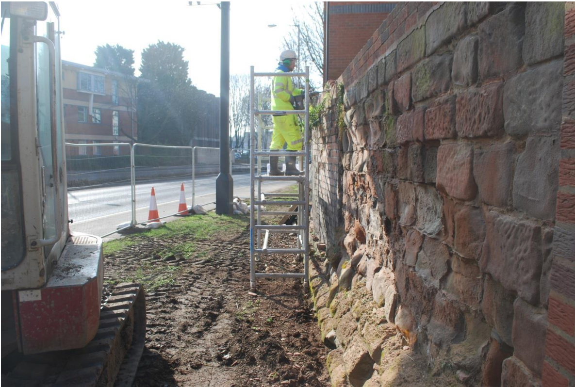
Plate 7: Reducing the brick parapet on a freestanding aluminium scaffold. View south.
