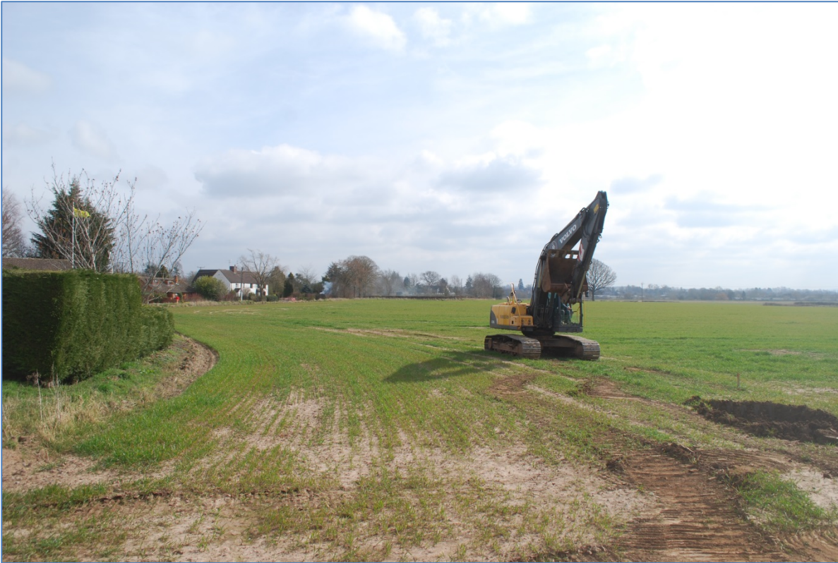
Plate 1: Area 1 looking east prior to excavation (no scales)
