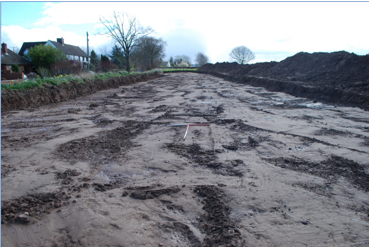
Plate 6: Area 2; western extent after soil strip; view east (2x 1m scales)
