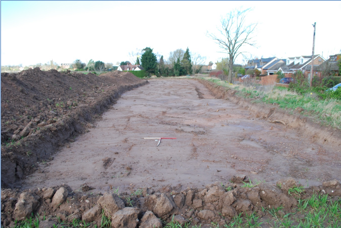
Plate 5: Area 1; eastern extent after soil strip; view west (2x 1m scales)
