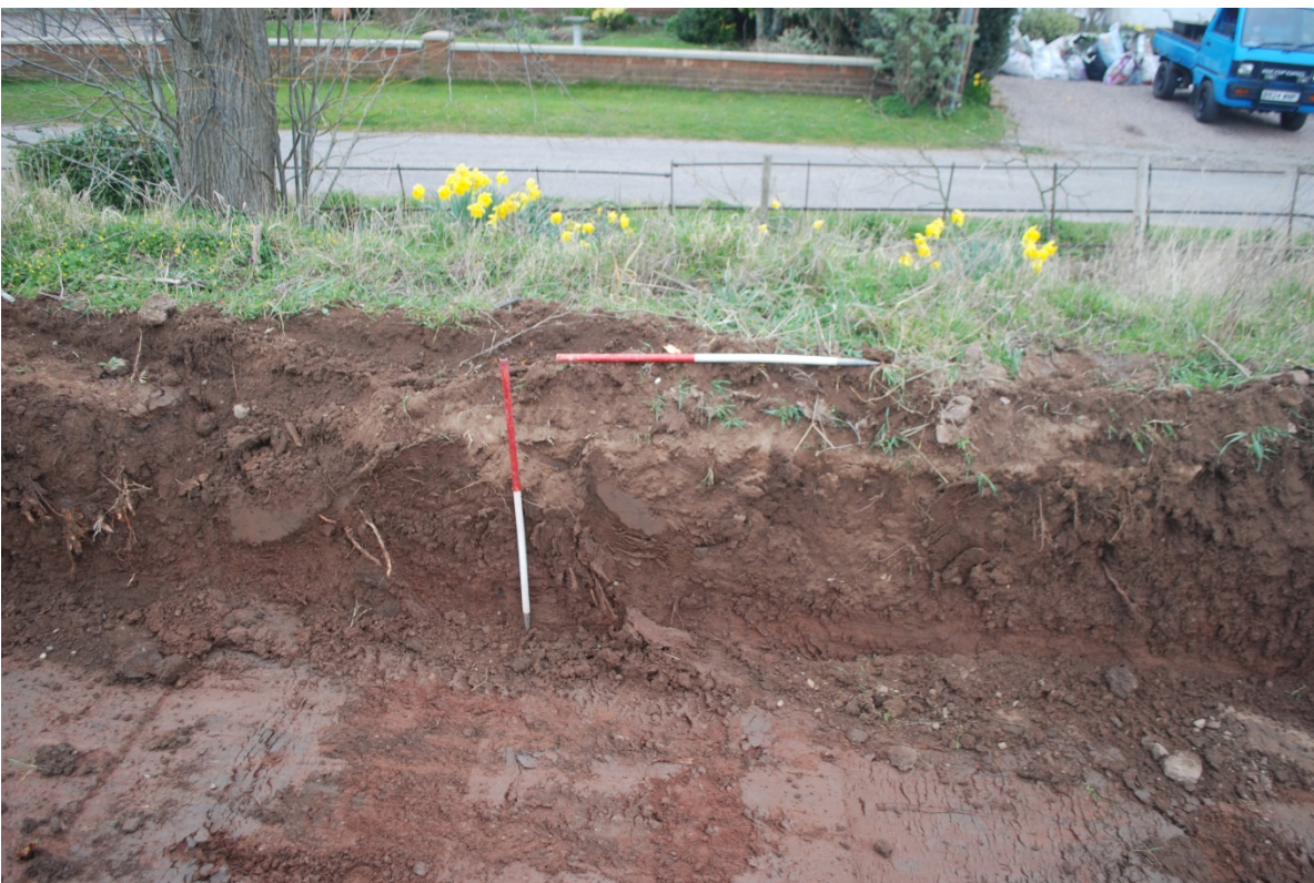
Plate 4: Area 1; deeper section on the northern edge stripped to natural (2x 1m scales)
