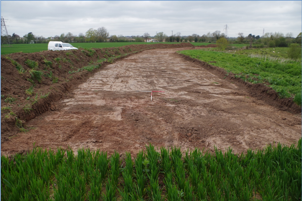
Plate 9: Area 3; eastern extent; view west (2x 1m scales)
