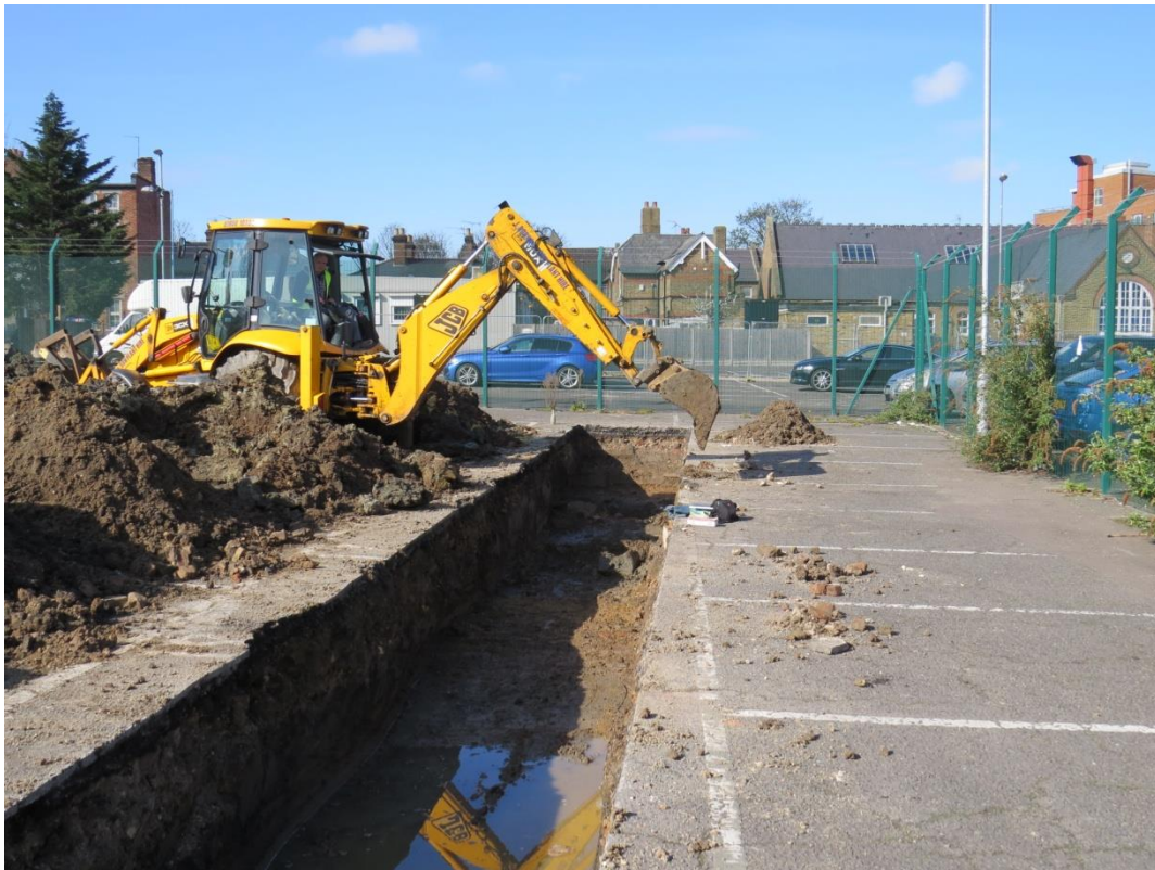
Plate 2. General view of Trench 3, looking westwards towards TP 2.
