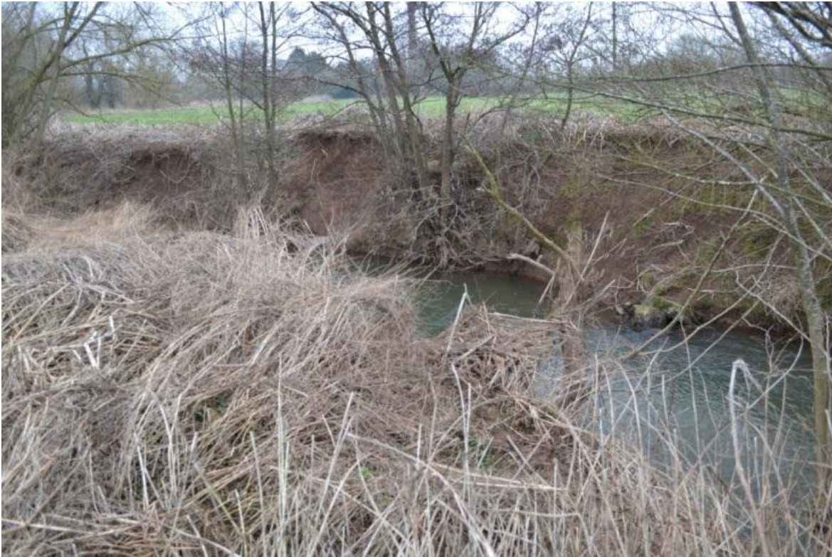
Plate 5 View east over leat, from adjacent to weir
