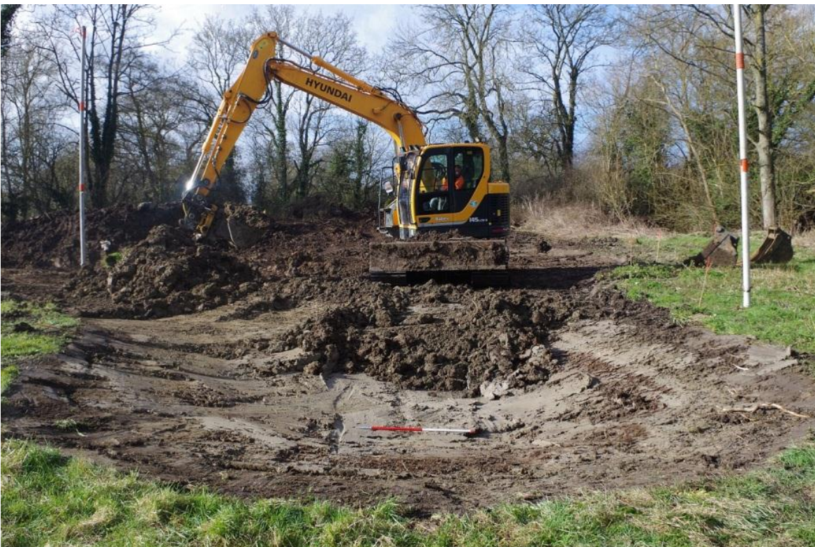
Plate 4; Pond 2 under construction, scale 1m, looking west
