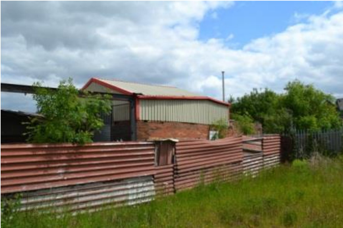
Plate 4 View east-south-east towards industrial buildings
