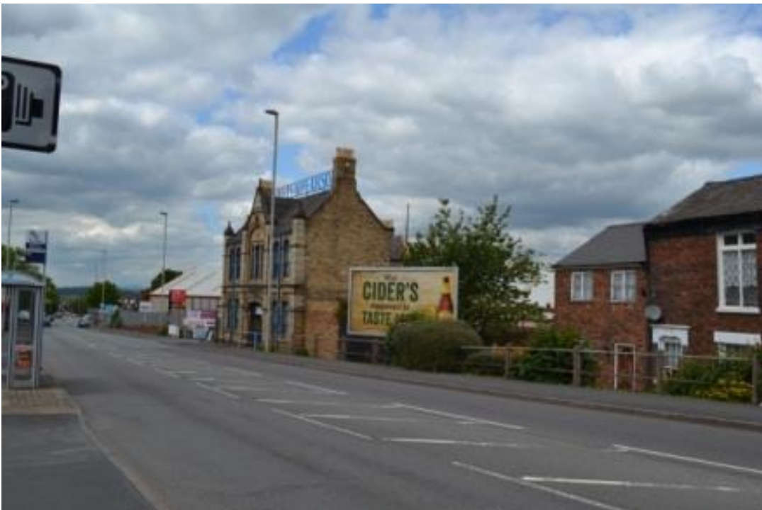
Plate 10 View north-east, showing site with Harris and Pearson building and The Old Crown Inn in the right of the picture
