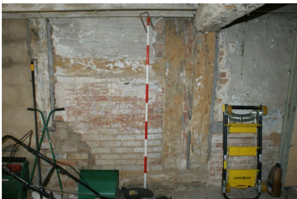
Plate 14 Phase 2 inserted post and beam, looking north-west
