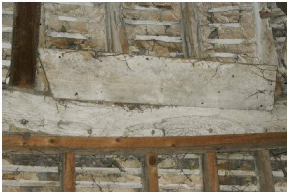
Plate 11 Offset peg holes and rafters in a purlin of the Phase 2 Kitchen, looking north-east
