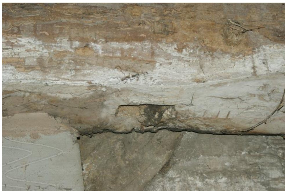
Plate 12 Mortise in the centre of the Phase 2 kitchen gable end frame, looking north-west
