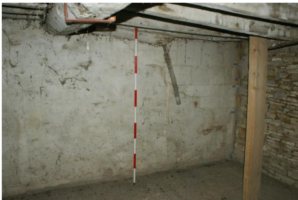
Plate 4 Possible former chimney breast on the former gable of 41 Main Street, looking south-east
