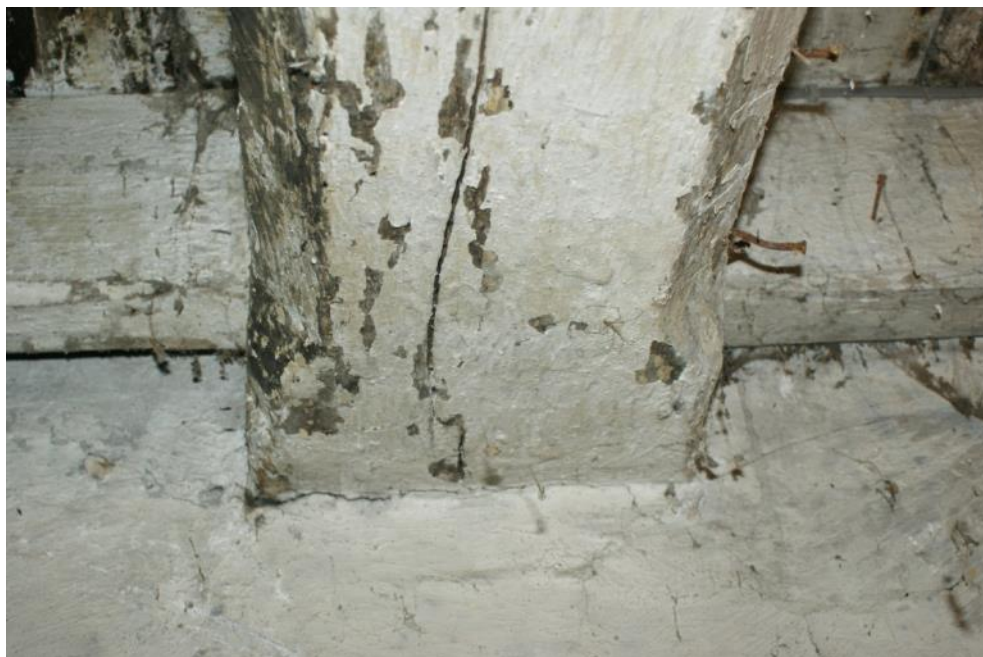
Plate 15 Phase 2 beam with simple chamfers, looking south-east
