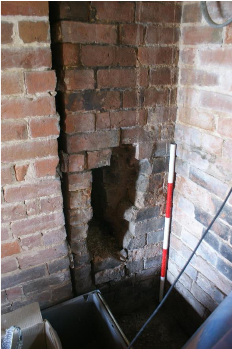
Plate 14 Former chimney flue, looking west
