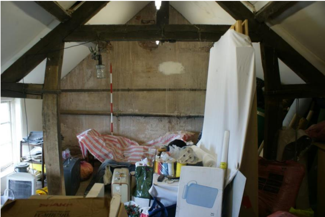
Plate 8 First floor room, looking west
