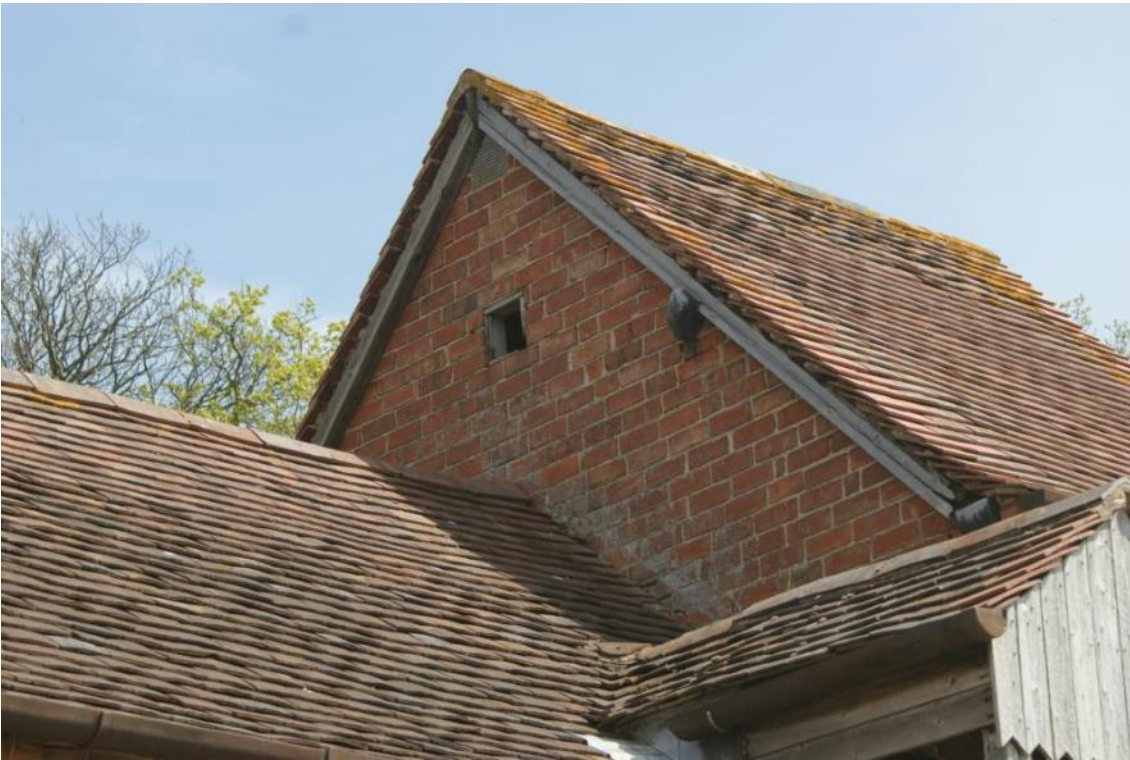
Plate 18 Vent hole in western gable, looking north-east
