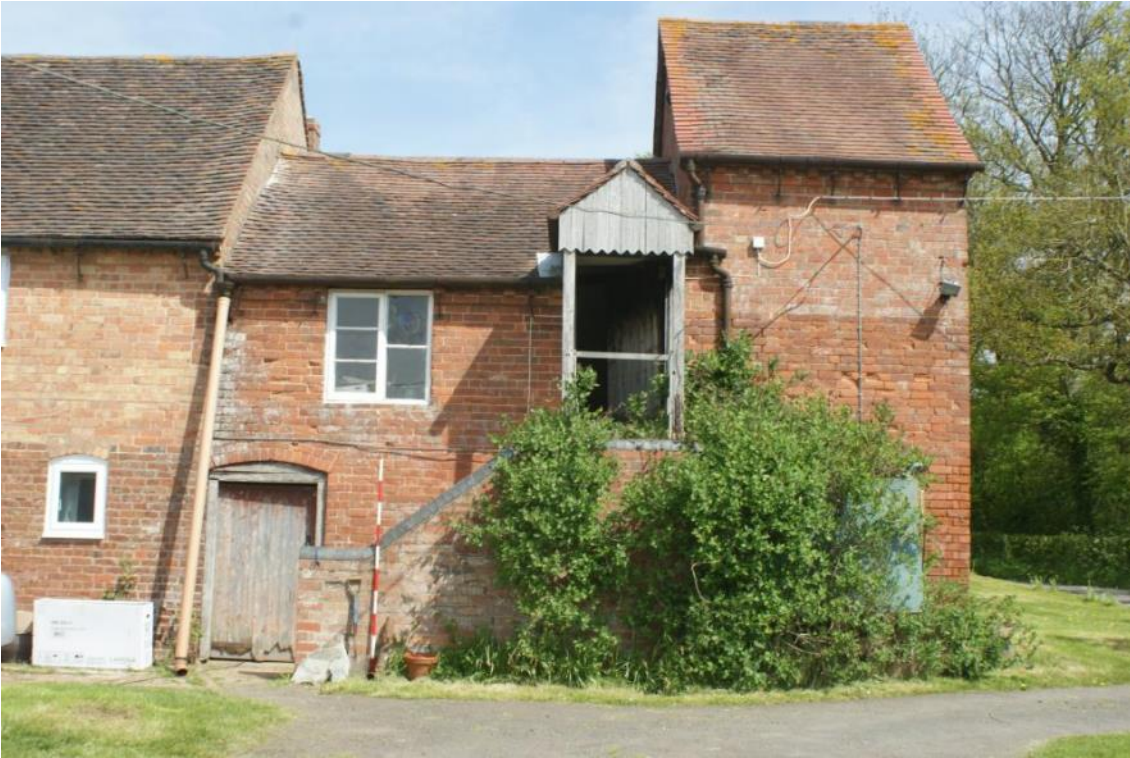
Plate 3 The building, looking north
