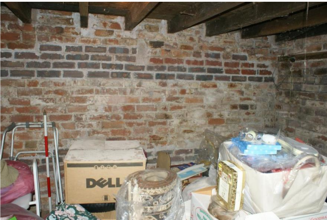
Plate 19 Replaced brickwork visible in smaller first floor room, looking west
