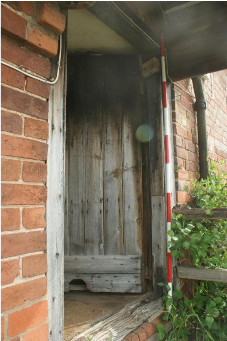
Plate 10 First floor door, looking north-east
