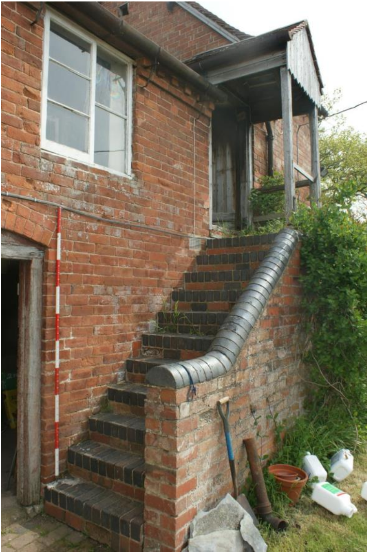
Plate 5 Phase 2 steps, looking north-east
