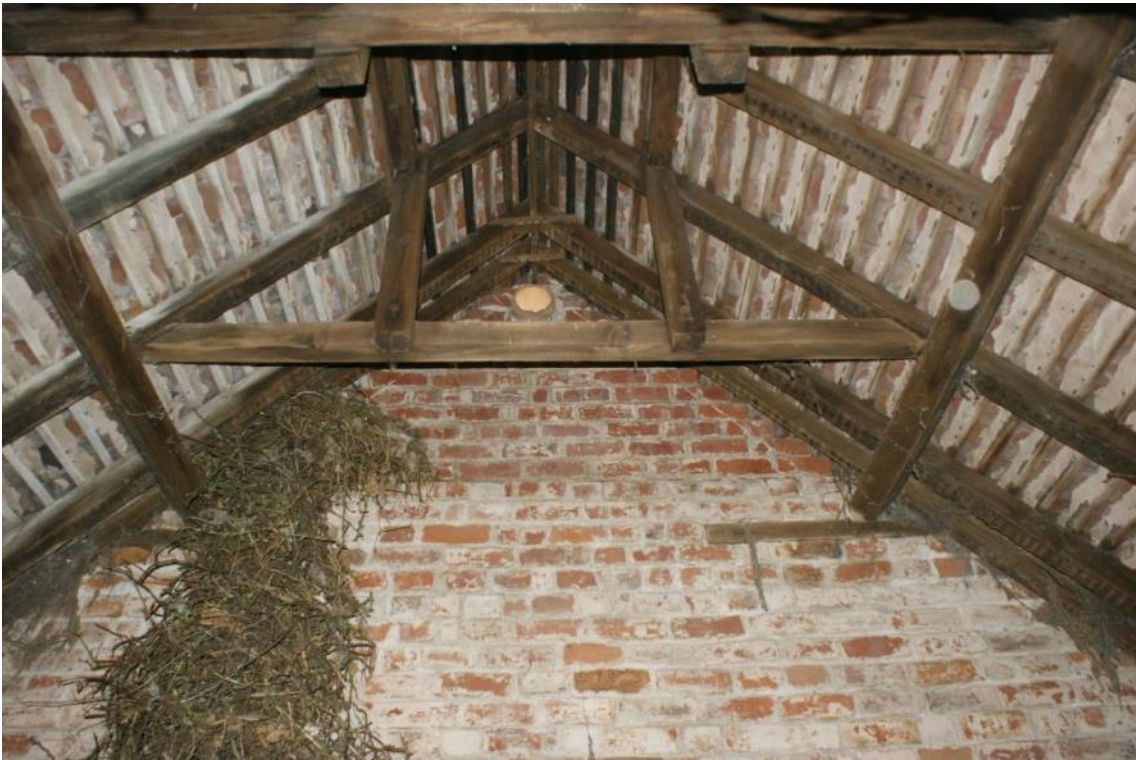
Plate 24 Roof of Phase 2 addition, looking east
