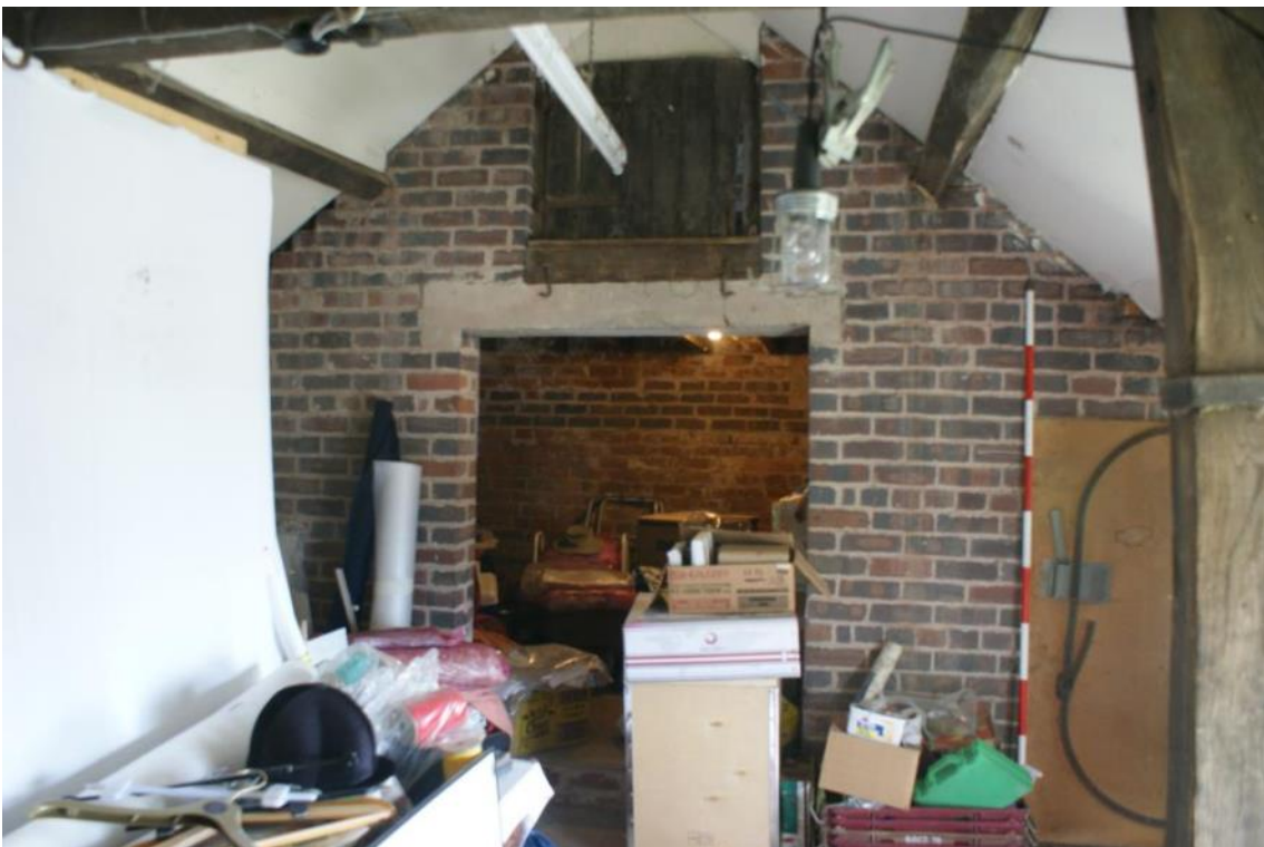
Plate 7 First floor room, looking east
