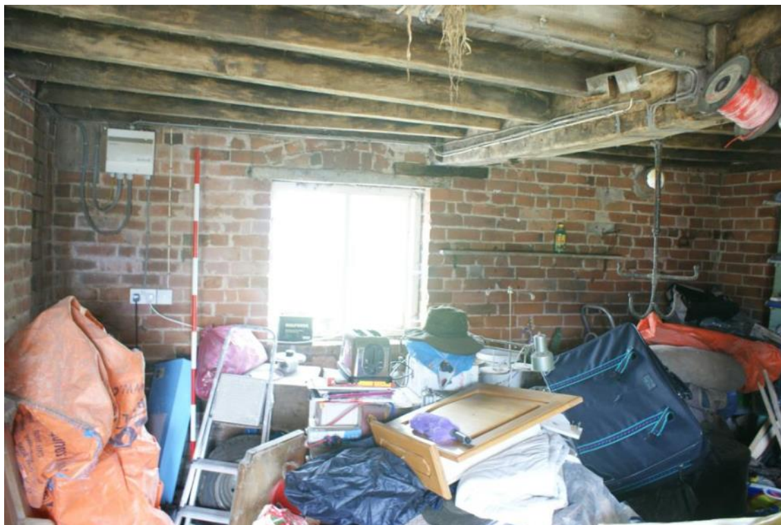
Plate 13 First floor room, looking north
