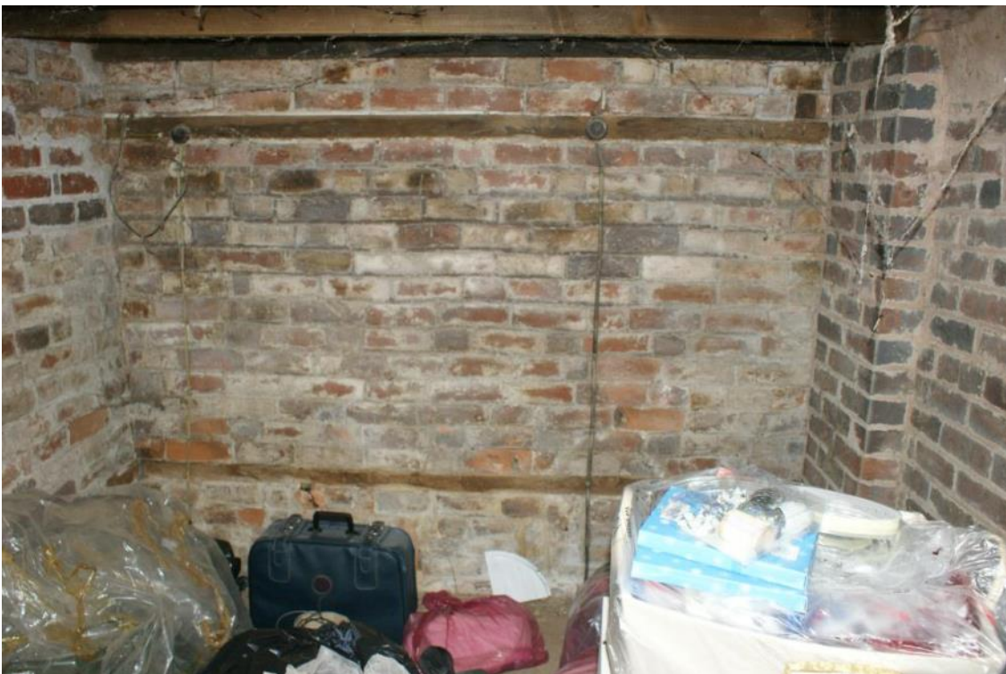
Plate 16 Smaller first floor room, looking south
