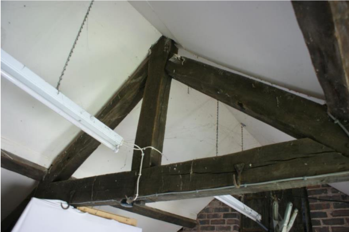
Plate 9 King post truss, looking north-east
