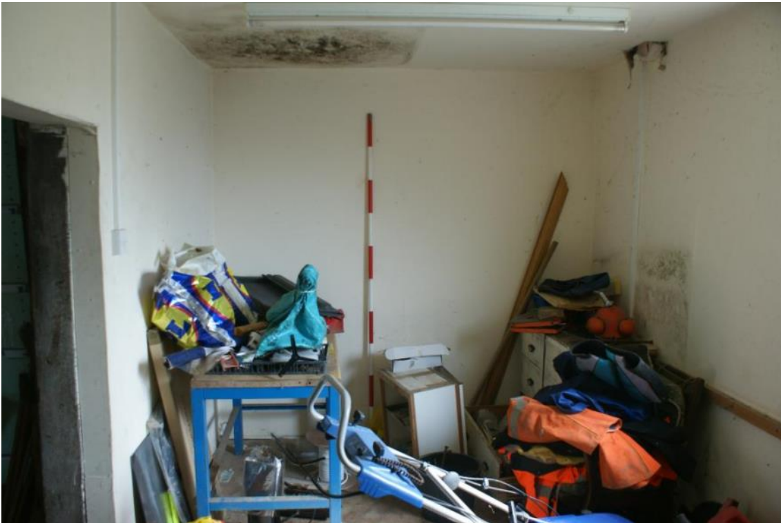
Plate 15 Smaller ground floor room, looking north
