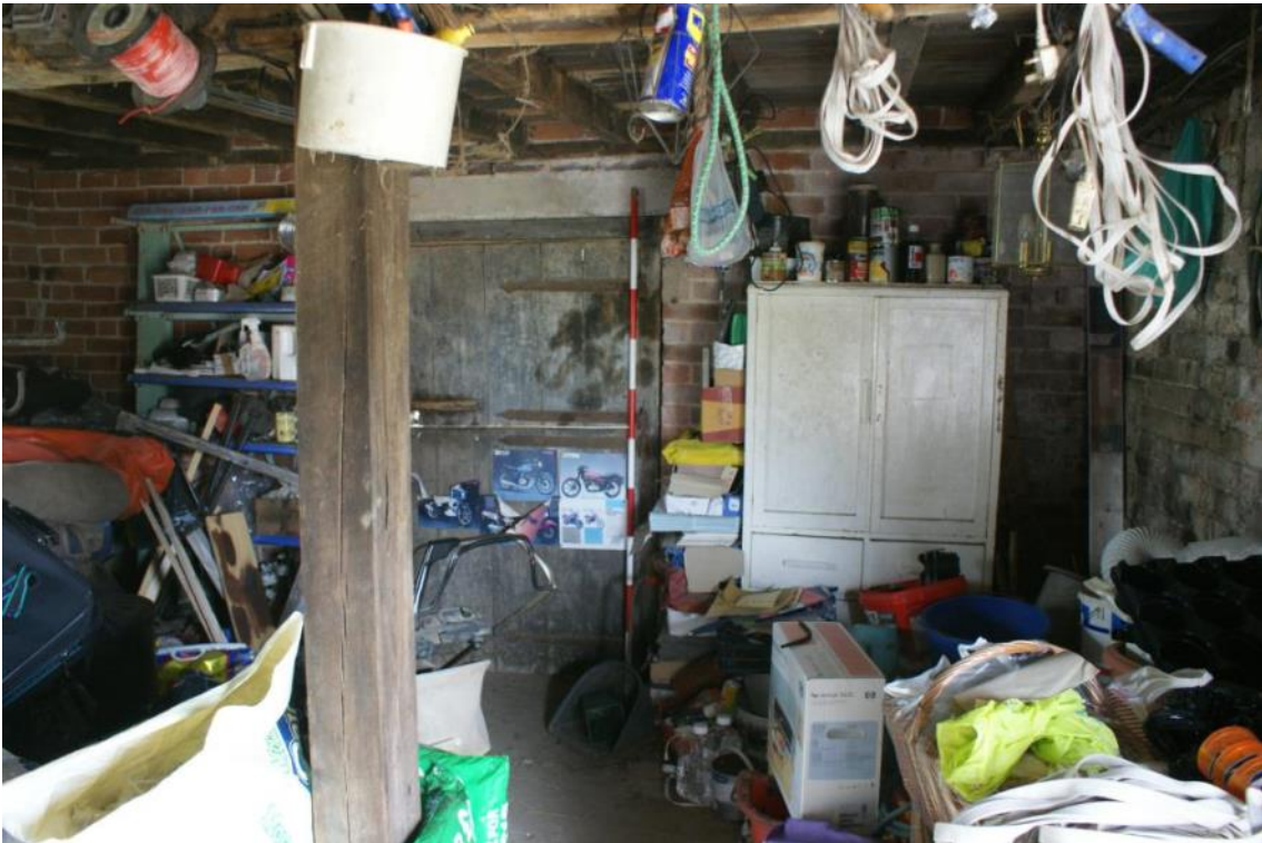
Plate 6 Ground floor room, looking east
