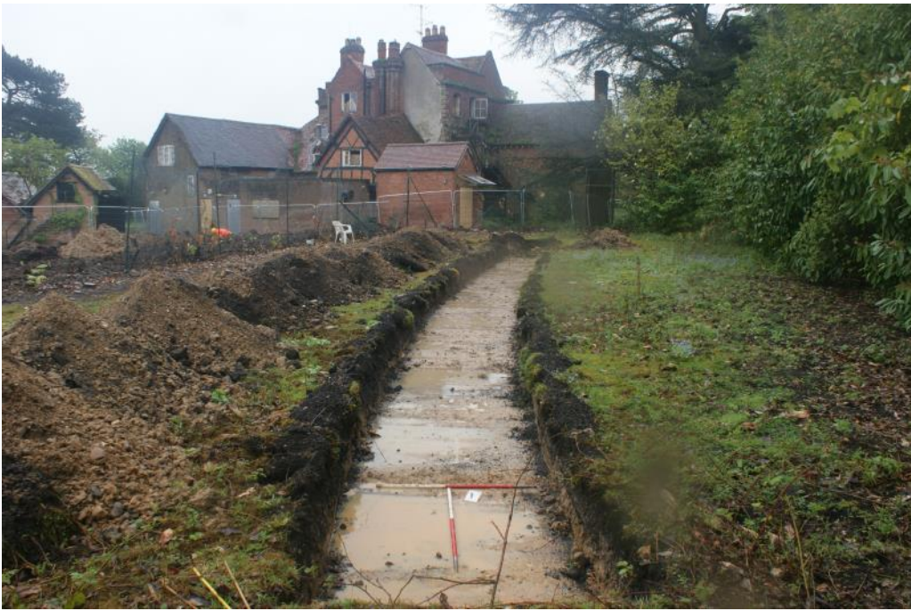
Plate 11 Trench 9 looking south-west
