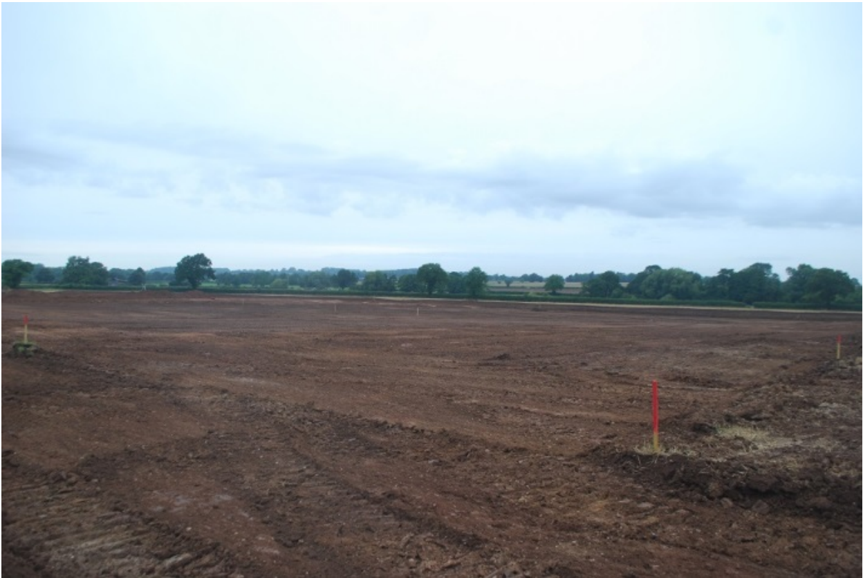
Plate 9, general view south-west of area stripped of topsoil, no scales
