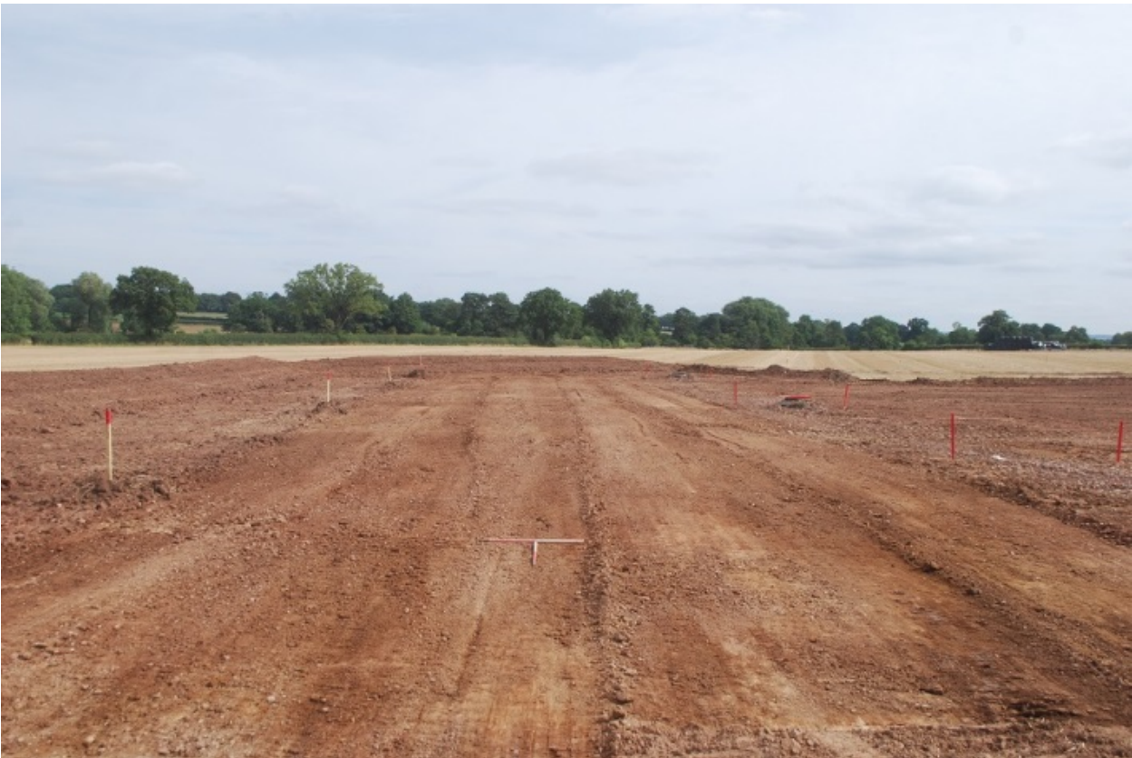
Plate 8, general view east of area stripped of topsoil, 2x 1m scales
