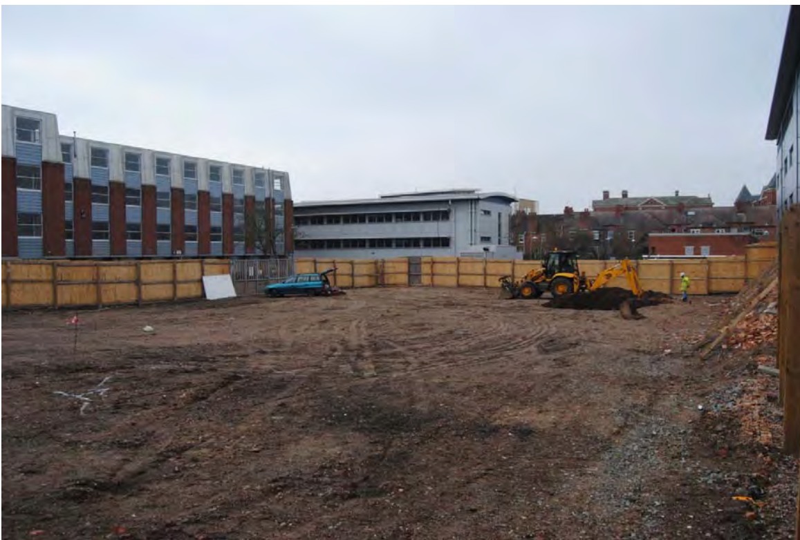
Plate 2 The site from the north-east after demolition of garage complex
