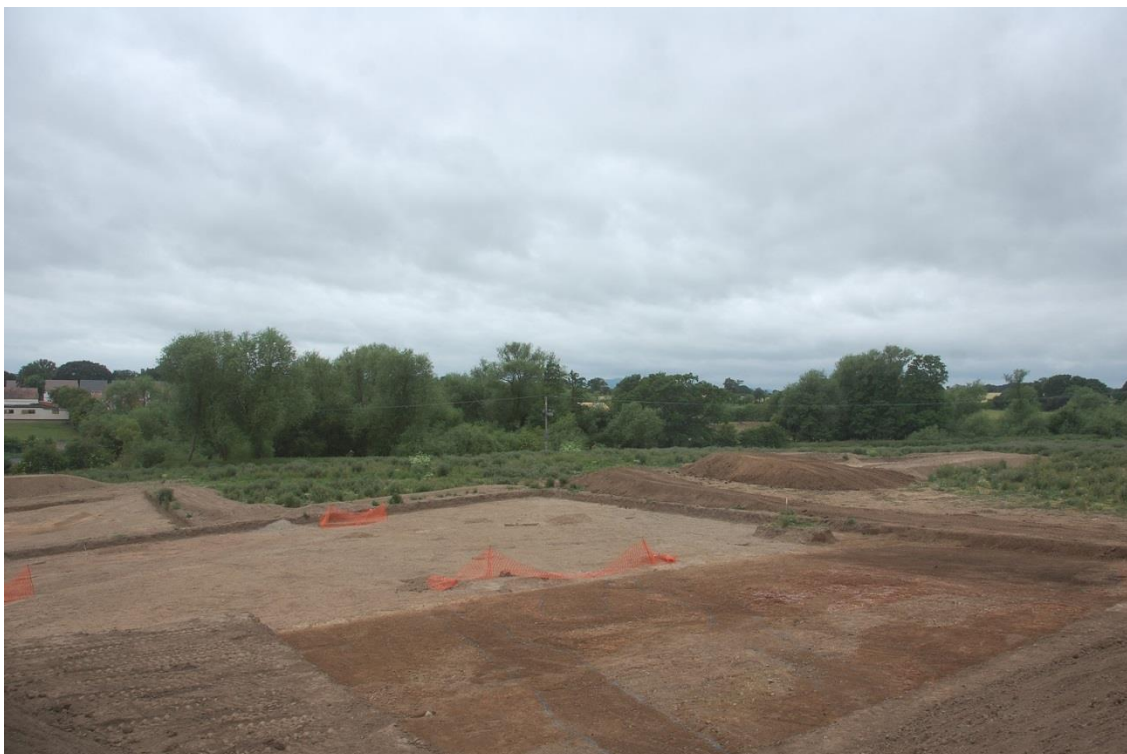
Plate 1: The site during excavation, facing south-west (Area 2 in the foreground)
