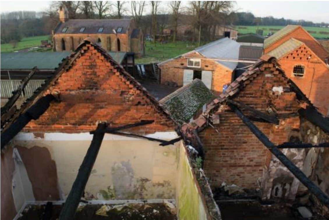
Plate 37 Phases 5 and 5 gables, looking north
