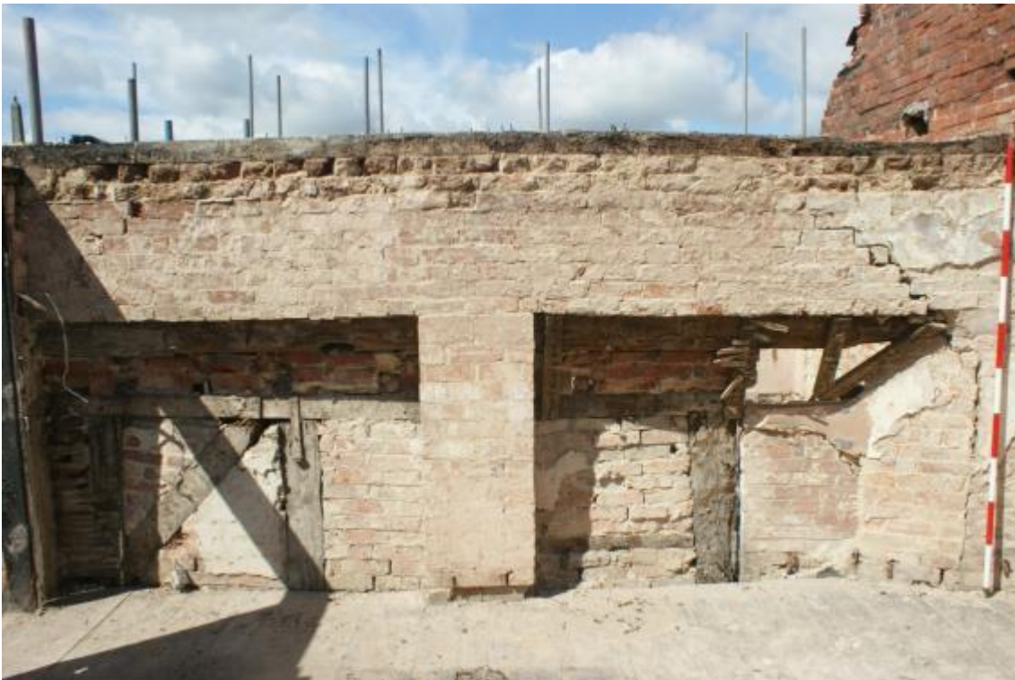
Plate 19 Phase 2 wall frame, first floor looking west
