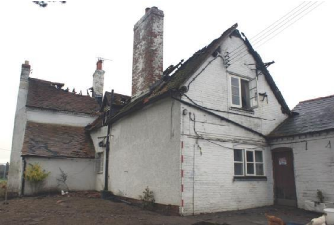
Plate 5 The farmhouse, looking north-west
