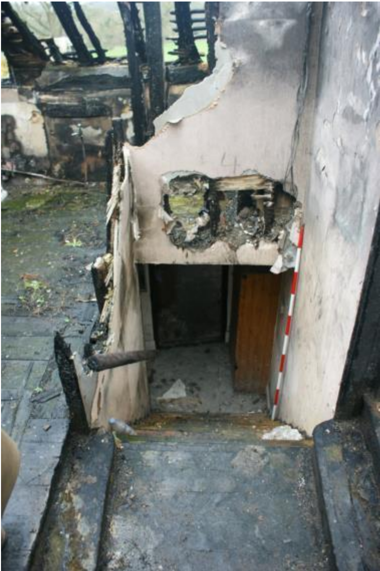
Plate 51 Phase 4 central staircase, looking south
