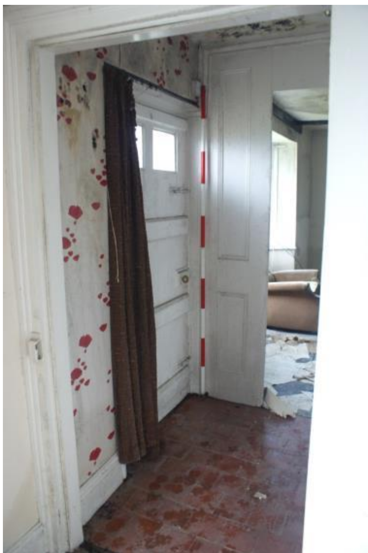
Plate 38 Phase 4 baffle entrance, looking north
