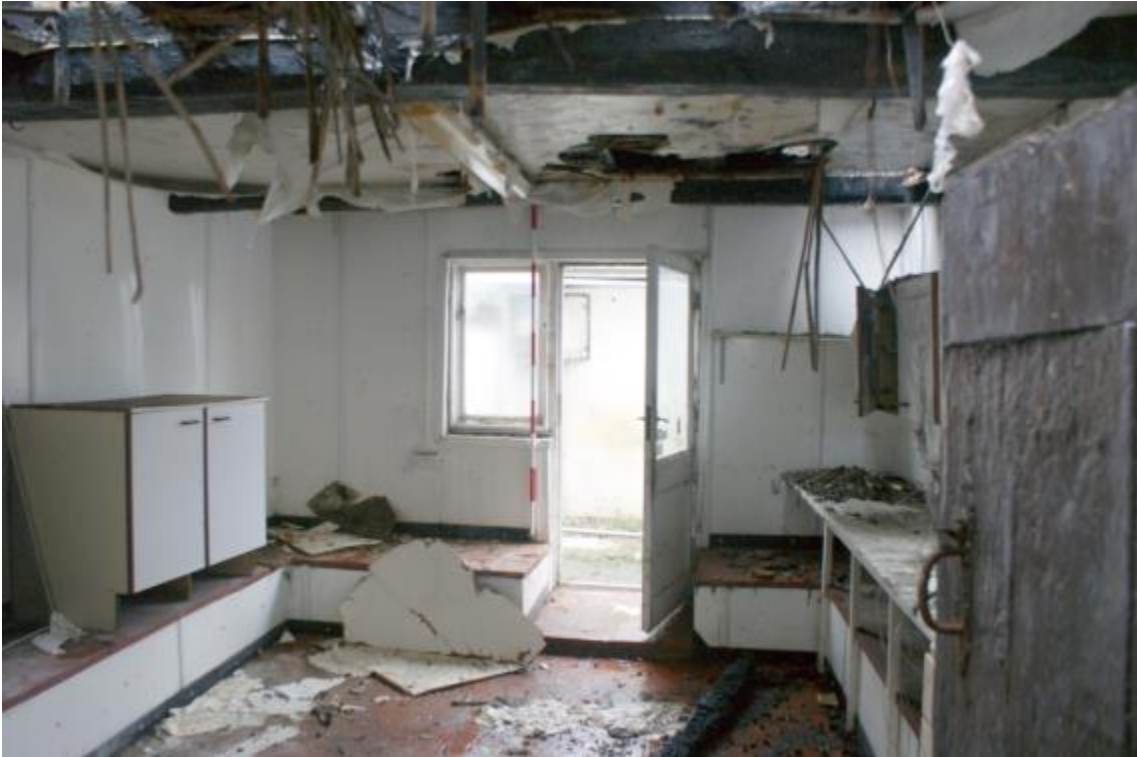
Plate 60 Phase 5 buttery, looking north
