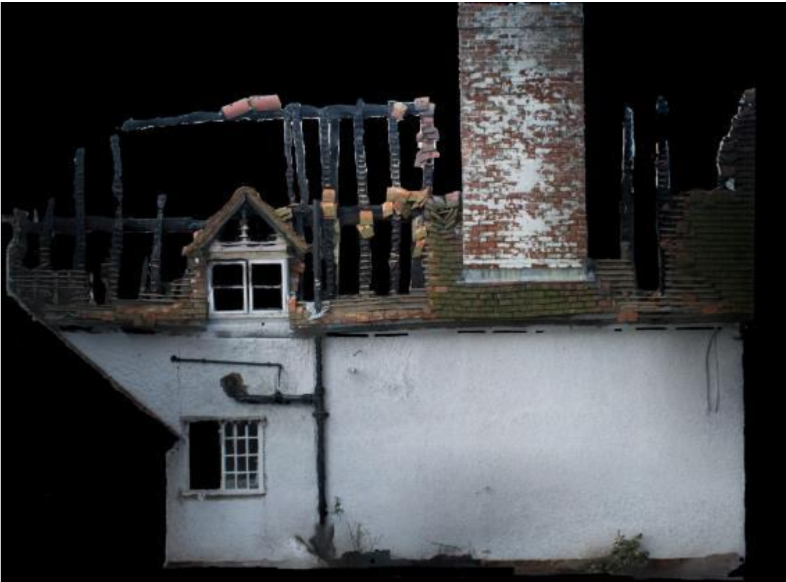
Plate 11 Rectified photograph of Phase 1 and 3 roof structures, looking north
