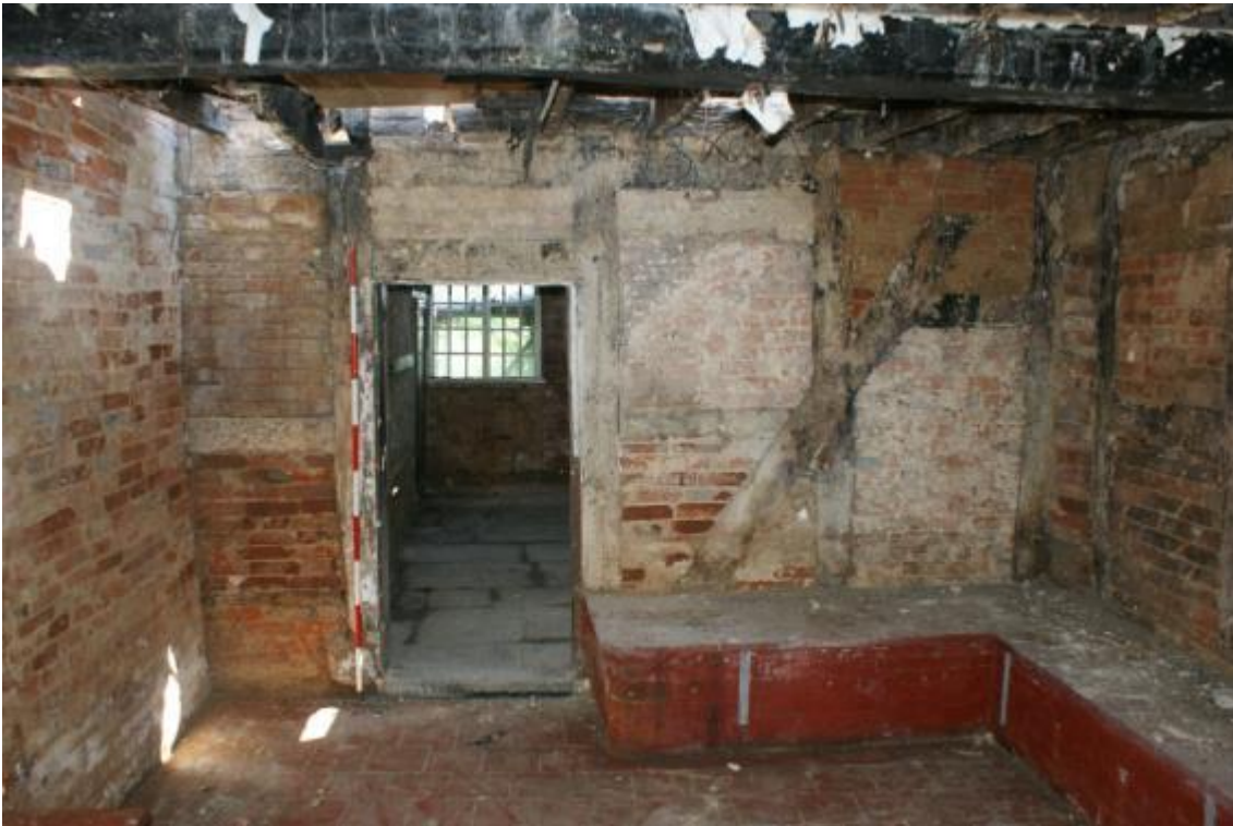
Plate 7 Phase 1 Wall frame visible at ground floor level, looking south
