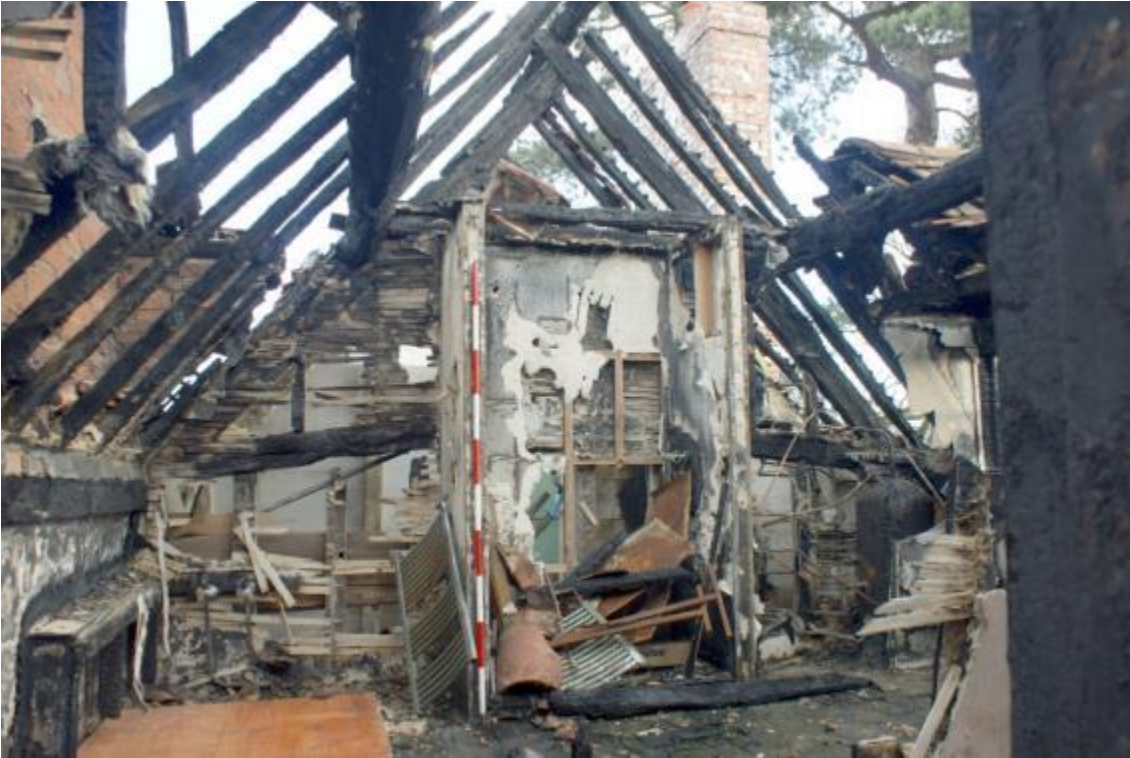
Plate 52 Phase 4 room above former hall, looking east
