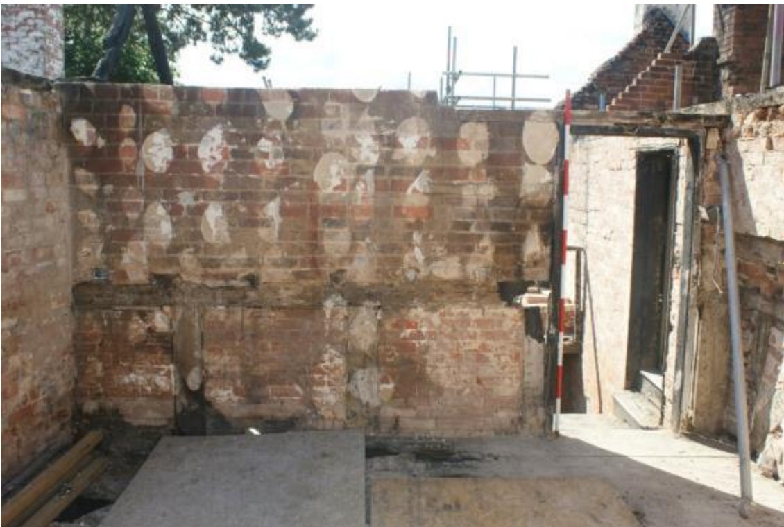
Plate 6 Phase 1 Wall frame with common rafters ends visible above the wall plate, looking south
