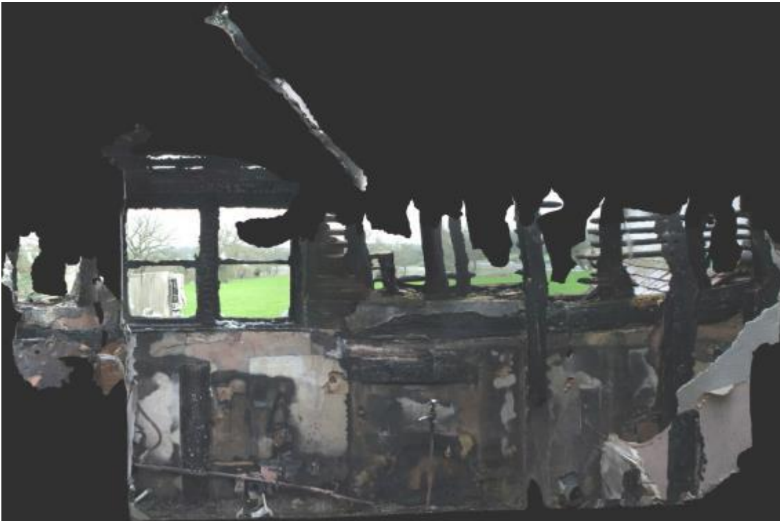
Plate 14 Rectified photograph of Phase 1 wall framing, looking south
