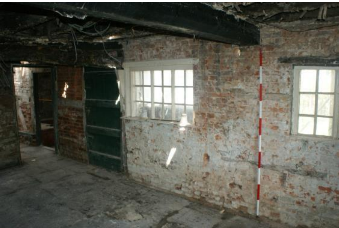
Plate 30 Phase 3 window arches above the later insertions, looking north-west
