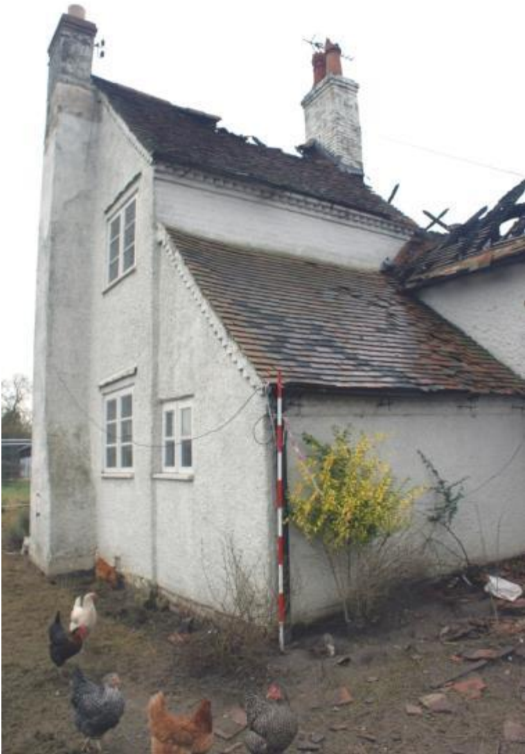
Plate 58 Phase 4, looking north-west
