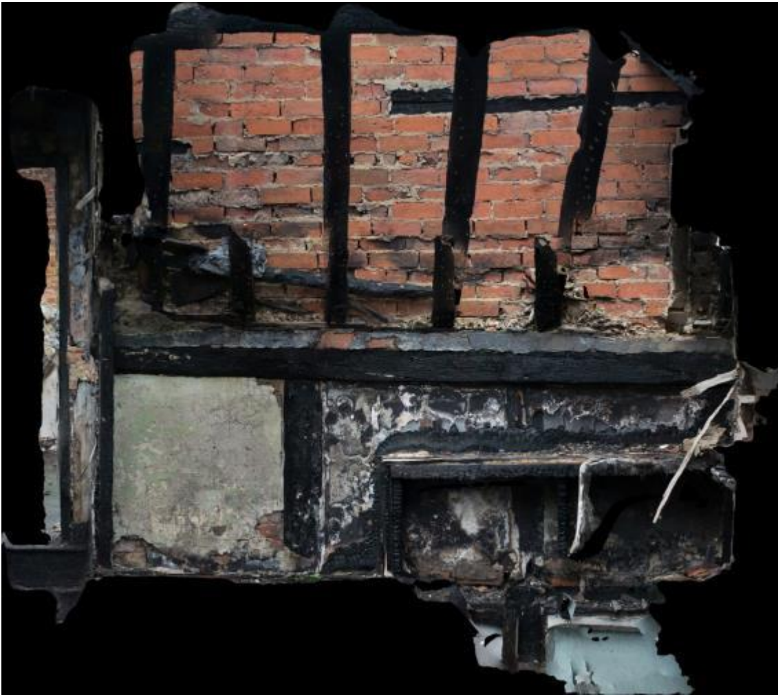
Plate 13 Rectified photograph of Phase 1 wall framing, looking north
