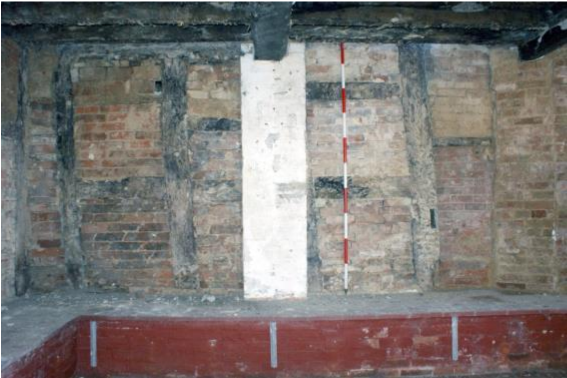
Plate 20 Phase 2 wall frame, ground floor looking west
