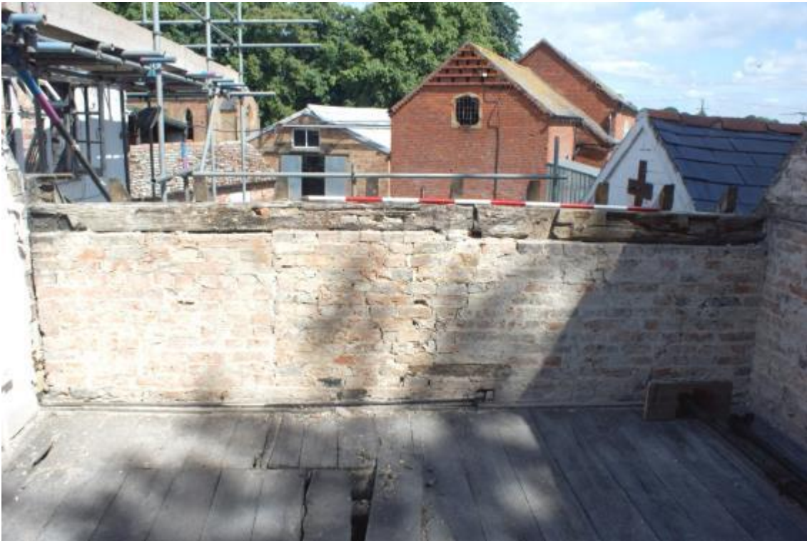
Plate 31 Blocked Phase 3 window and reused wall plate, looking north
