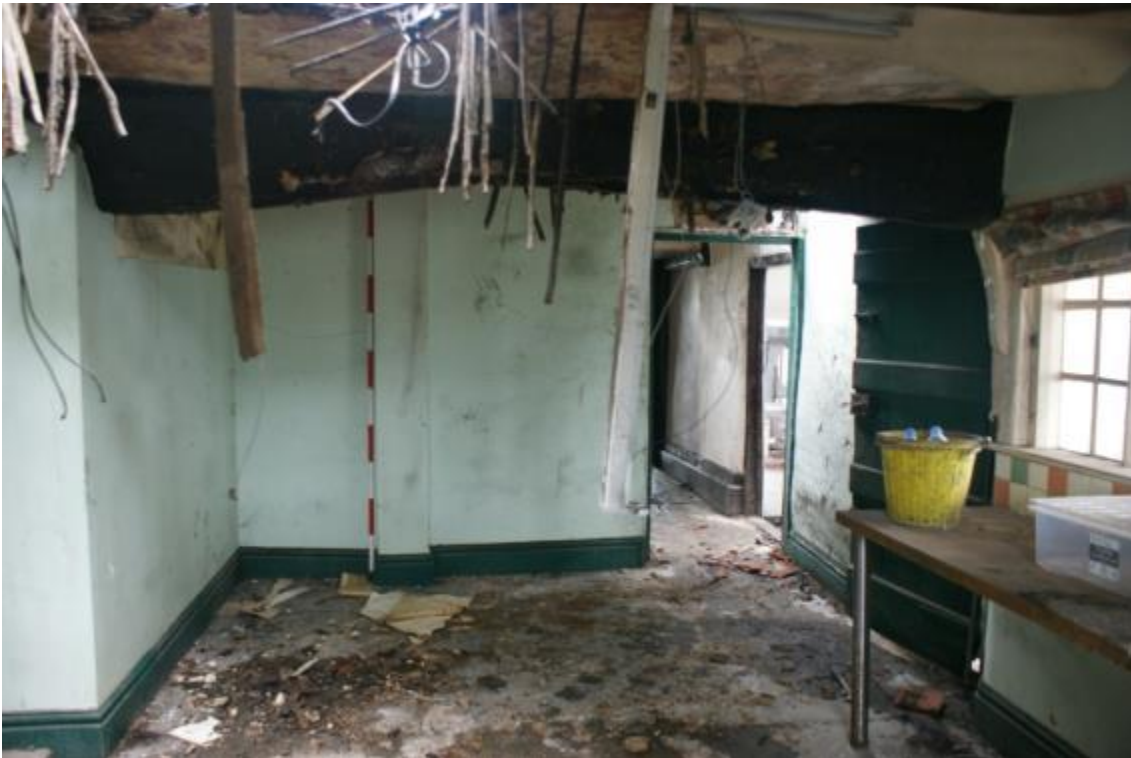
Plate 33 Phase 2 and later kitchen, looking west
