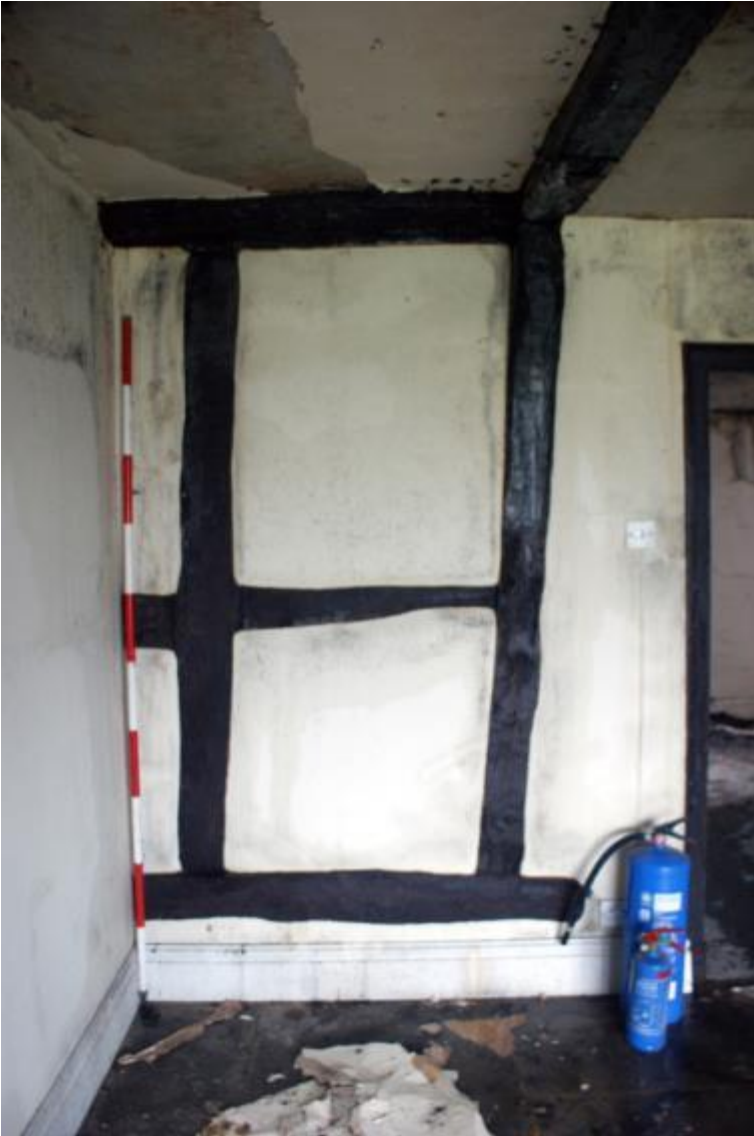
Plate 22 Phase 2 wall and cross frame post, looking east
