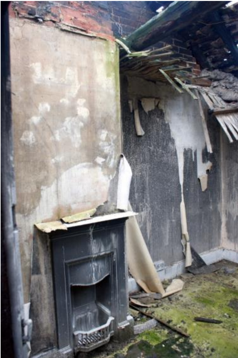
Plate 56 Phase 4 bed room, looking south-west
