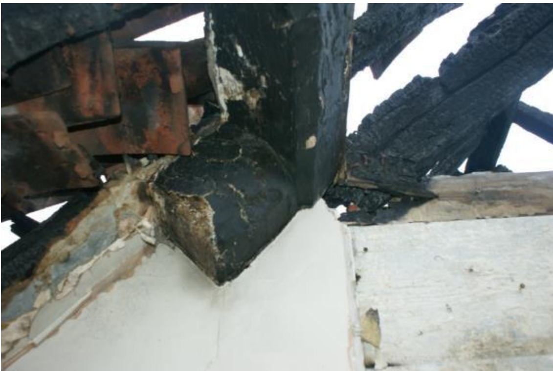
Plate 15 Phase 1 chamfered purlin end, looking west
