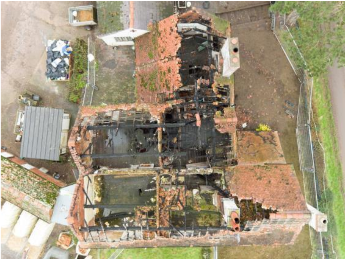
Plate 3 The farmhouse roof, vertical
