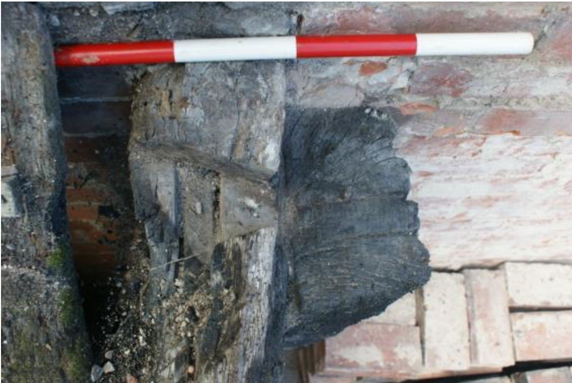
Plate 18 Detail of the Phase 1 jowl post head showing the dovetail joint and sawn off tenon on the eastern side of the frame, looking west, scale 0.40m
