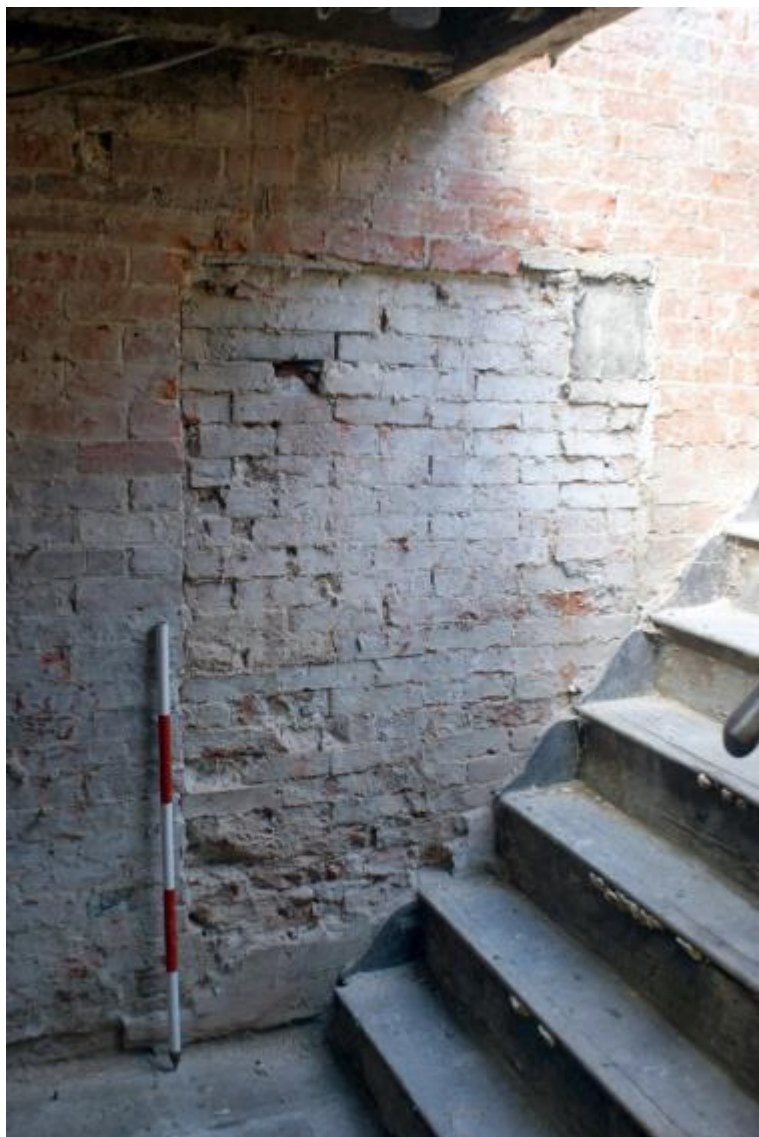
Plate 25 Building breaks showing the possible Phase 2 chimney, looking west
