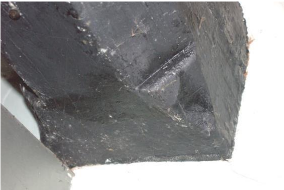
Plate 34 Chamfer on Phase 3 beam, looking north
