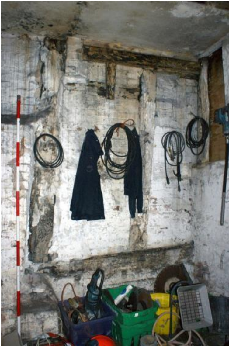
Plate 21 Phase 2 wall and cross frame post, looking east
