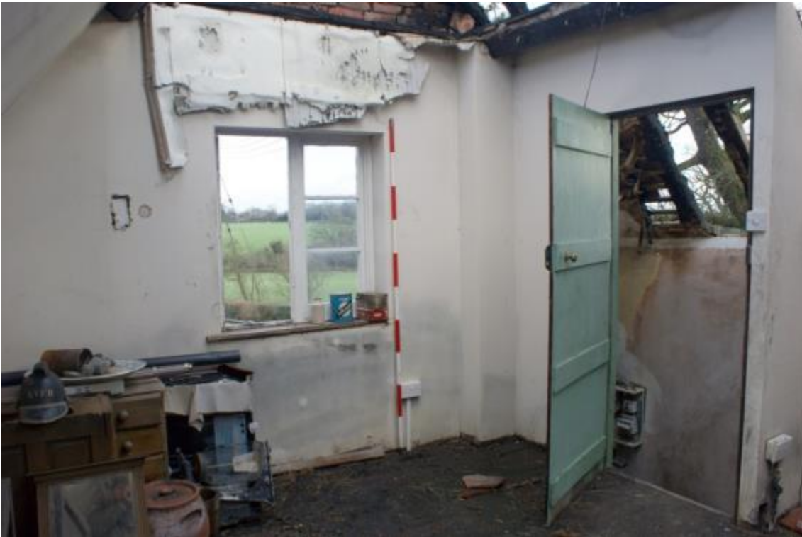
Plate 27 Phase 2 extension, looking south east
