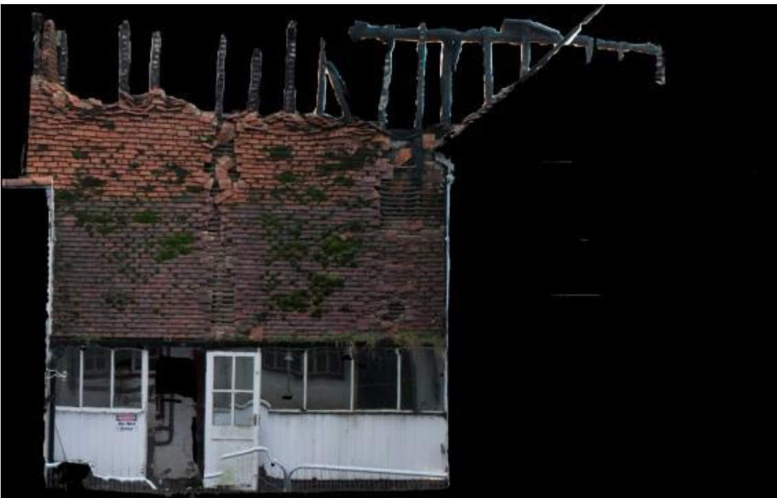
Plate 12 Rectified photograph of Phase 1 and 3 roof structures, looking south
