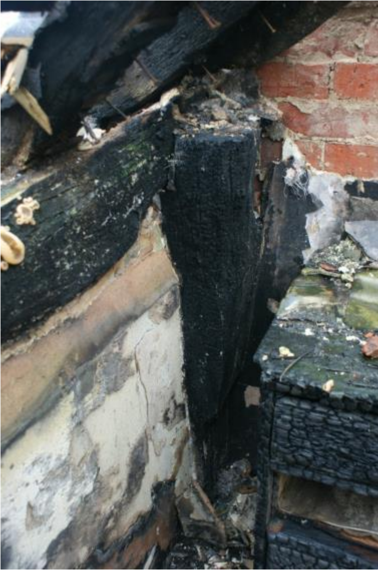
Plate 17 Phase 1 jowl post, looking south-west
