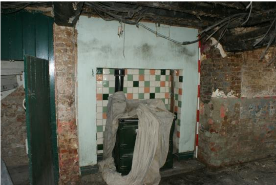
Plate 32 Probable Phase 3 fireplace, looking south
