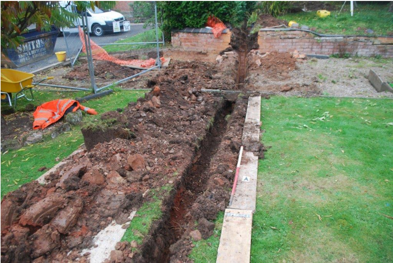
Plate 7 Demolition deposit 109 to the north of wall 108 and trench across driveway
