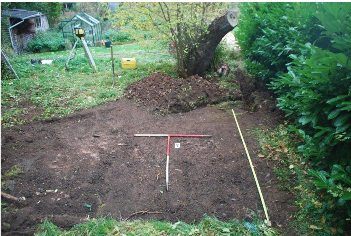
Plate 2 The excavation for the foundation pad, looking south
