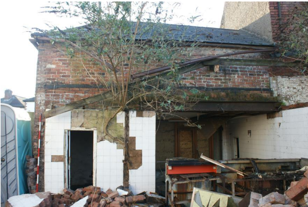
Plate 40 Phase 3 Number 23, looking south-east
