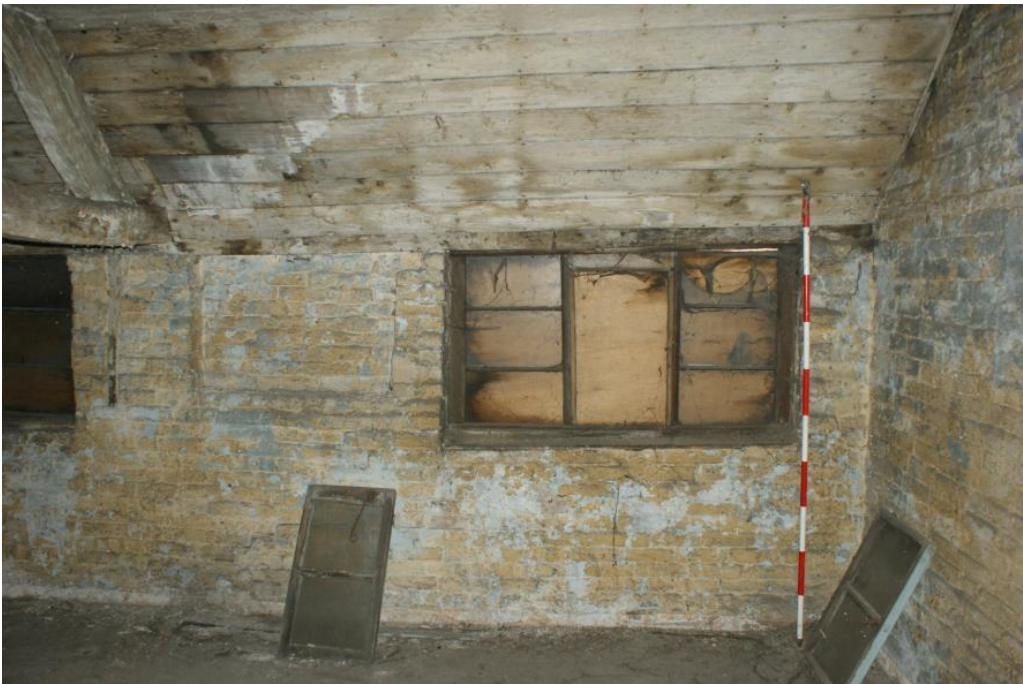
Plate 14 Phase 1 second floor room, looking south-east
