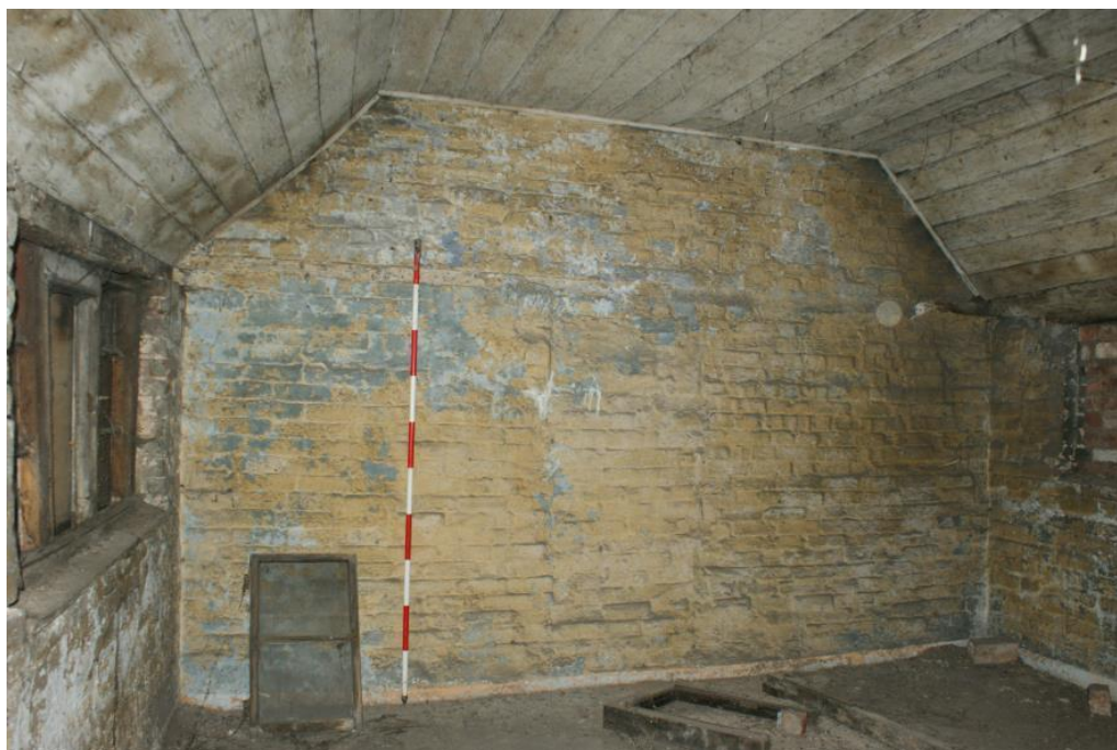
Plate 21 Blocked doorway in the Phase 1 gable end, looking south-west
