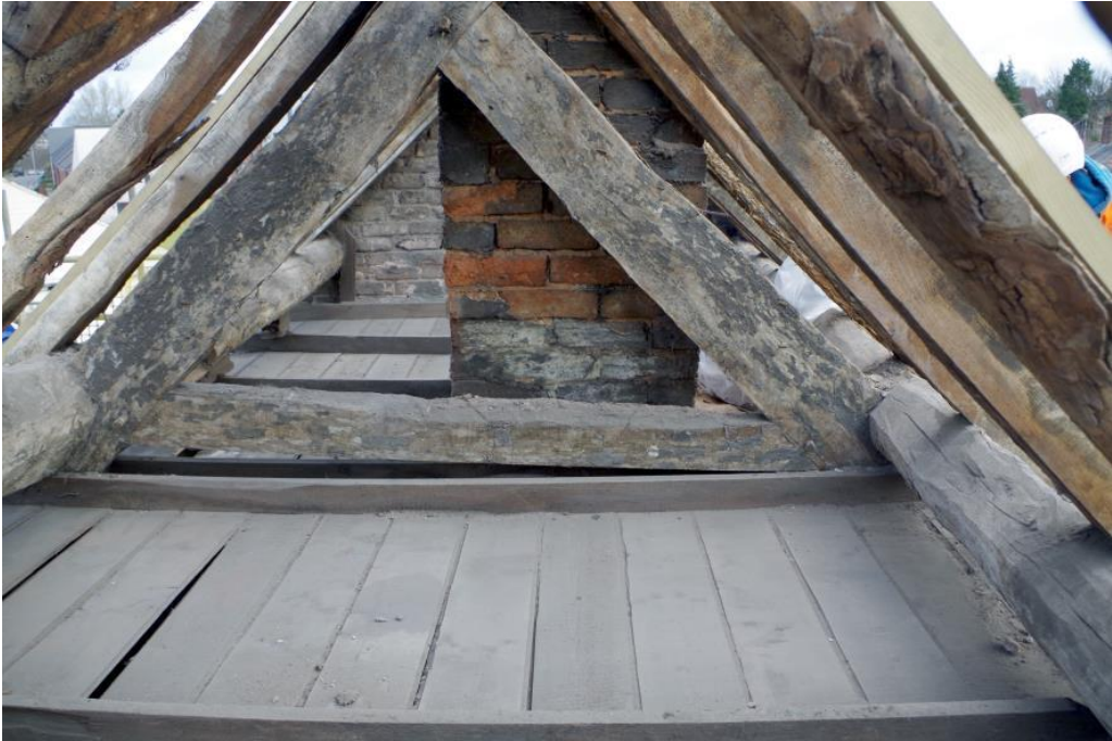
Plate 15 Phase 1 roof structure, looking north-east
