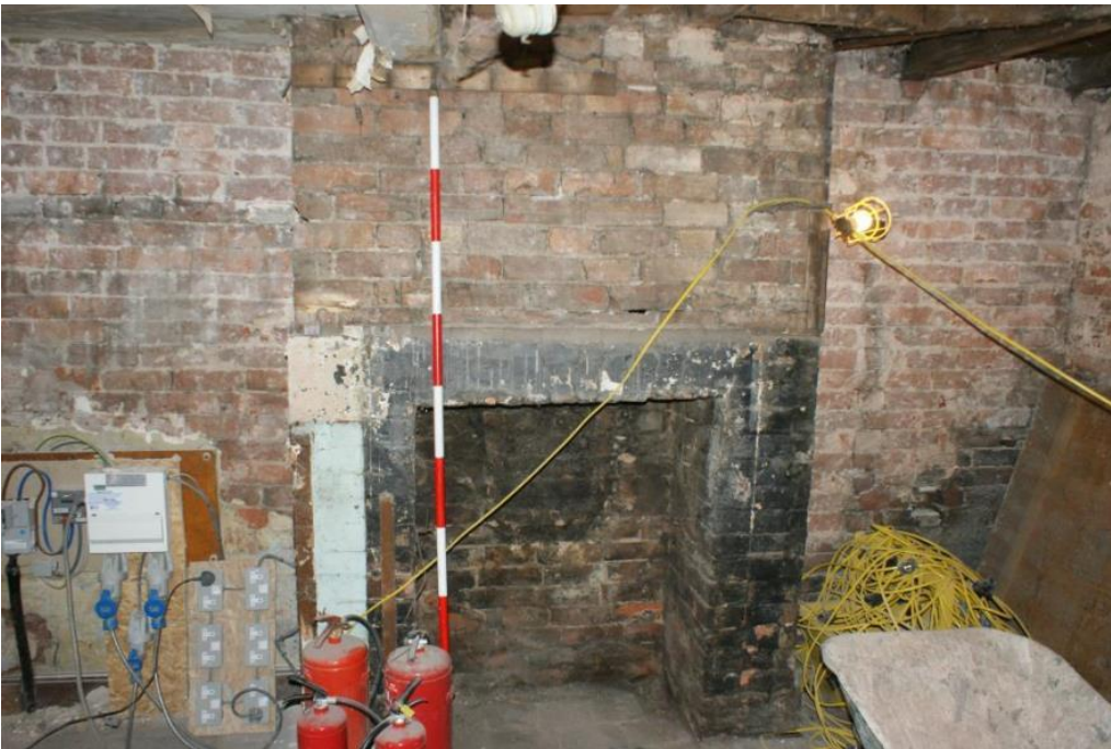
Plate 30 Phase 3, Number 21 ground floor, looking south-west
