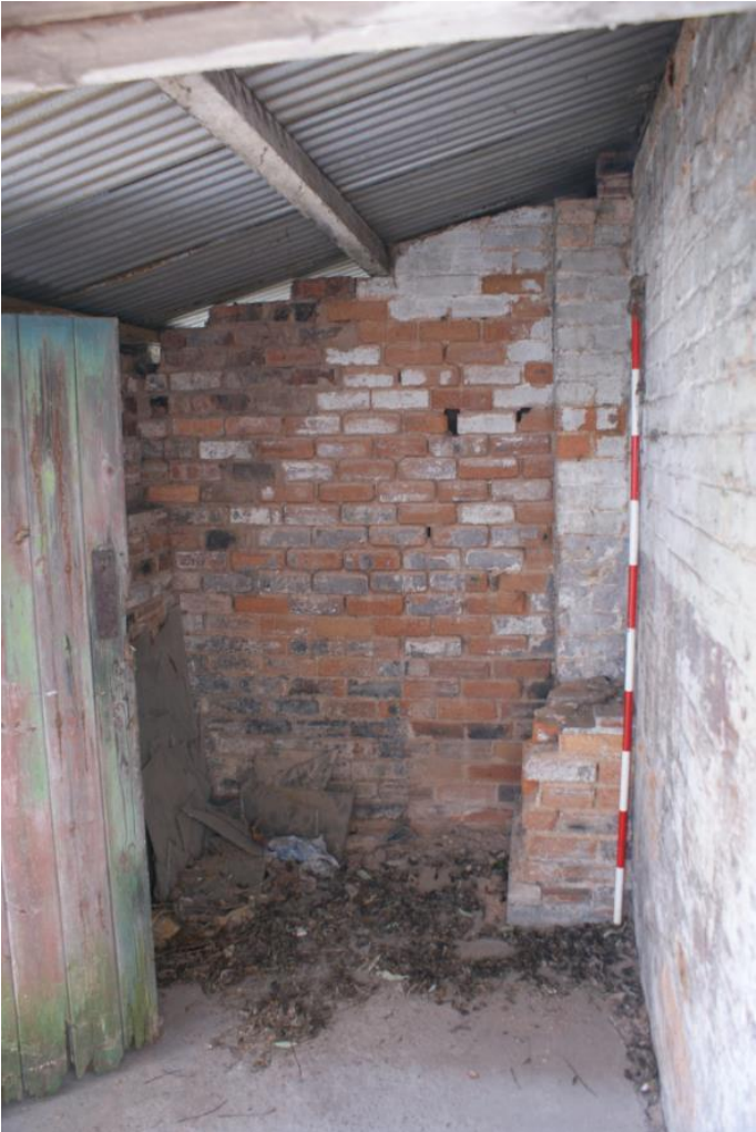
Plate 55 Phase 5 kitchens or washrooms, looking east
