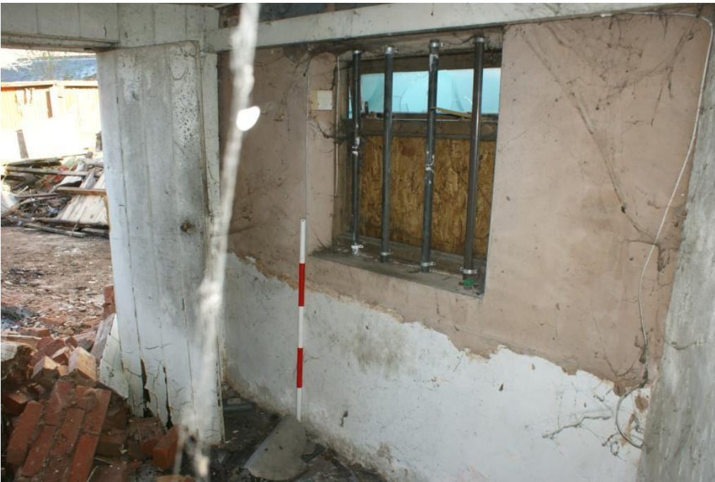
Plate 41 Phase 3 Number 23 ground floor, looking north
