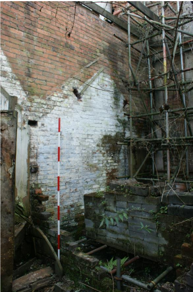
Plate 49 Phase 4 rooms, looking south
