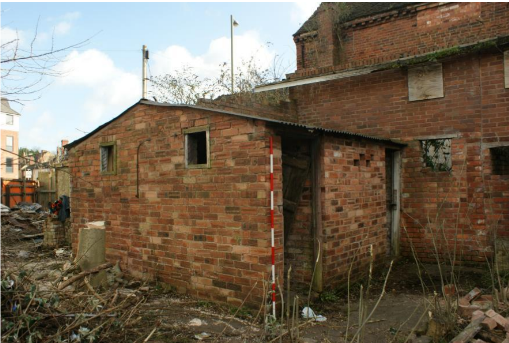
Plate 53 Phase 5 kitchens or washrooms, looking east
