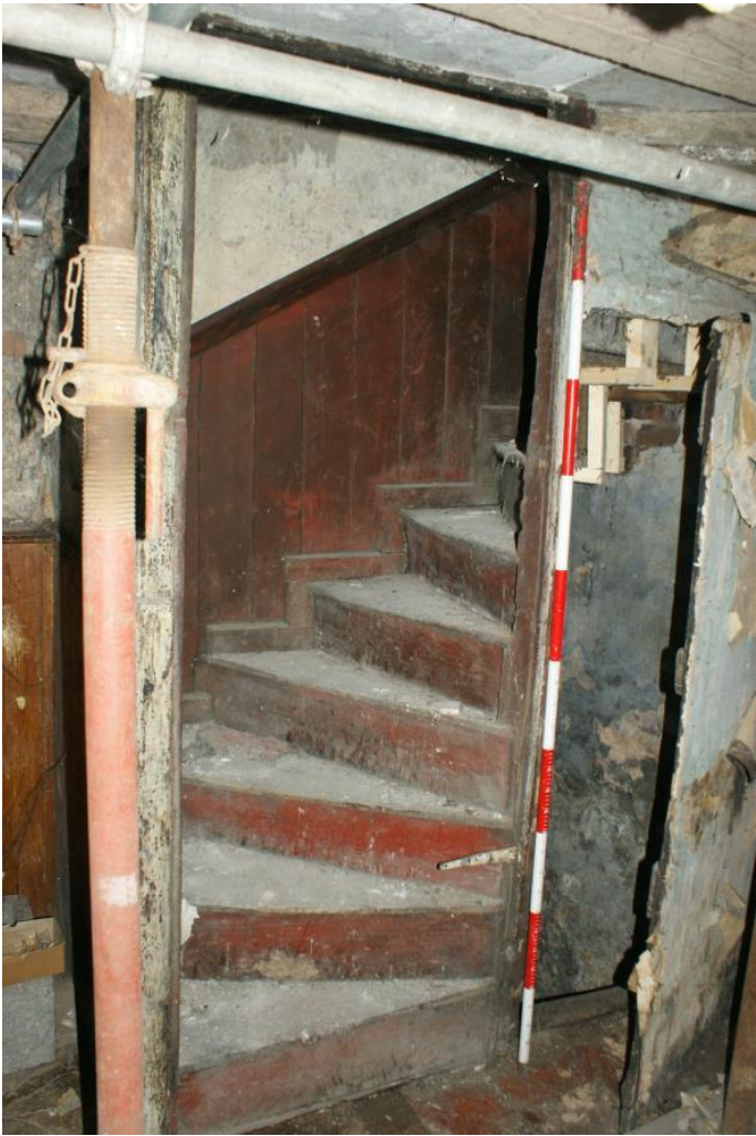
Plate 7 Phase 1 staircase, looking north
