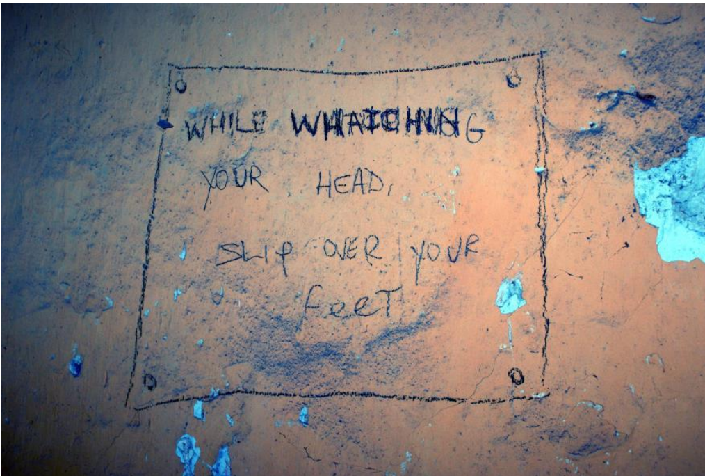
Plate 65 Phase 6 sketches in number 20 in the stair well between the first and second floor, looking south
