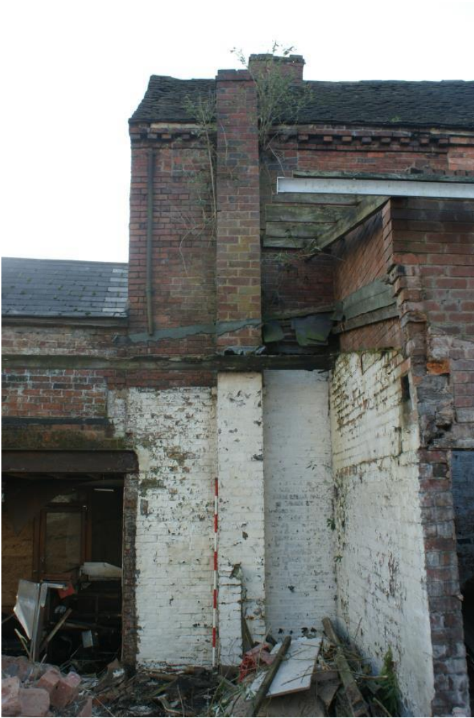
Plate 56 Phase 5 chimney, after demolition of Phase 6 structures, looking south-east
