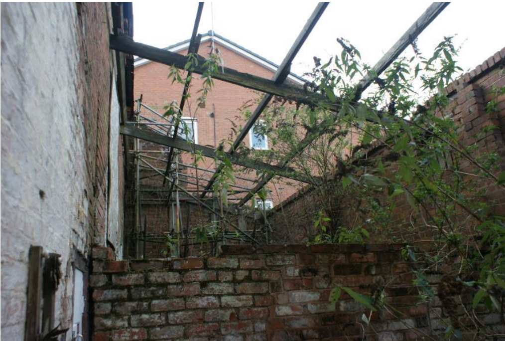
Plate 50 Phase 4 rooms, looking south-west
