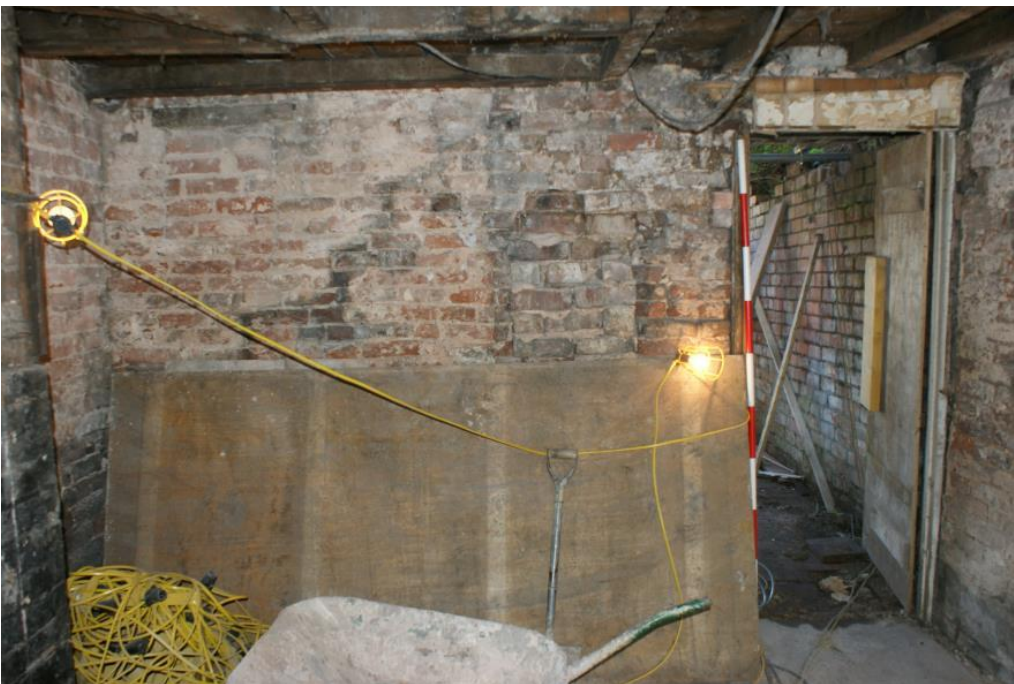
Plate 31 Phase 3, Number 21 ground floor showing evidence of former stairs, looking north-west
