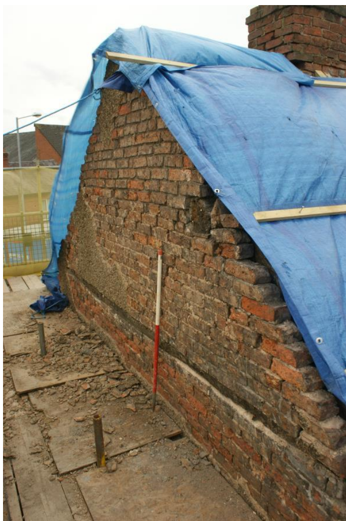
Plate 20 Phase 1 gable end, looking south
