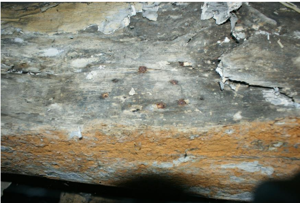
Plate 23 Nails visible in the tie beam of the Phase 1 second floor room, looking north-east
