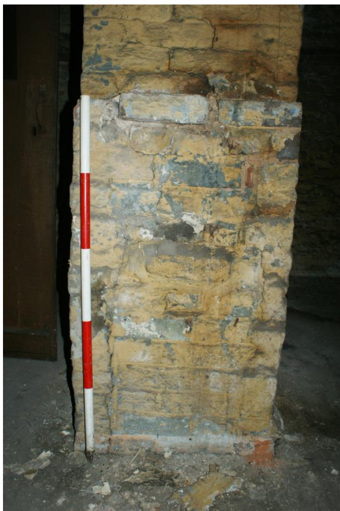
Plate 13 Possible Phase 1 former fireplace, looking north-east
