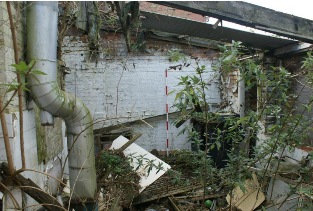
Plate 62 Phase 6 extension to Number 23, looking south-west
