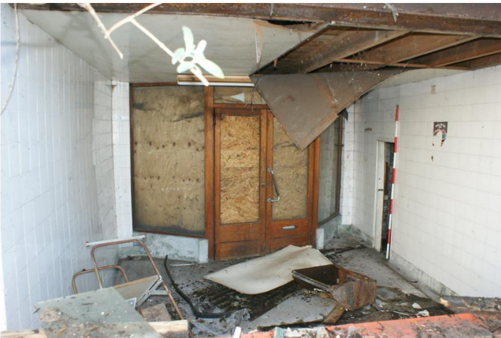
Plate 42 Phase 3 Number 23 ground floor, looking south-east
