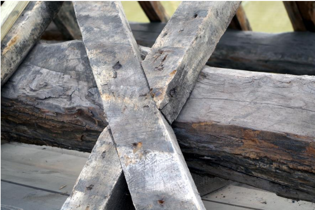
Plate 16 Phase 1 roof structure, looking north-east
