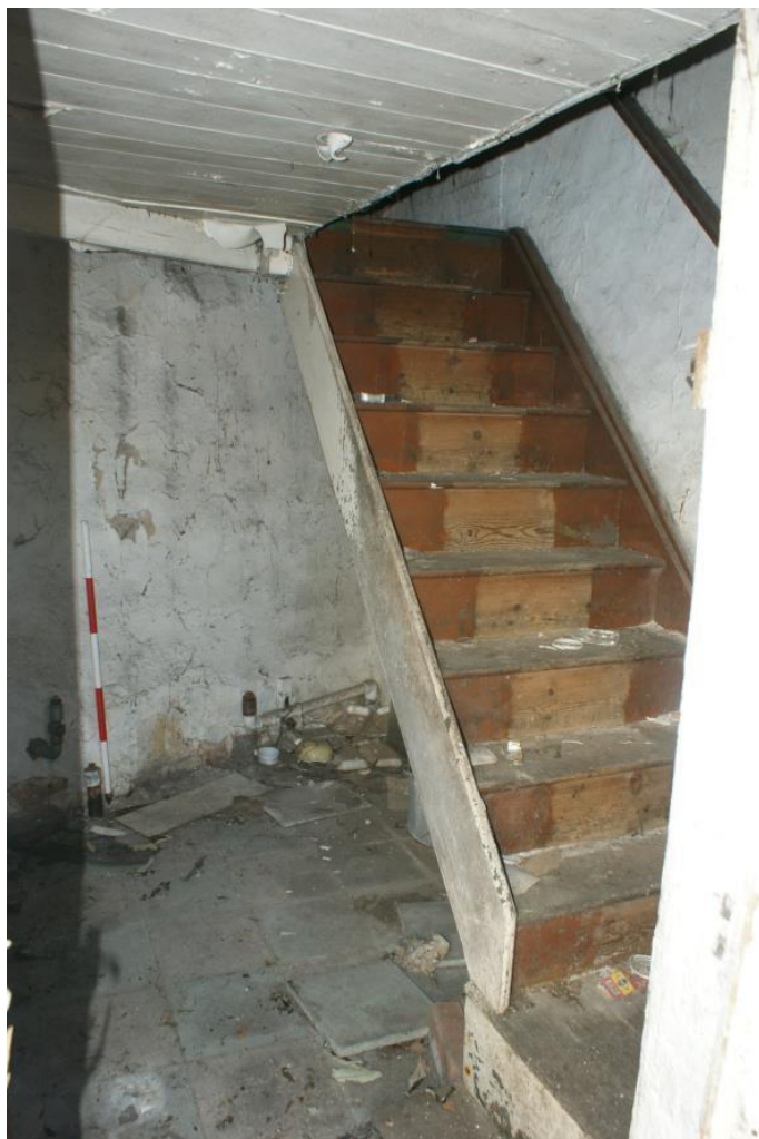
Plate 43 Phase 3 Number 23 ground floor, looking south
