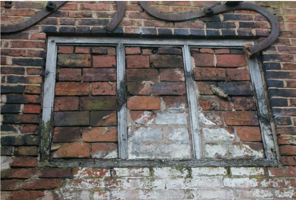
Plate 11 Phase 1 blocked window, looking south-east
