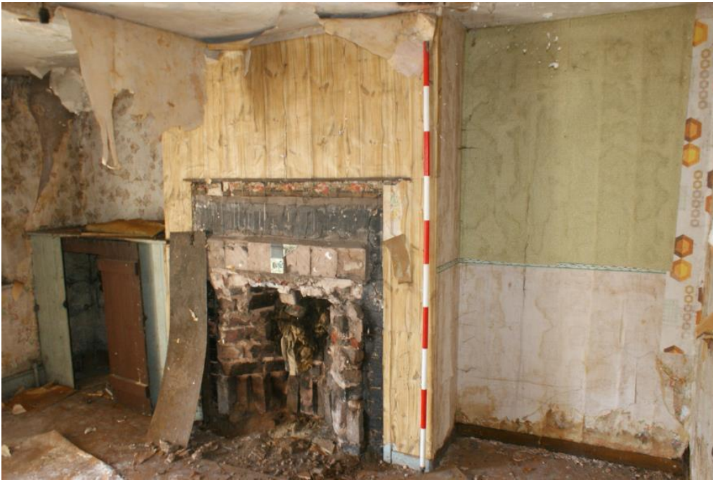
Plate 27 Phase 3, Number 21 ground floor, looking south
