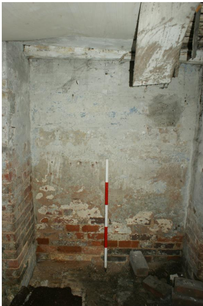
Plate 6 Phase 1 groundfloor storage room, looking north-west
