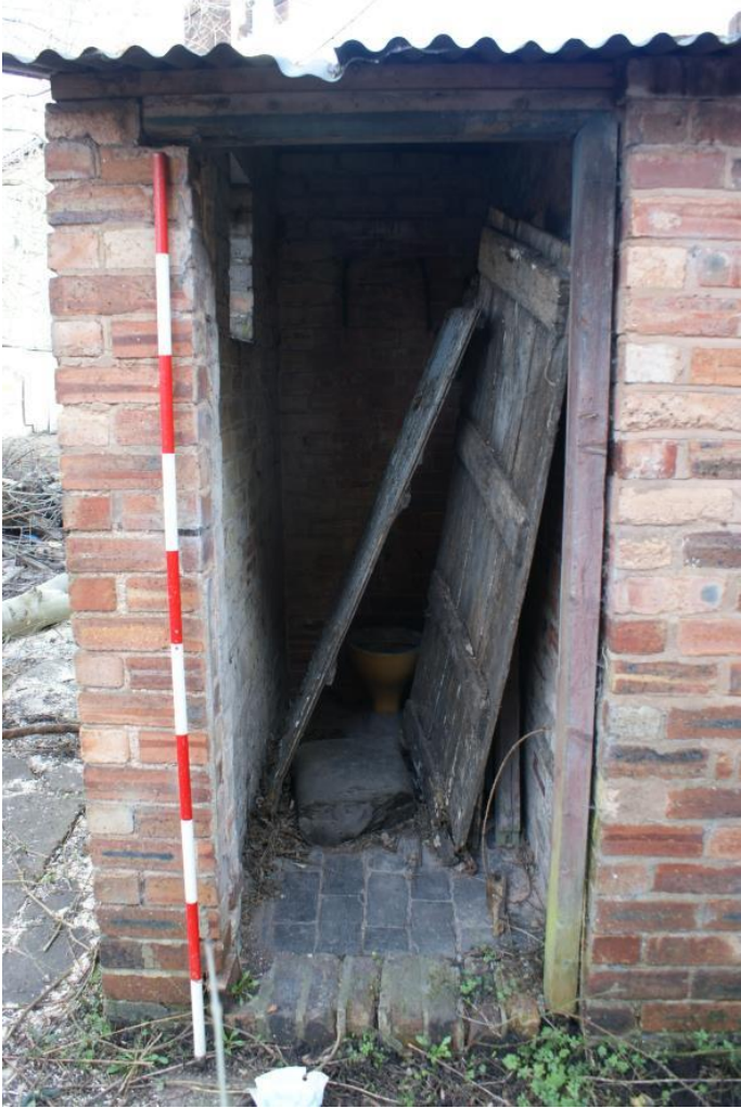
Plate 54 Phase 5 toilet, looking east
