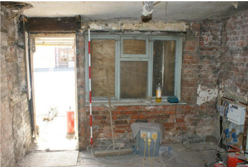
Plate 29 Phase 3, Number 21 ground floor, looking south-east
