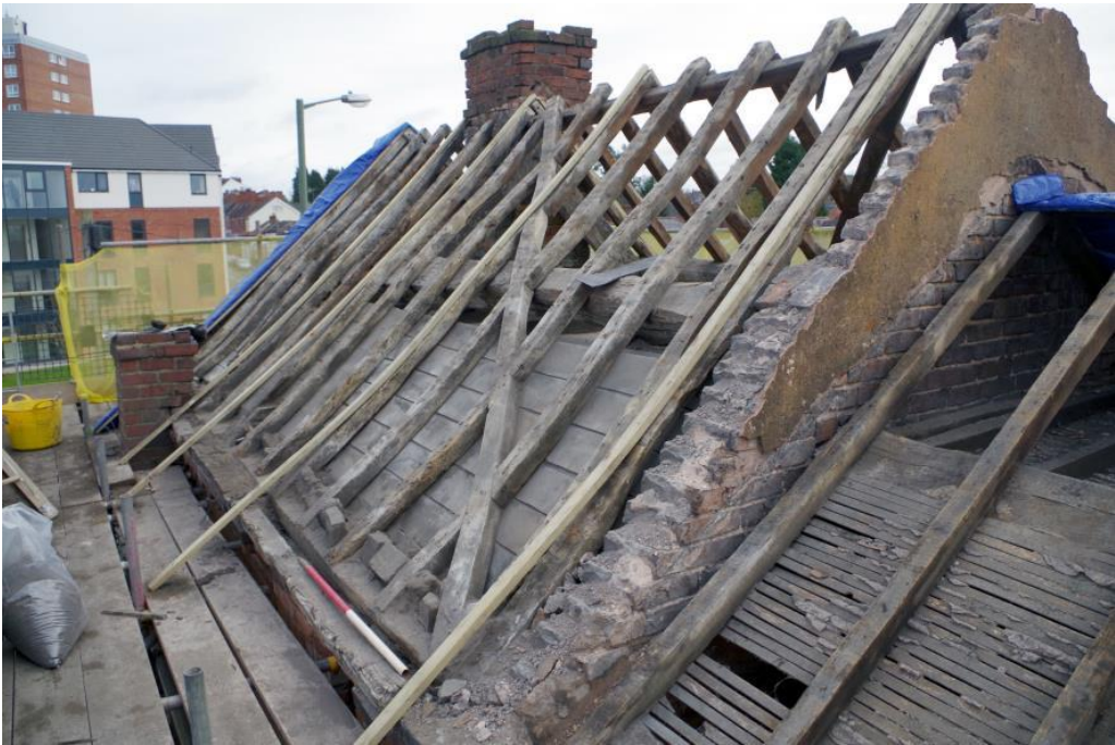
Plate 17 Phase 1 roof structure, looking north-east
