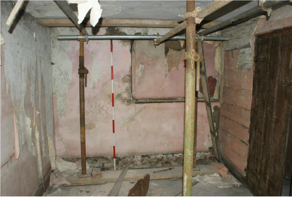
Plate 10 Phase 1 first floor bedroom, looking north-west
