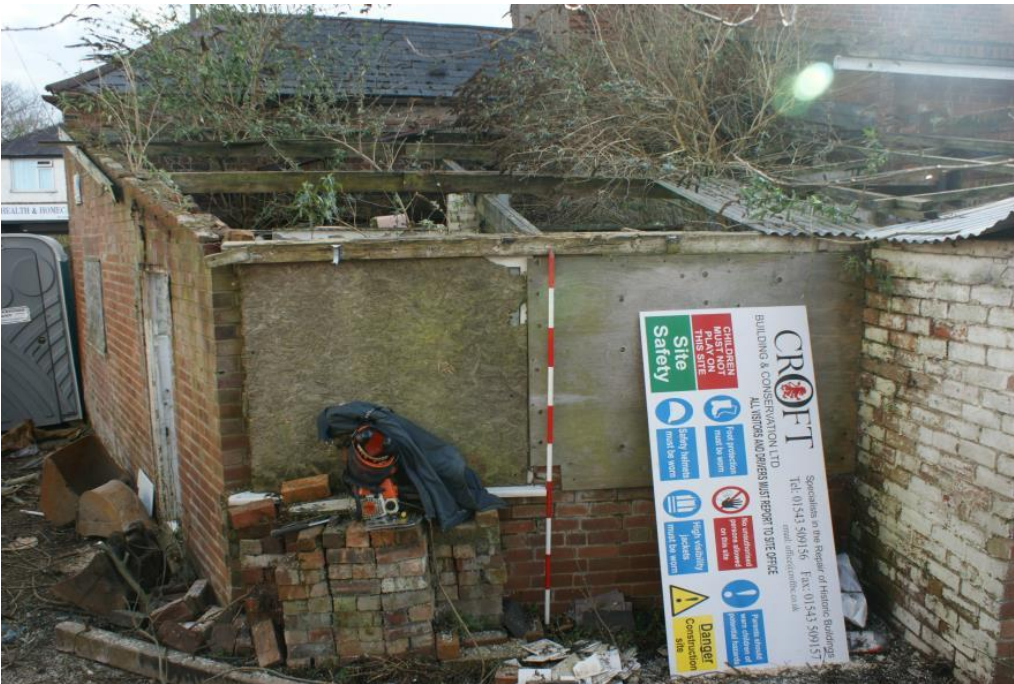
Plate 61 Phase 6 extension to Number 23, looking south-east
