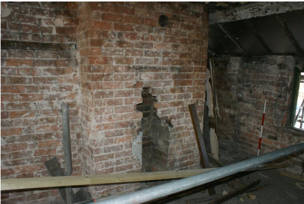
Plate 34 Phase 3, Number 21 second floor, looking south-west
