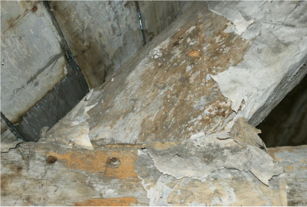
Plate 24 Pegging visible in the principle rafter of the Phase 1 second floor room, looking south-west
