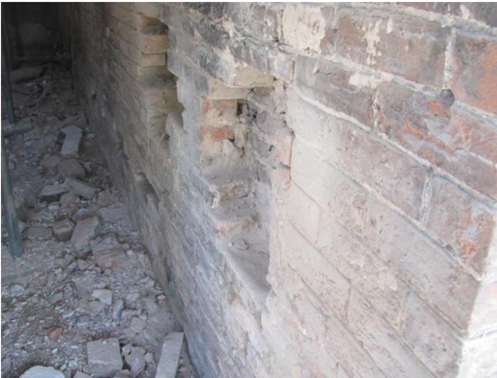
Plate 22 Bricks visible in the gable end of Number 20, suggesting the presence of an earlier structure, looking north
