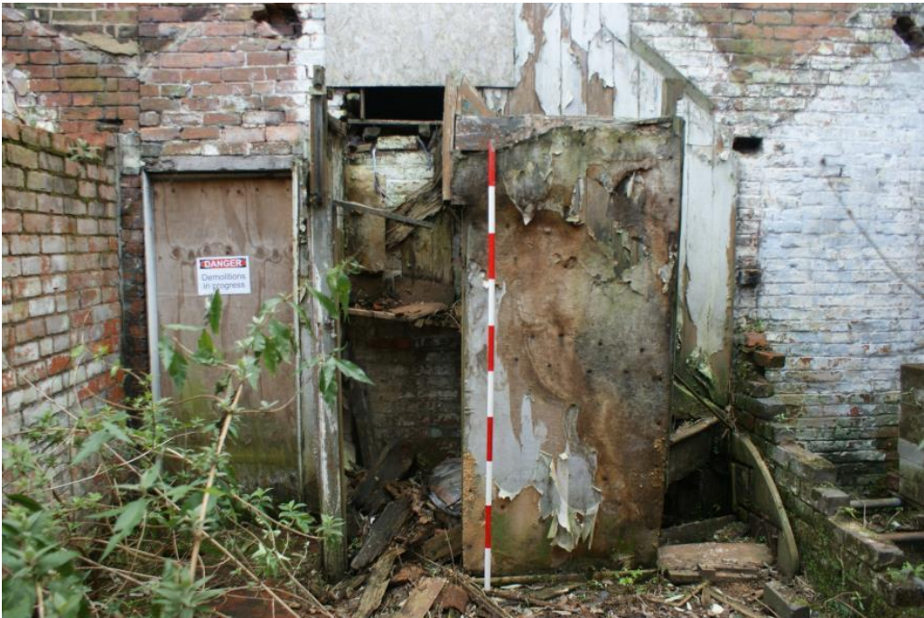
Plate 48 Phase 4 rooms, looking south -east
