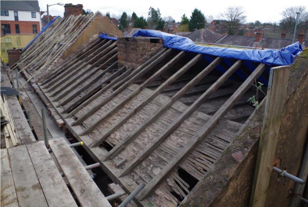
Plate 35 Phase 3 numbers 20 and 21 roof structure, looking east
