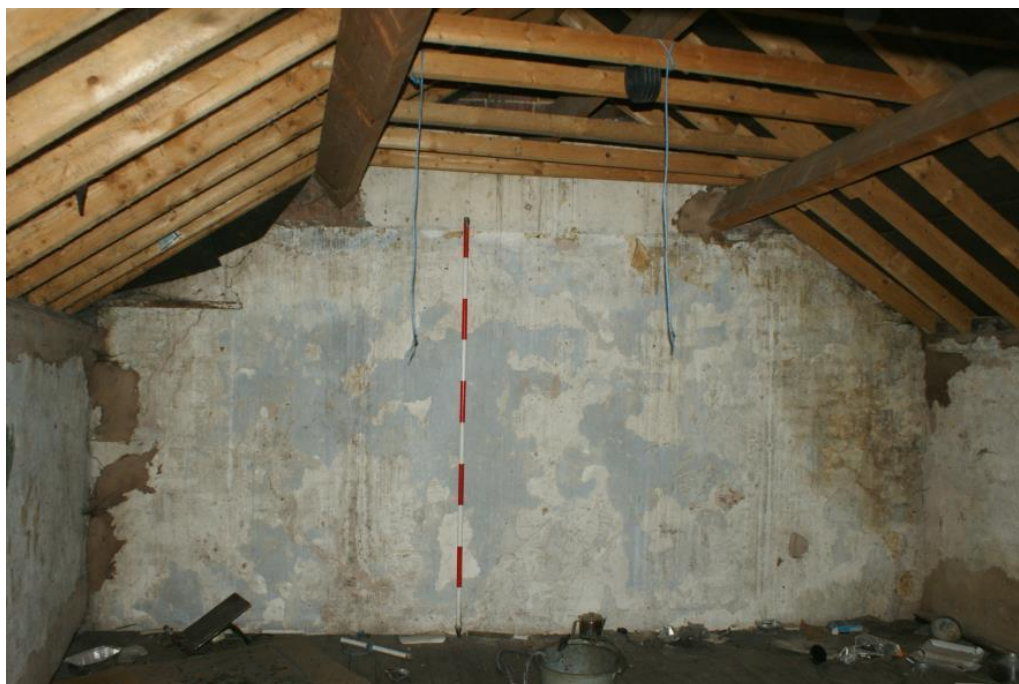
Plate 44 Phase 3 Number 23 first floor, looking south-west
