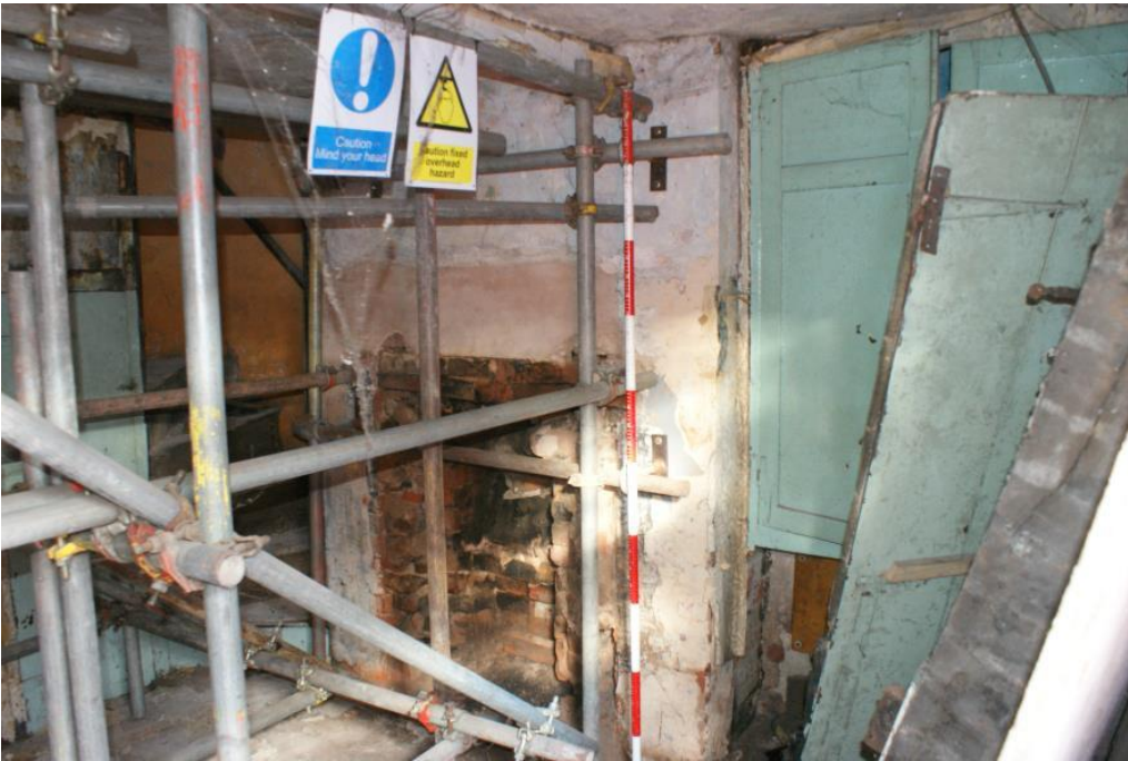
Plate 28 Phase 3, Number 20 ground floor, looking north
