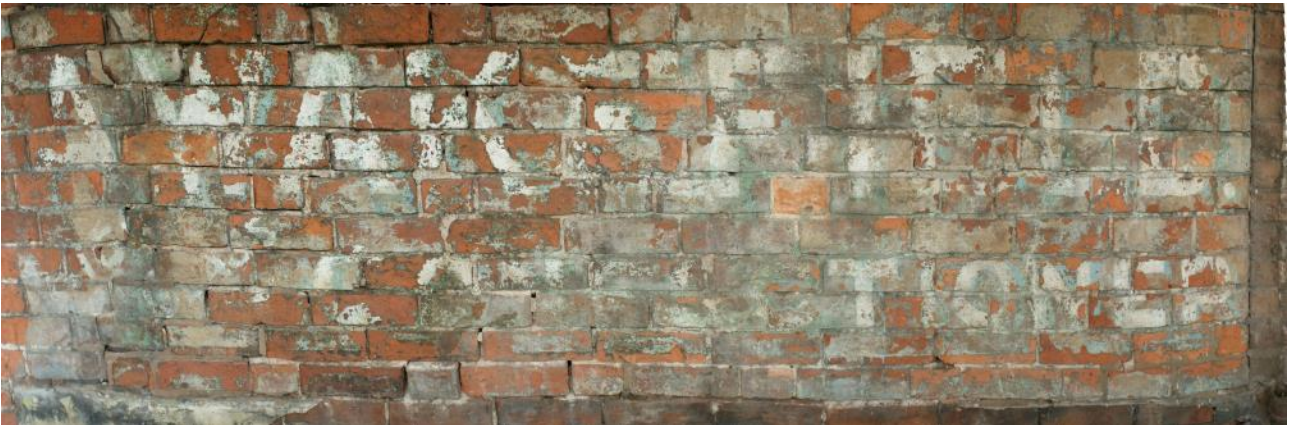
Plate 58 Phase 6 painted sign on Number 21 first floor frontage, looking north-west
