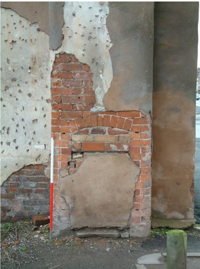
Plate 36 (Robson-Glyde 2004) Phase 3 ground floor fireplace place of the former Cock Inn, Number 20 gable, looking north-east
