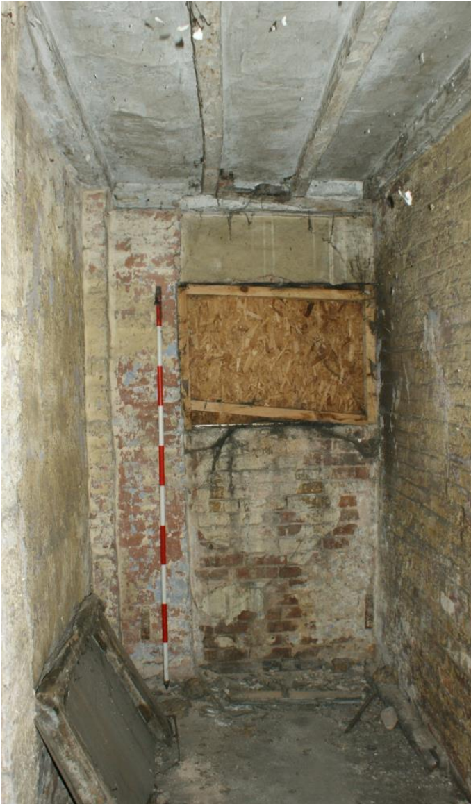
Plate 9 Phase 1 first floor storage room, looking south-east
