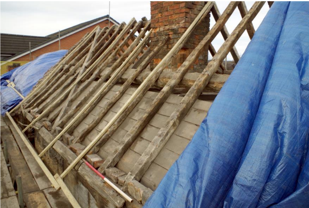
Plate 18 Phase 1 roof structure, looking south-west
