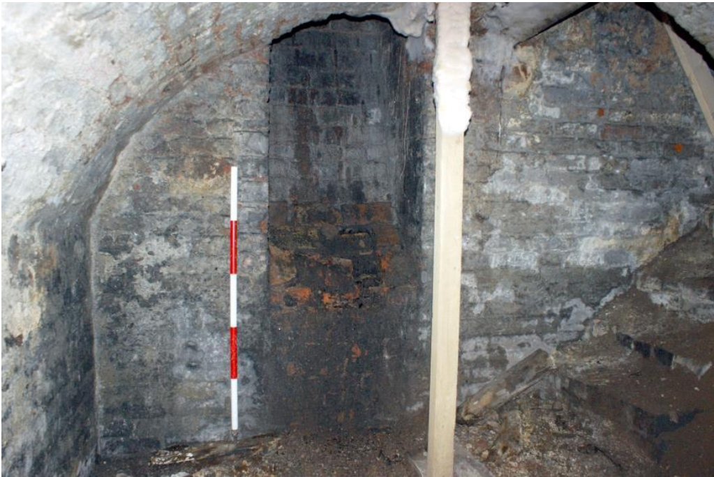
Plate 4 Phase 1 cellar, looking north-west
