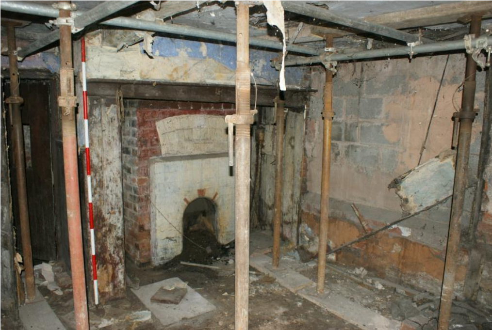
Plate 2 Phase 1 living room, looking east
