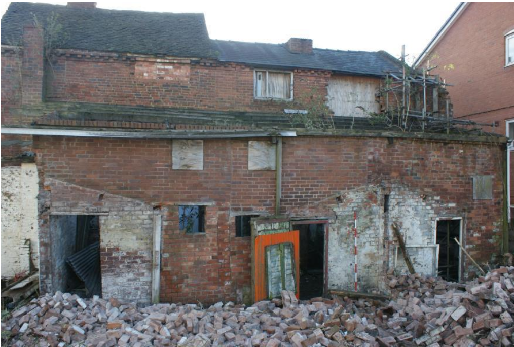
Plate 46 Phase 4 structures, after demolition of Phase 5 structures, looking south-east
