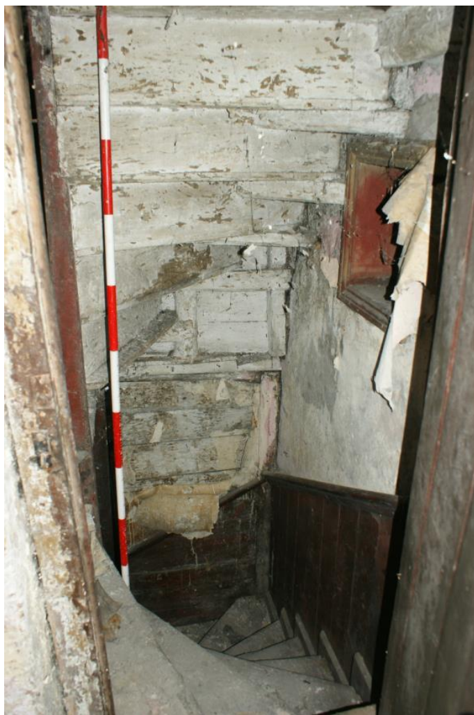
Plate 8 Phase 1 Staircase from the first floor, looking west
