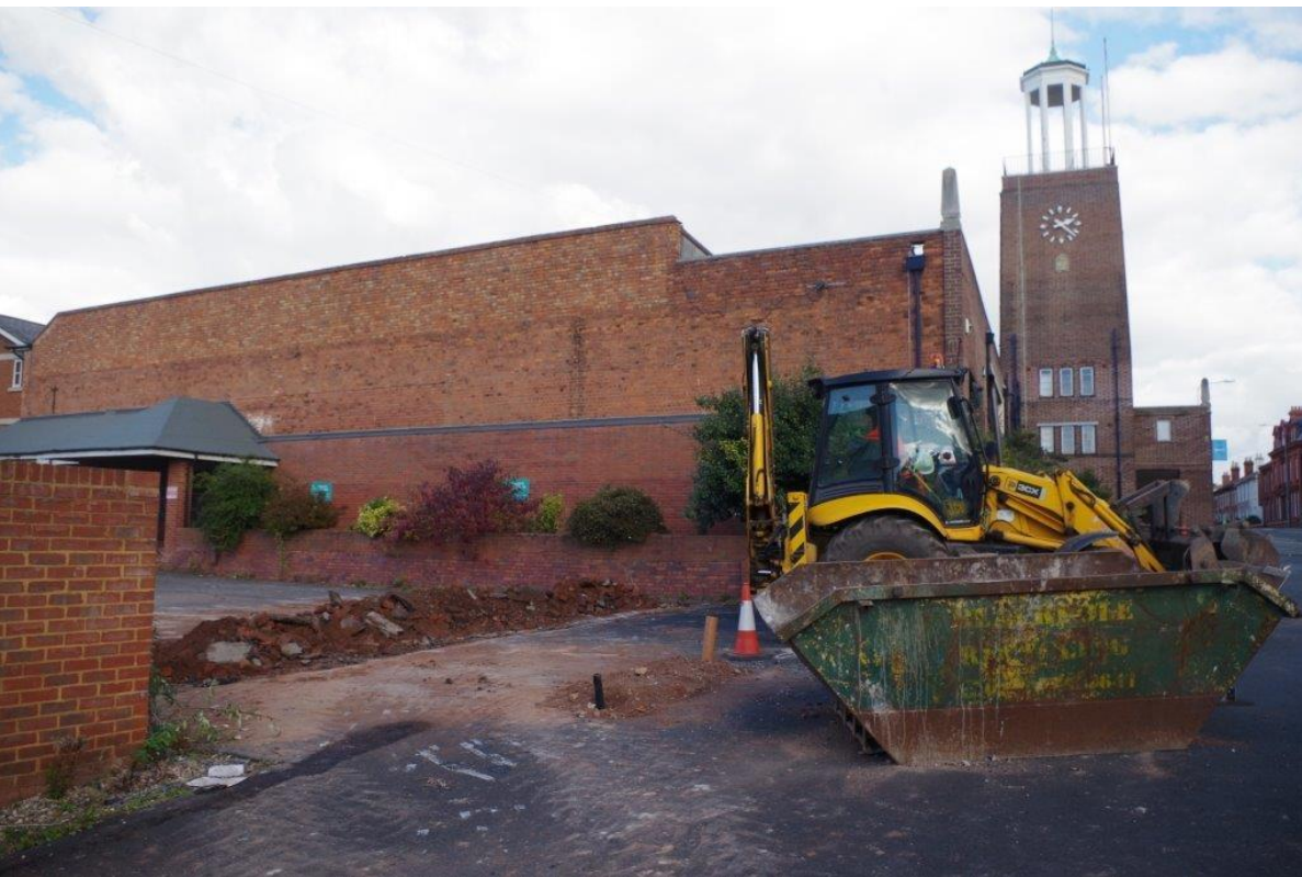
Plate 8 Location of Trench 2 and Test Pit 4 looking northeast after backfilling trenches
