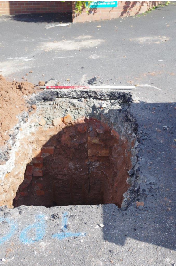
Plate 1 Brick wall of cellar in Test Pit 4
