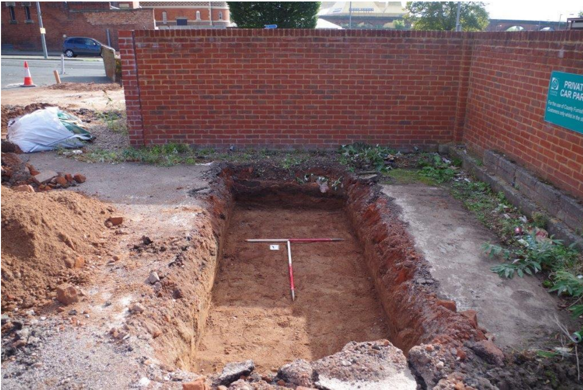
Plate 3 Trench 1 looking south after excavation
