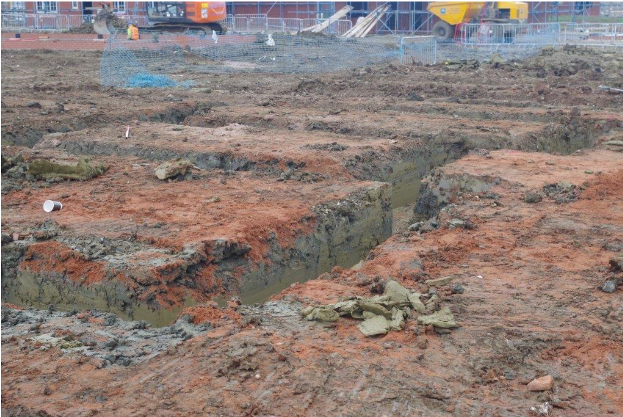
Plate 5: Plot 109 (western part of plot). Facing south-east
