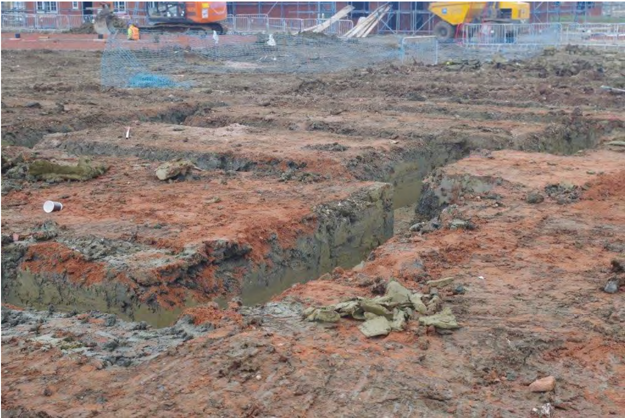
Plate 5: Plot 109 (western part of plot). Facing south-east
