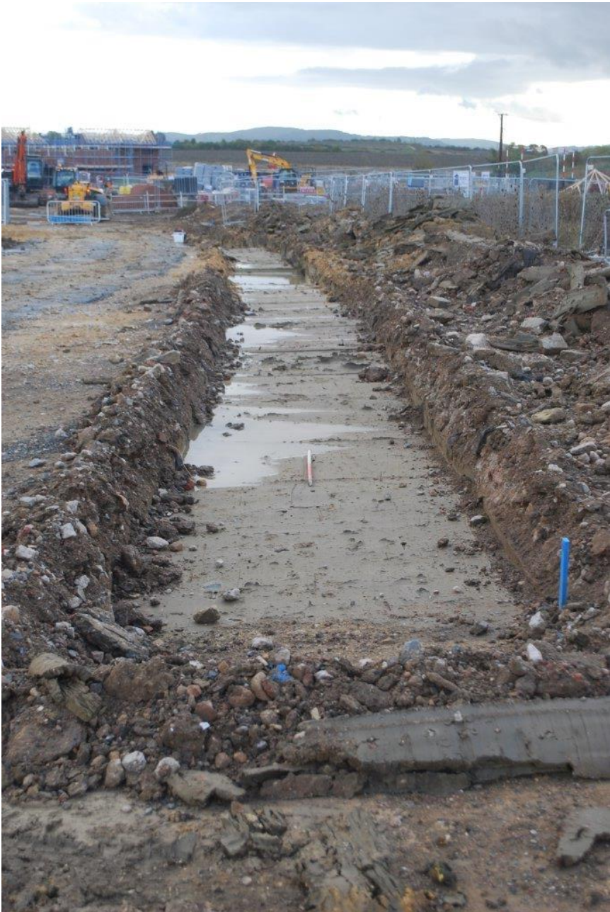
Plate 3: Trench 2. Facing south
