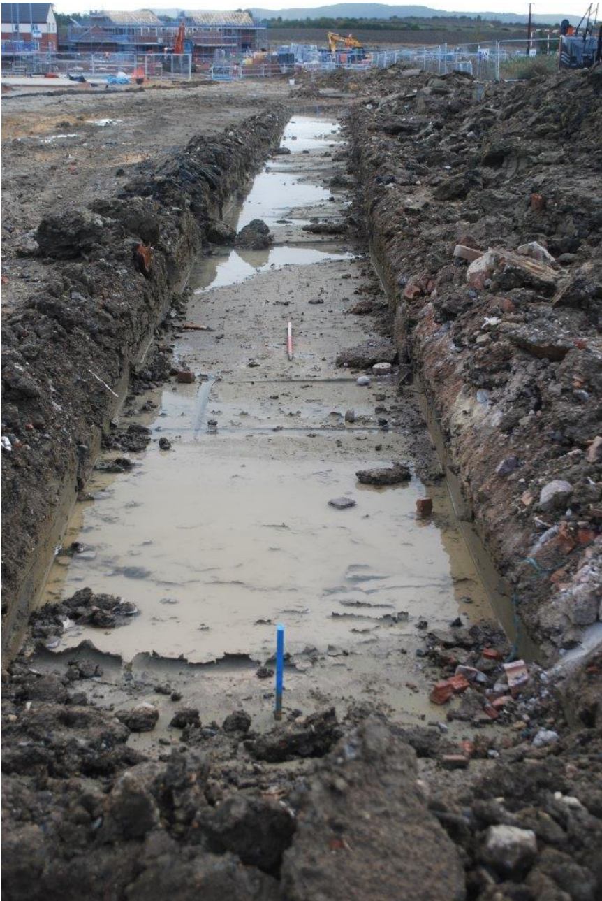
Plate 1: Trench 1. Facing south
