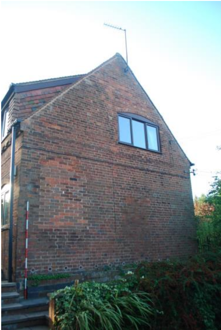
Plate 6 Phase 1 building, looking south
