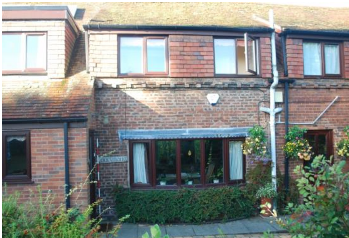
Plate 22 Phase 2 building, looking west
