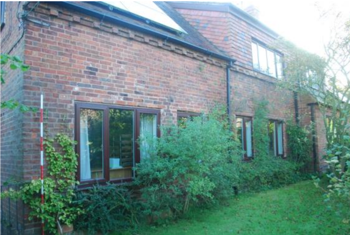
Plate 4 Former front of the Phases 1 and 2 buildings, looking south-east
