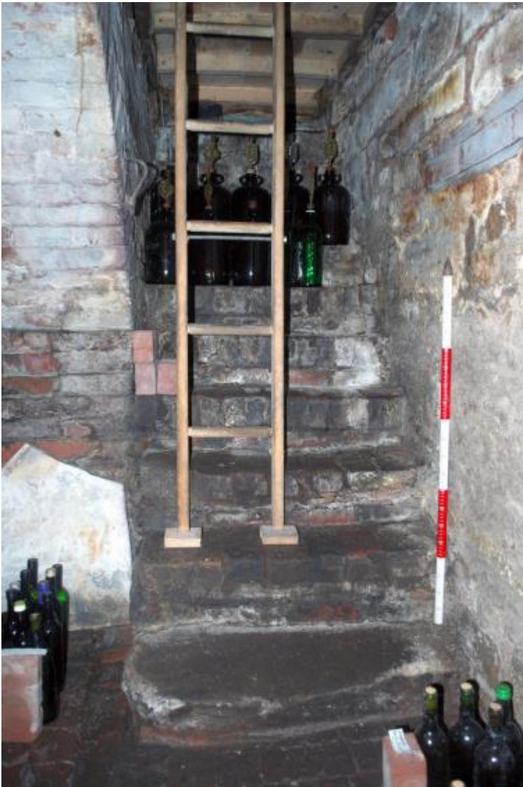
Plate 10 Phase 1 blocked cellar stairs, looking east
