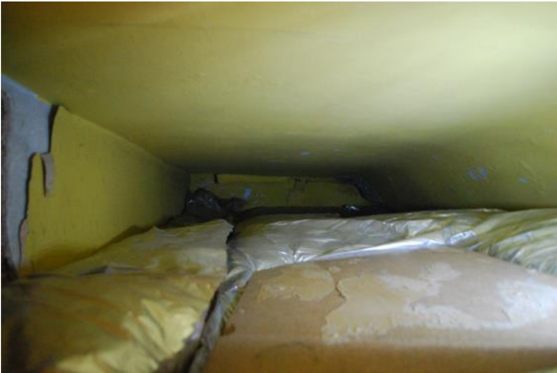
Plate 29 Phase 2 first floor room, looking south
