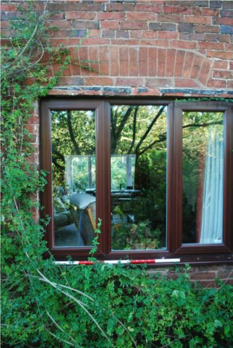
Plate 21 Phase 2 rubbed brick details of former window, looking east
