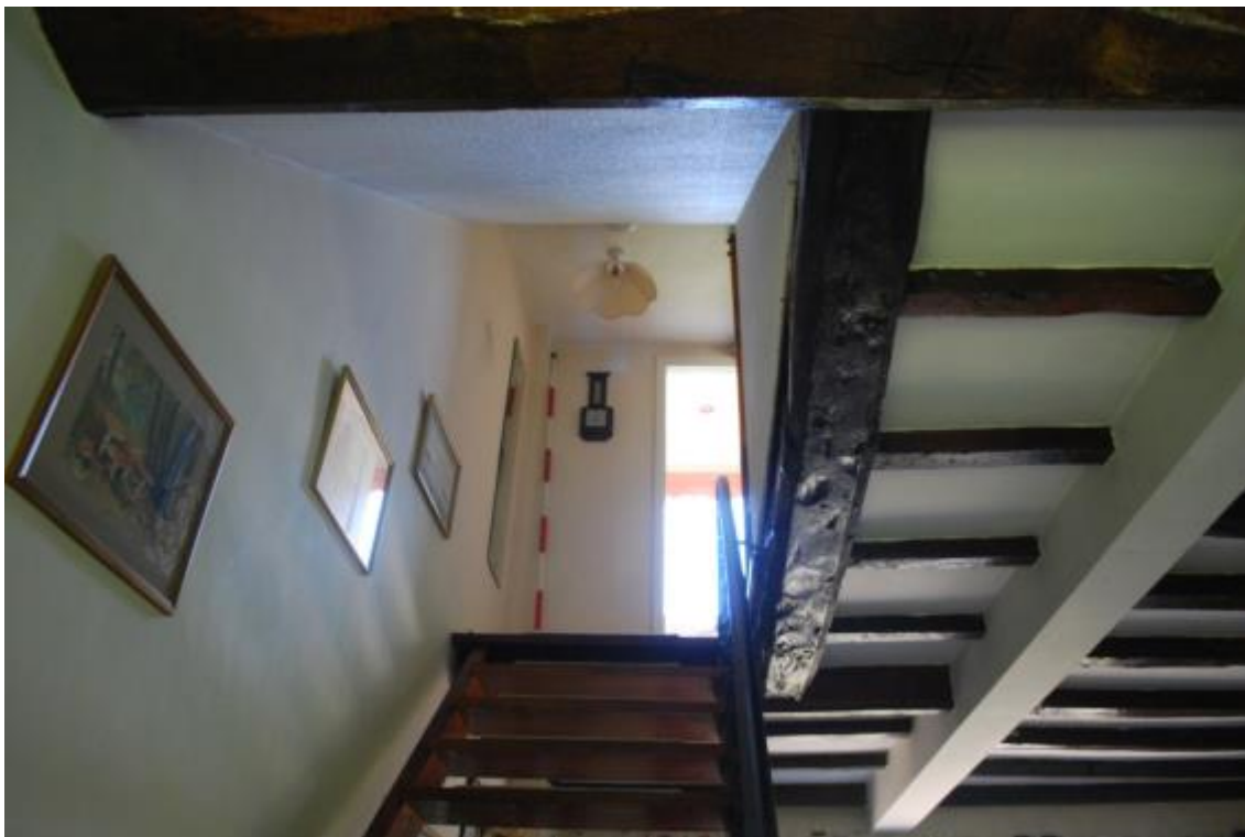
Plate 25 Phase 2 floor joists, looking east
