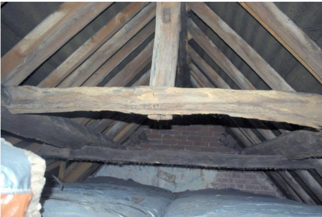
Plate 17 Phase 1 roof structure, looking south
