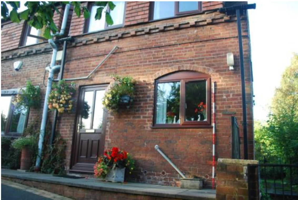
Plate 5 Phase 1 building, looking south-west
