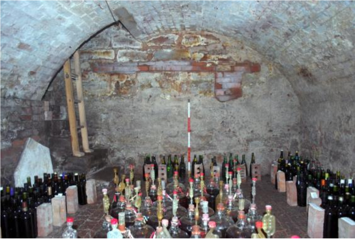
Plate 12 Phase 1 cellar, looking south
