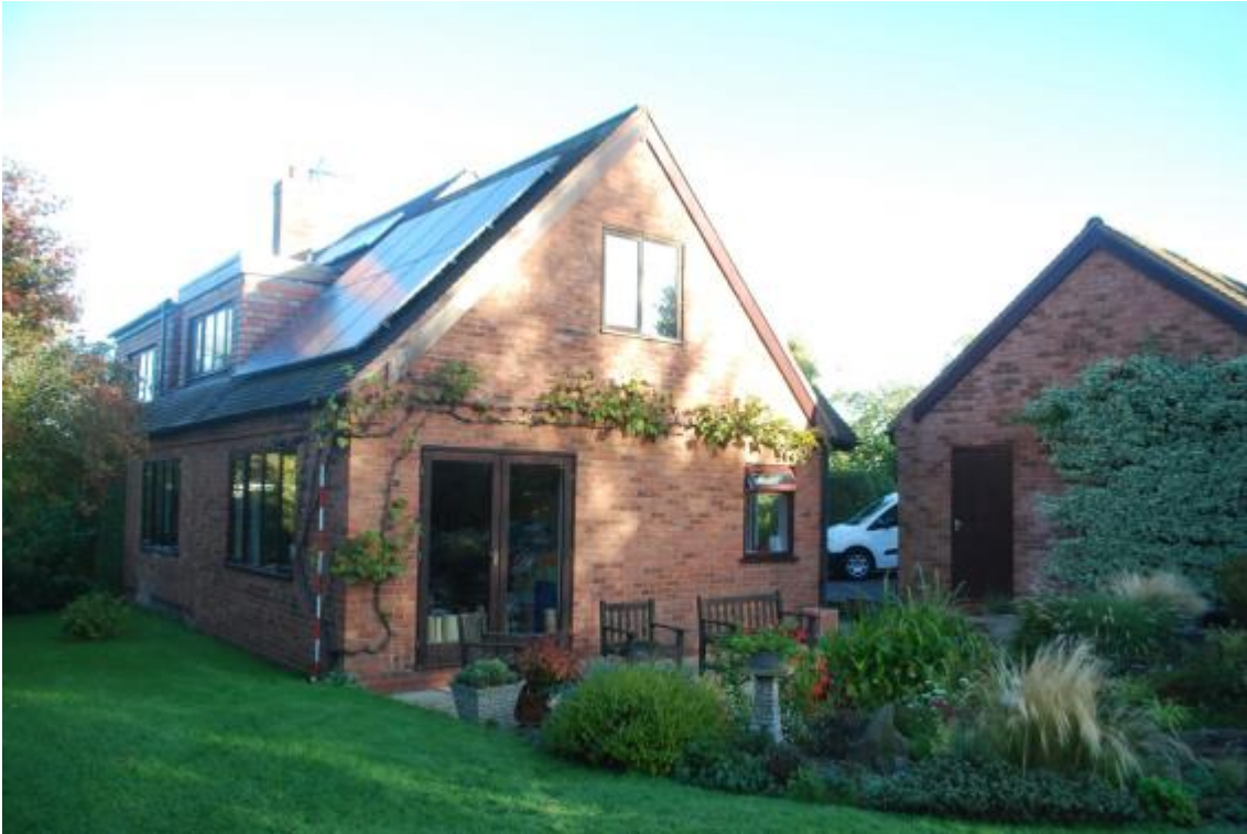
Plate 38 Phase 5 extension, looking north-east
