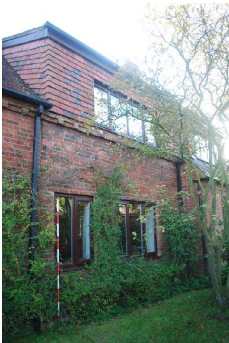
Plate 20 Phase 2 building, looking south-east
