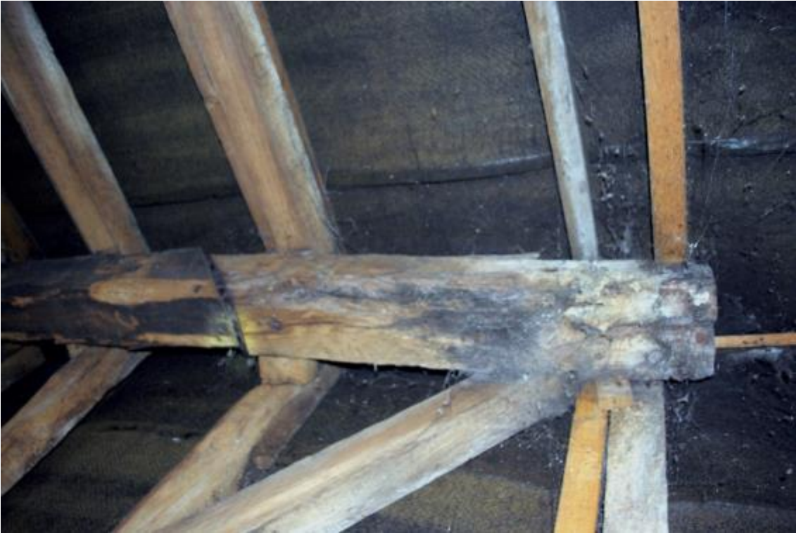
Plate 19 Phase 1 roof structure, looking upwards
