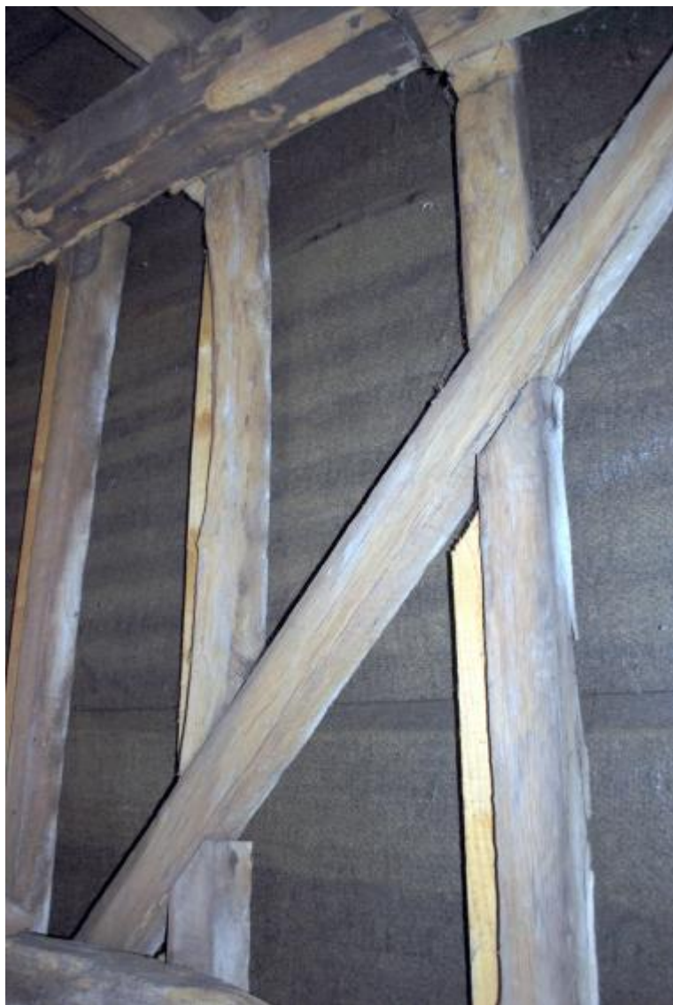
Plate 18 Phase 1 roof structure, looking south-west
