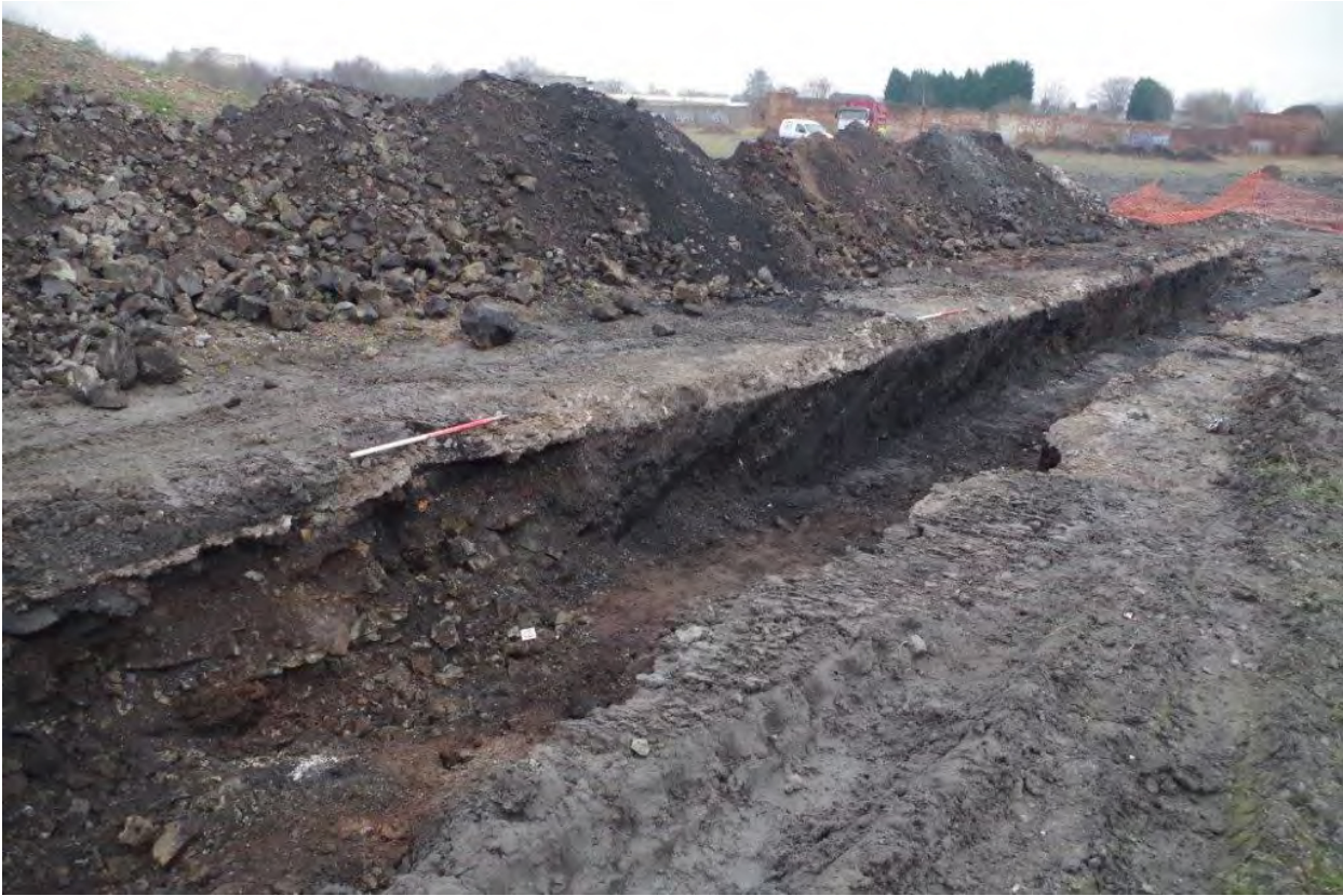
Plate 18 Trench 8, looking south-east (1m scales)
