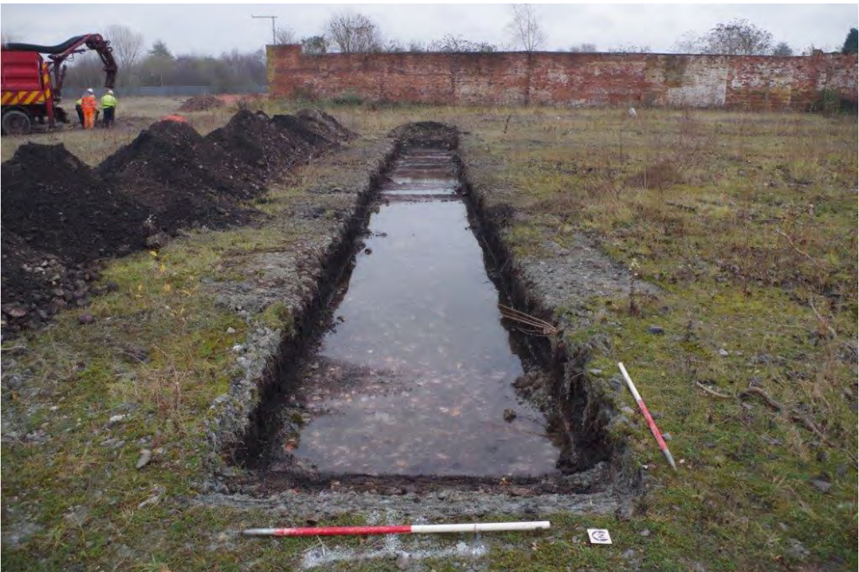
Plate 22 Trench 10, looking east (1m scales)
