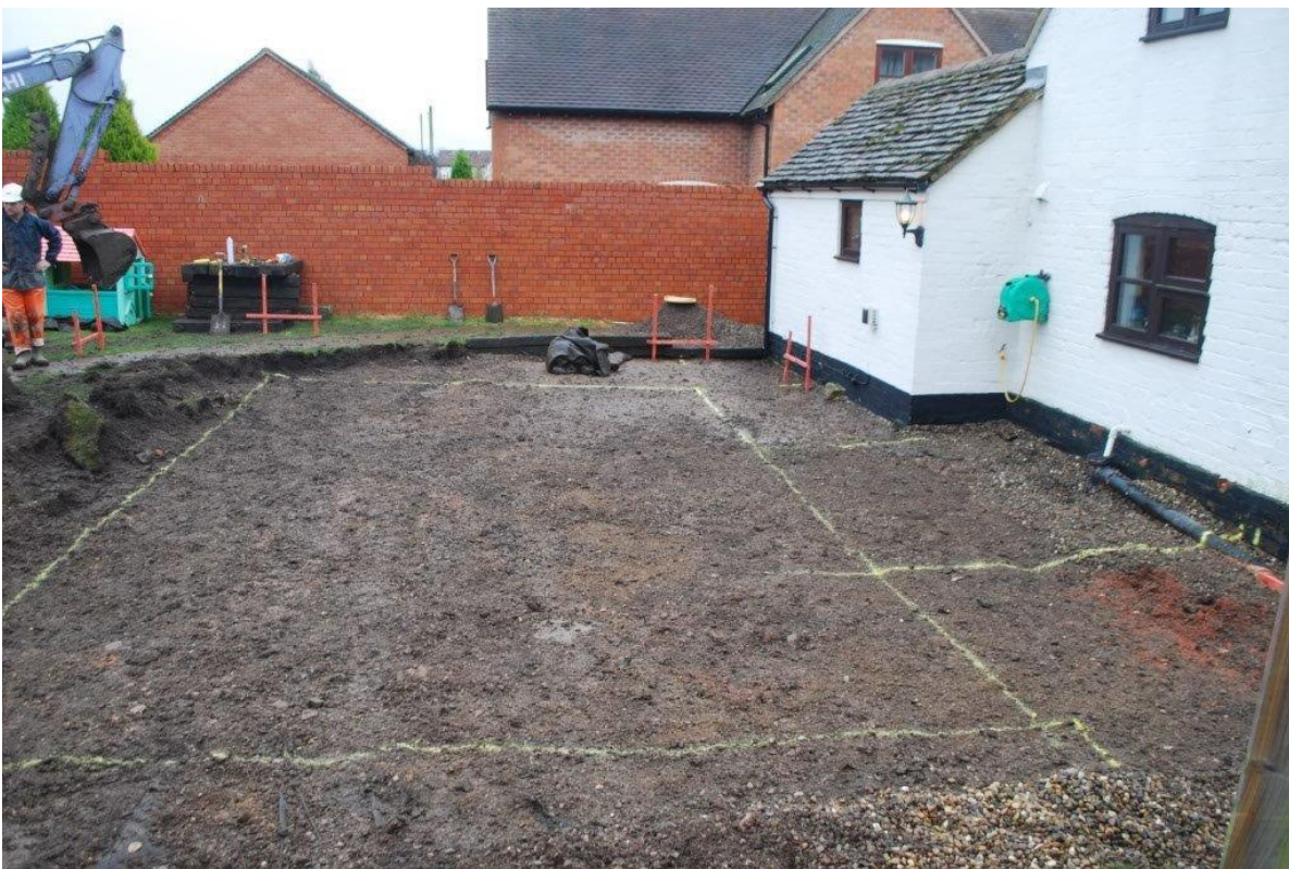
Plate 2 The site stripped of modern surfacing and topsoil, view east
