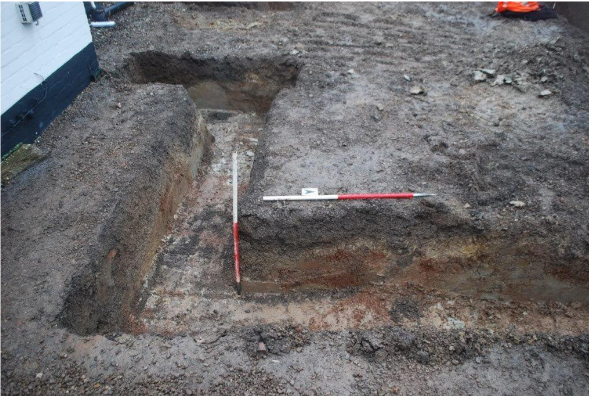
Plate 3 The southeastern corner of the foundations, showing natural gravels and marl. View west
