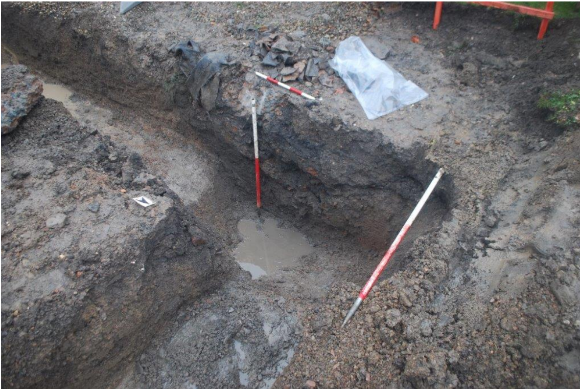
Plate 7 Full extent of pit exposed in Northwestern corner of site foundations.
