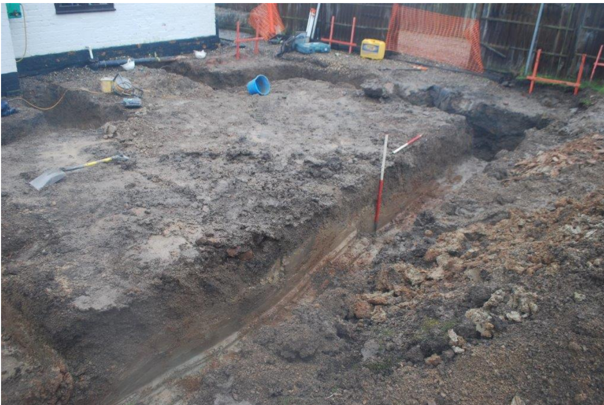
Plate 8 Foundation trenches after excavation. View southwest.
