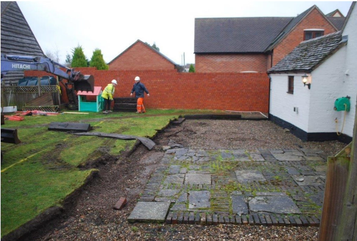
Plate 1 The site prior to excavation works, view east
