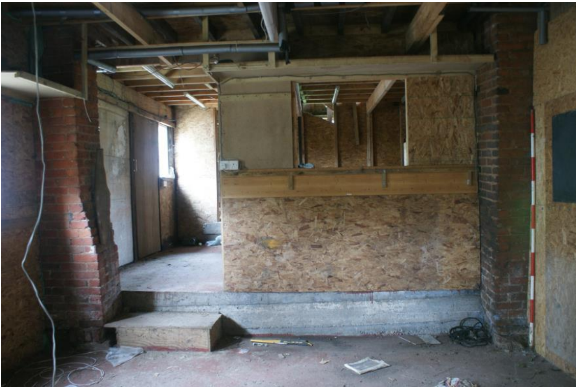
Plate 3 Toll Barn interior, looking north-east
