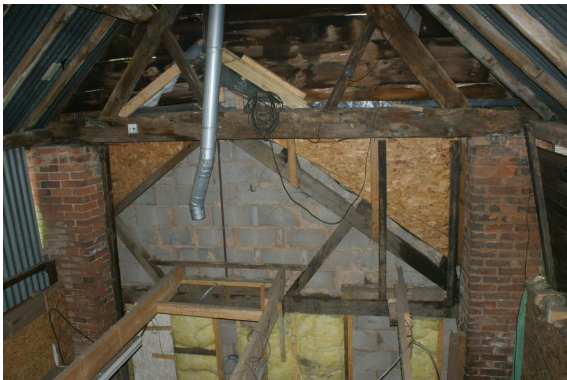
Plate 11 Phase 2 king post type truss, looking south-west
