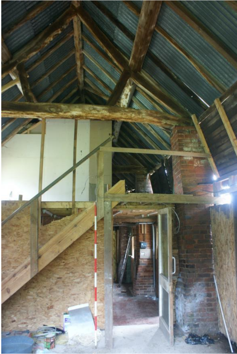
Plate 4 Toll Barn interior, looking south-west
