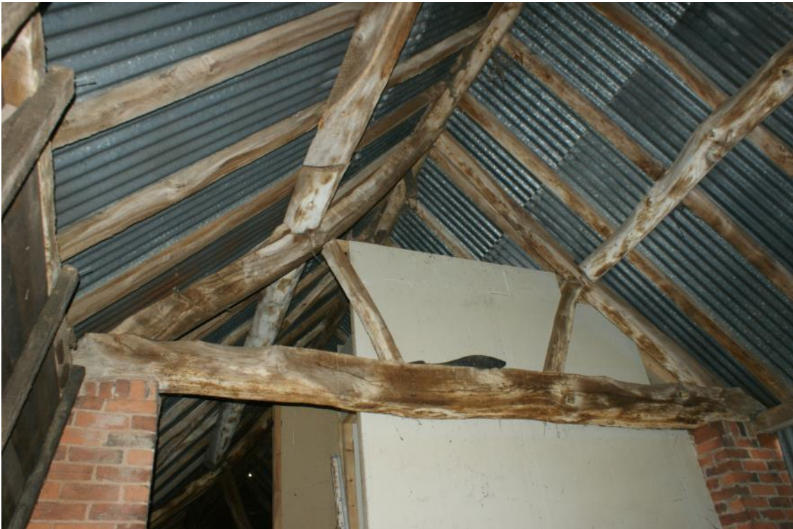
Plate 6 Roof truss, looking north-east
