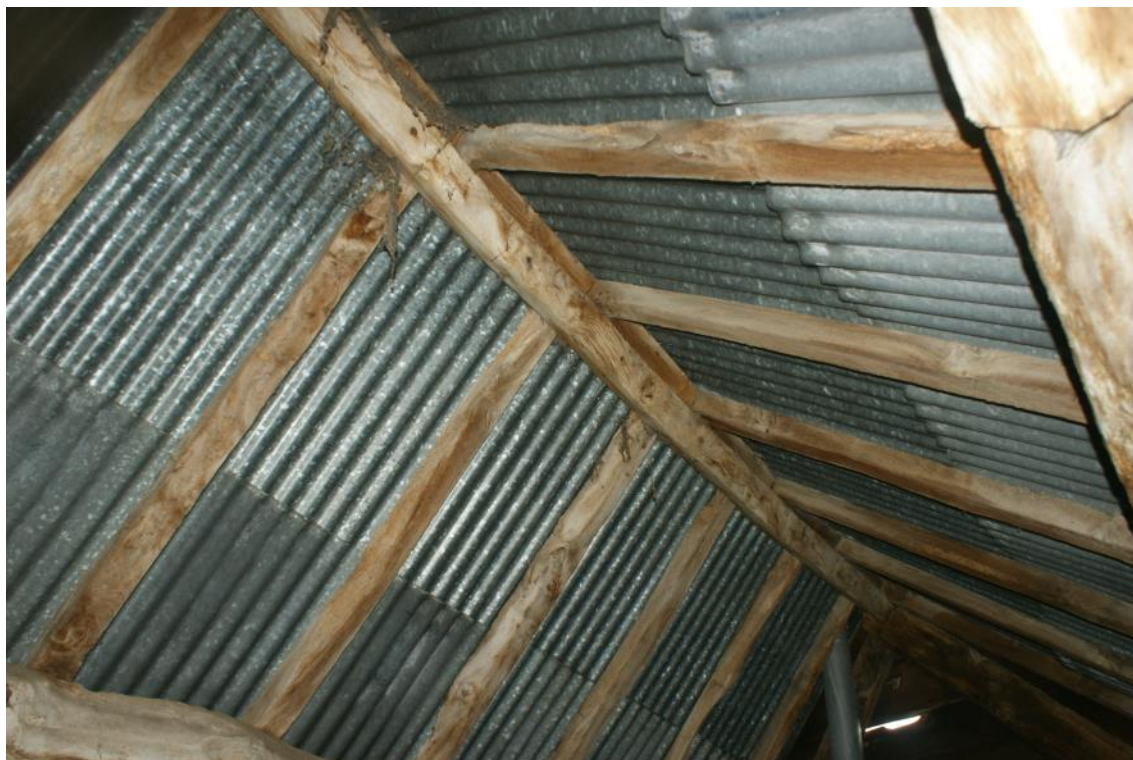
Plate 10 Peg holes visible within the ridge purlin, looking south-west
