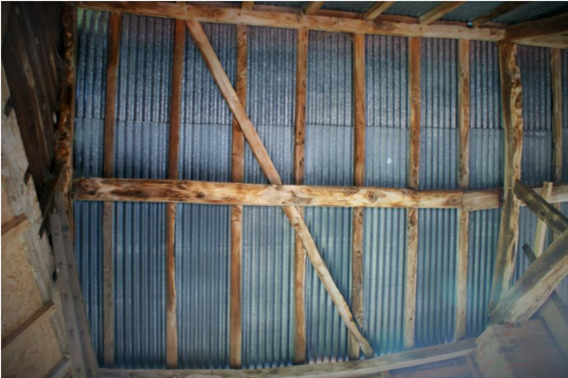
Plate 7 Roof structure, looking south-east
