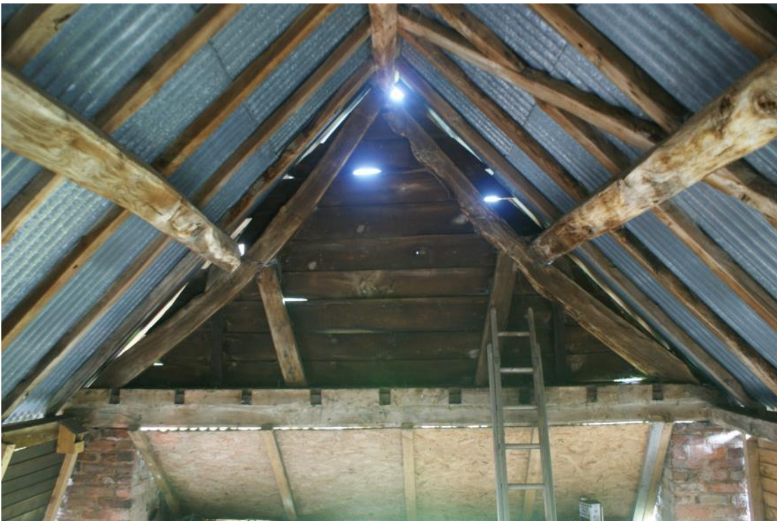
Plate 9 Reused timber as part of a tie beam, looking north-east
