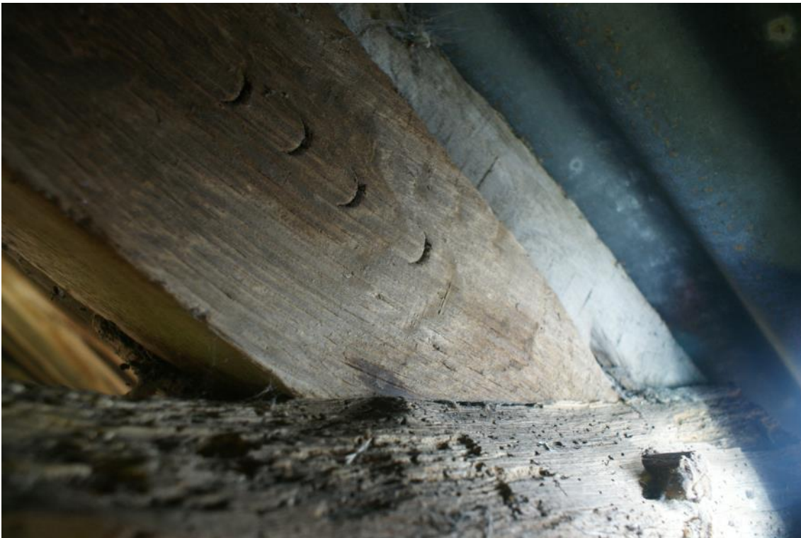
Plate 8 Carpenters marks and pegging, looking north-east
