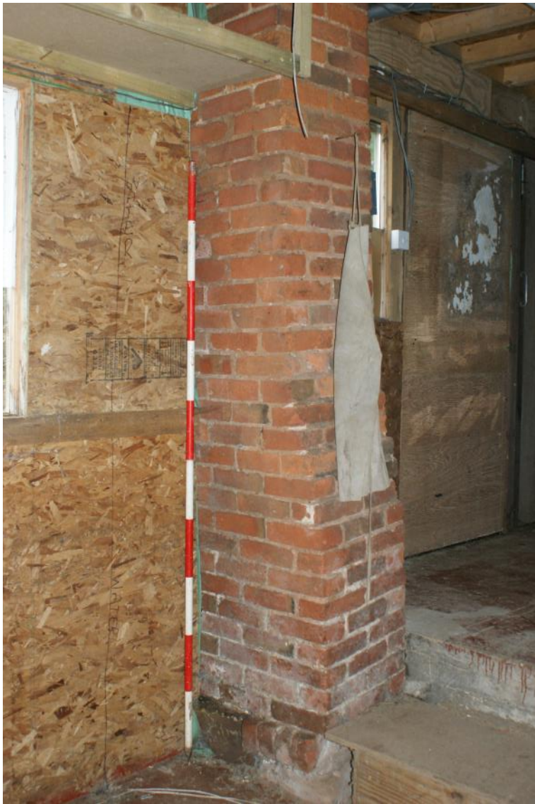
Plate 5 Brick pillar with sandstone base, looking north
