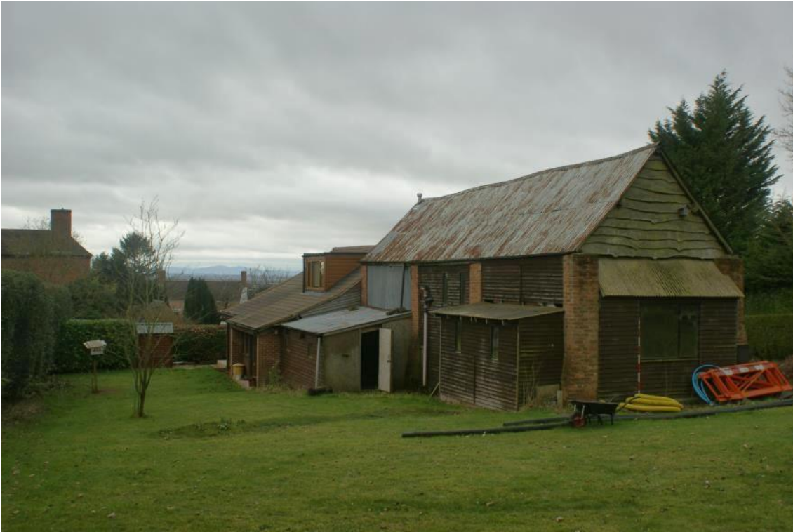
Plate 1 Toll Barn exterior, looking west
