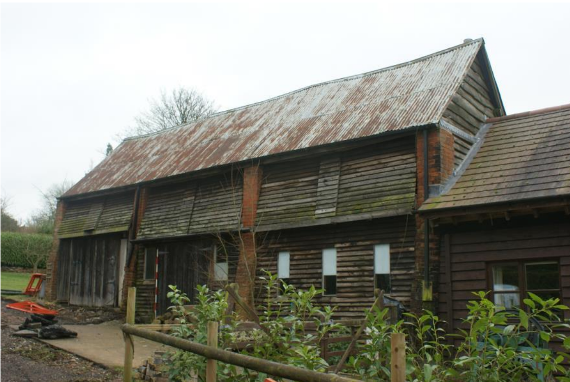
Plate 2 Toll Barn exterior, looking east
