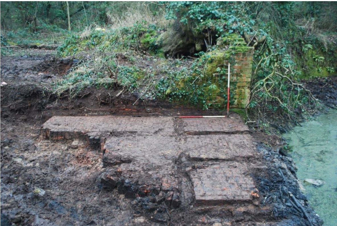
Plate 4 Sluice [100], with slots for wooden beams; view east; 2x 1m scales
