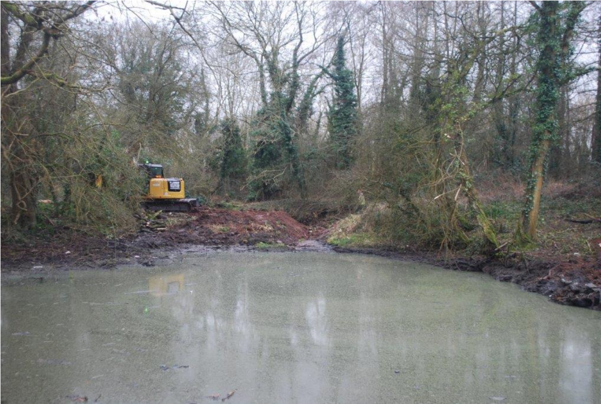
Plate 7 South outlet after de-silting and re-profiling; view south; no scales
