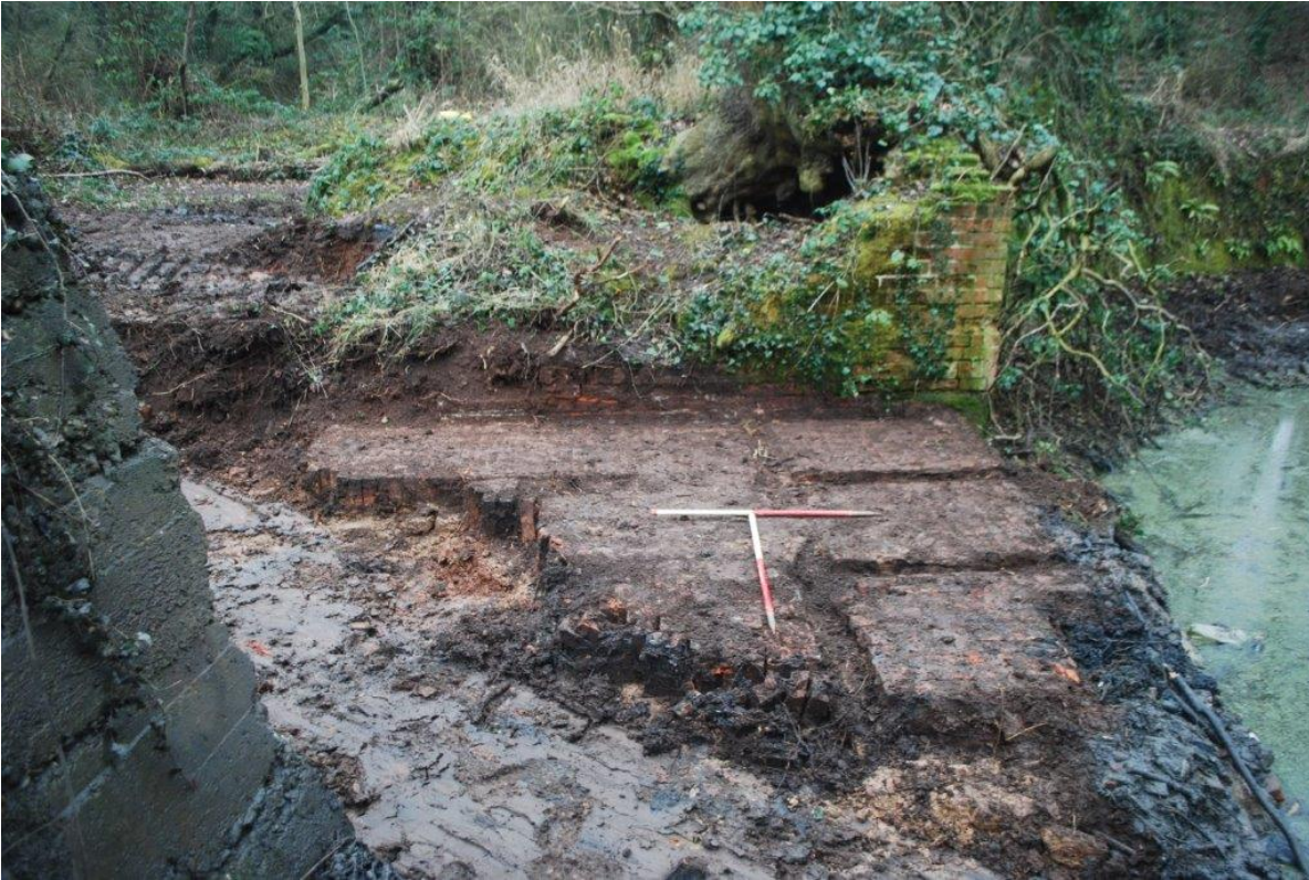
Plate 3 Sluice [100], with slots for wooden beams; view east; 2x 1m scales
