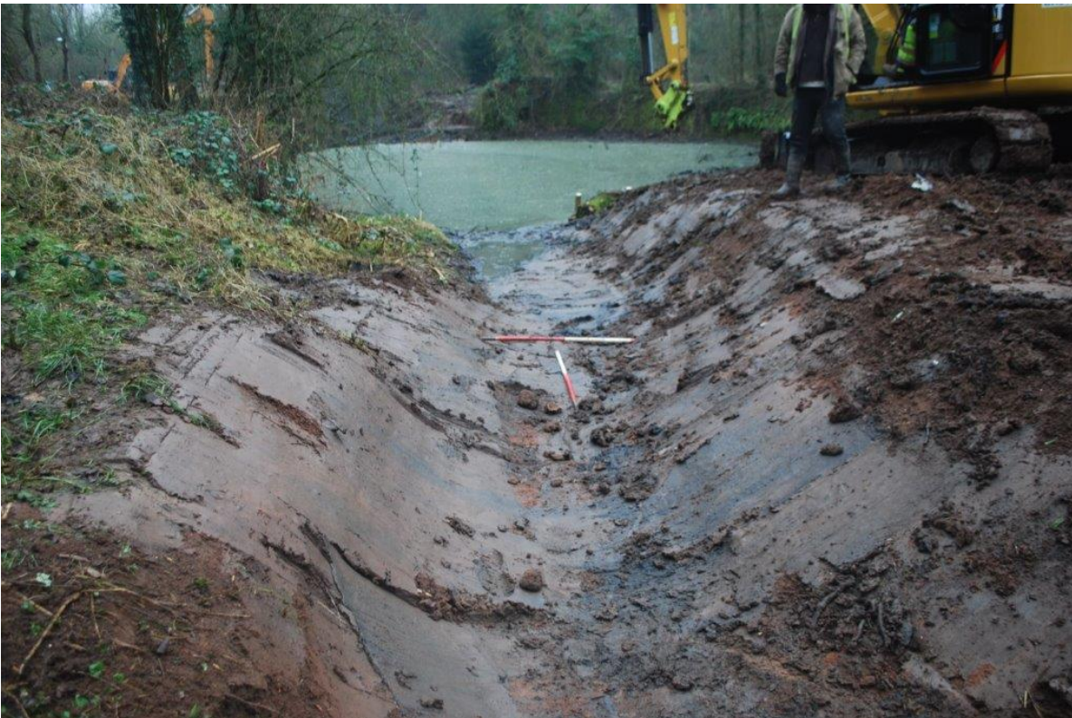
Plate 8 The re-profiled south outlet; view north; 2x 1m scales
