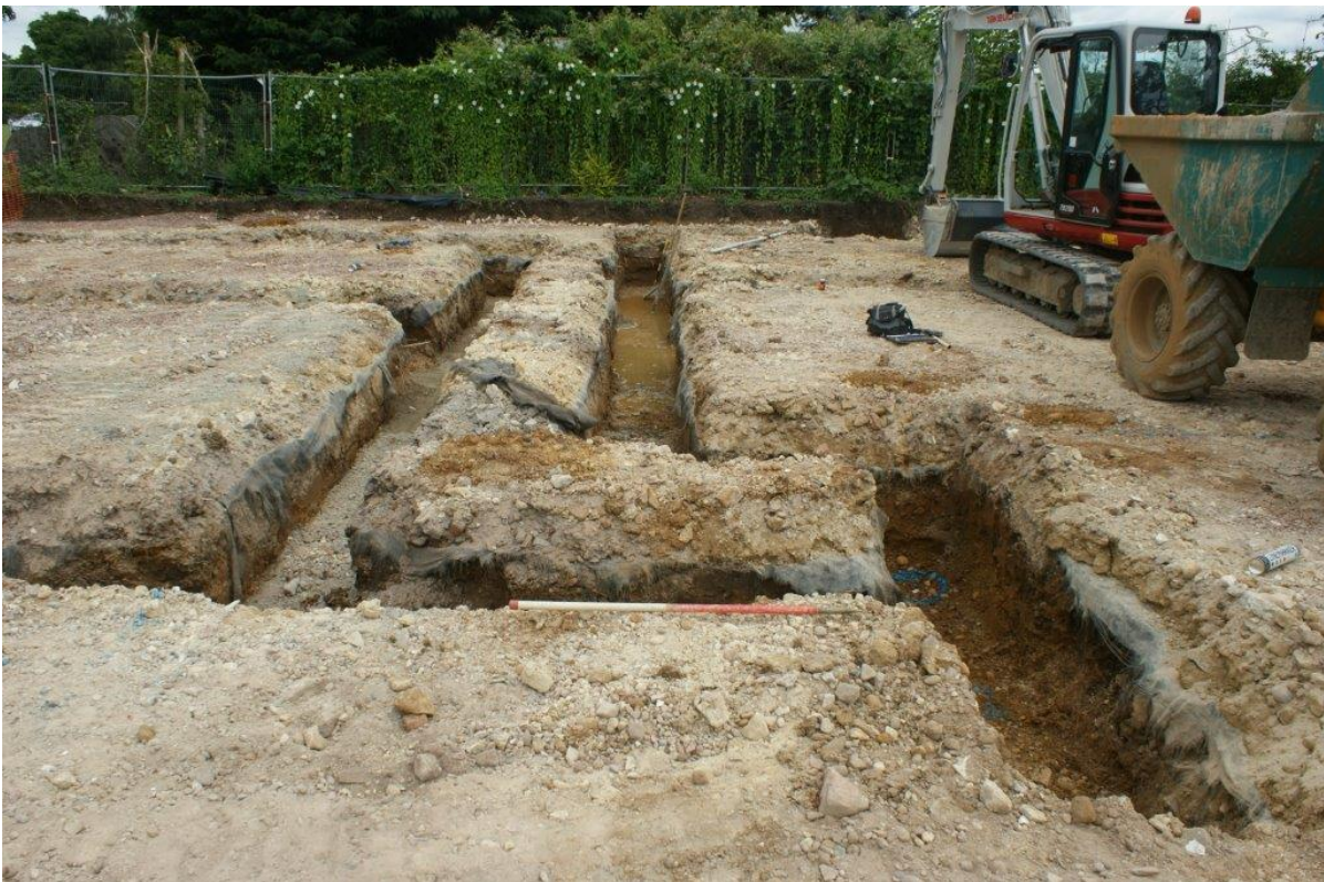
Plate 4 Trench 2 footings showing natural sand and gravel. 1m scale, view south
