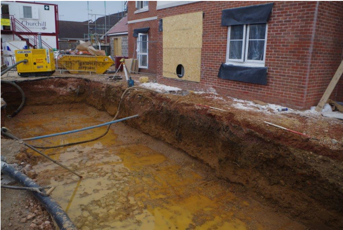
Plate 5 The attenuation tank (trench 3) view northeast
