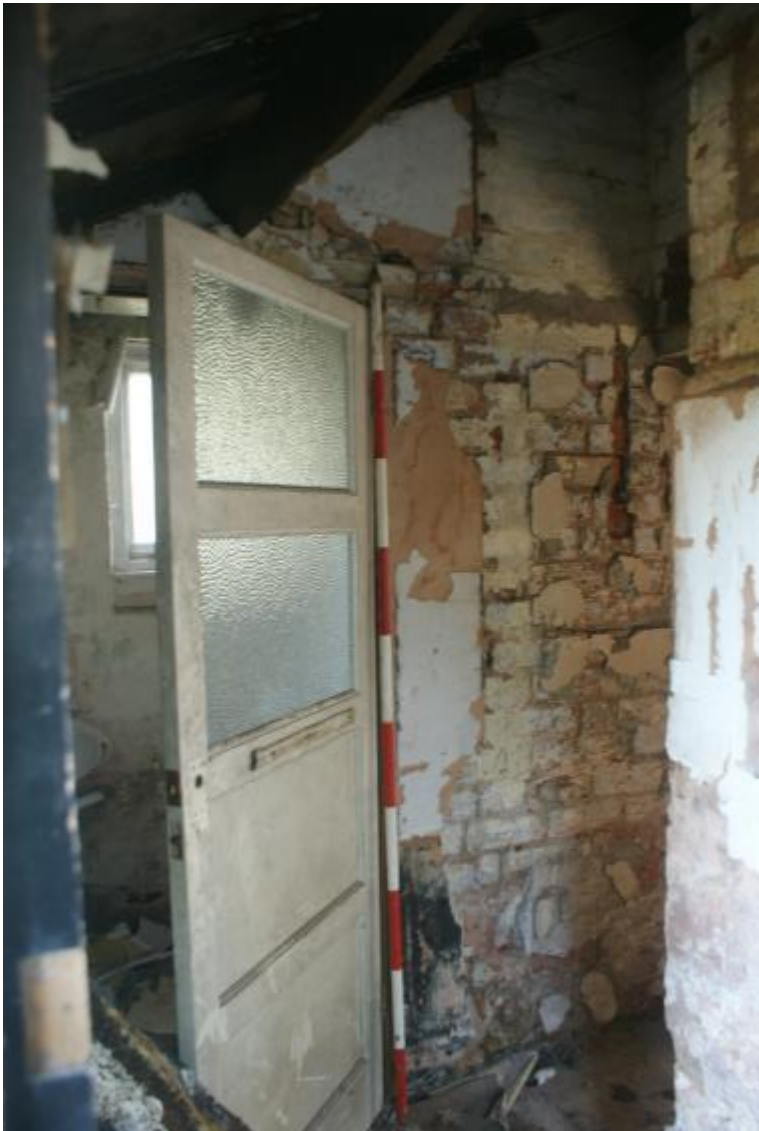
Plate 17 Phases 6 and 7 extension, looking south
