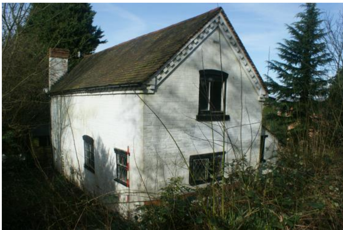
Plate 2 The building, looking north
