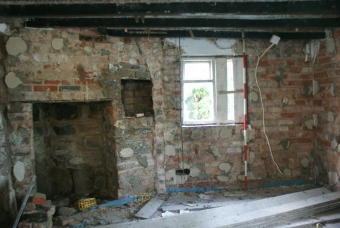
Plate 11 Phase 4 brickwork with Phase 5 fireplace, looking north-west
