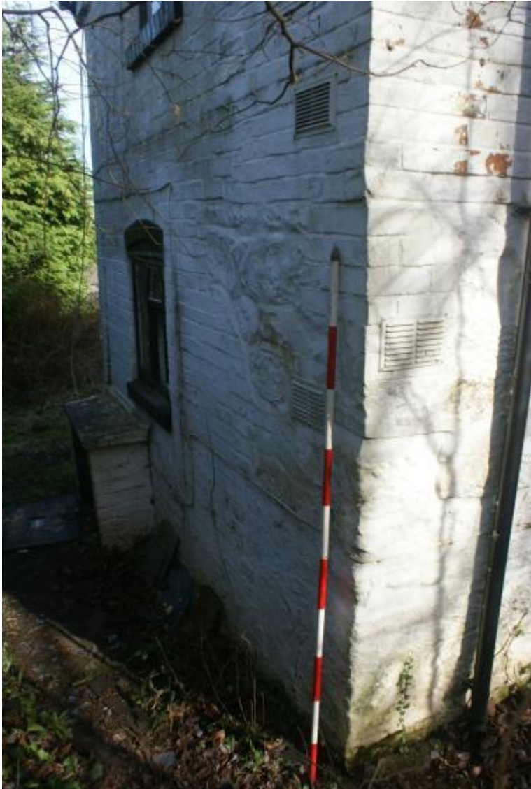
Plate 10 Phase 3 gable window, looking east
