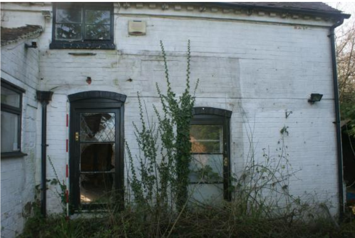
Plate 8 Phase 3 brickwork, looking south-west
