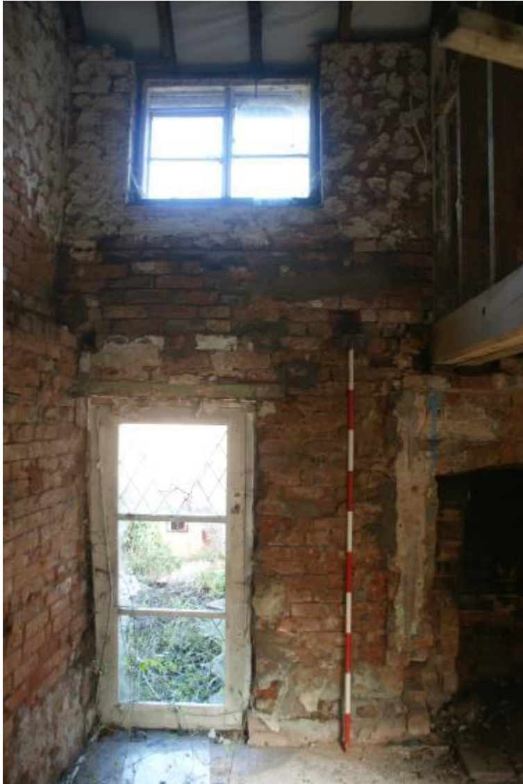
Plate 9 Phase 3 brickwork, looking north-east
