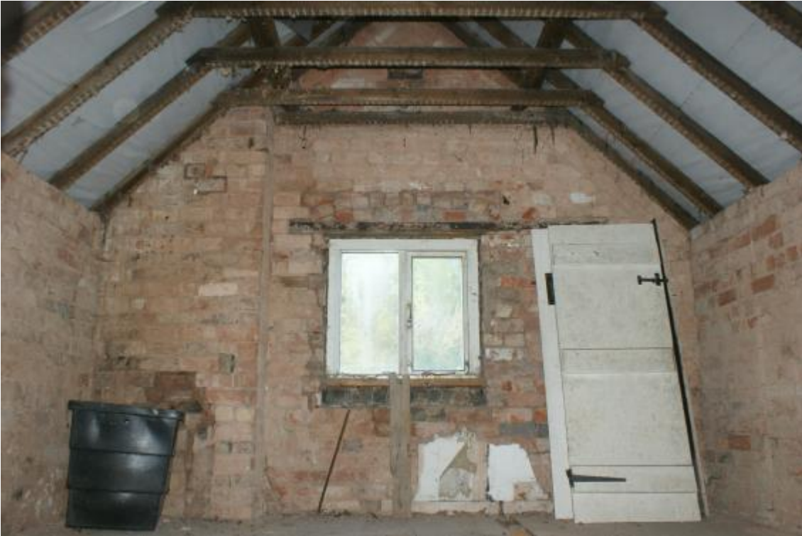
Plate 14 Phase 5 first floor room and roof structure, looking north-west
