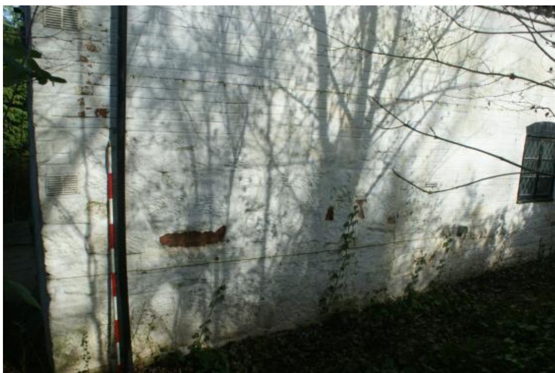
Plate 4 Phase 1 stonework, looking east
