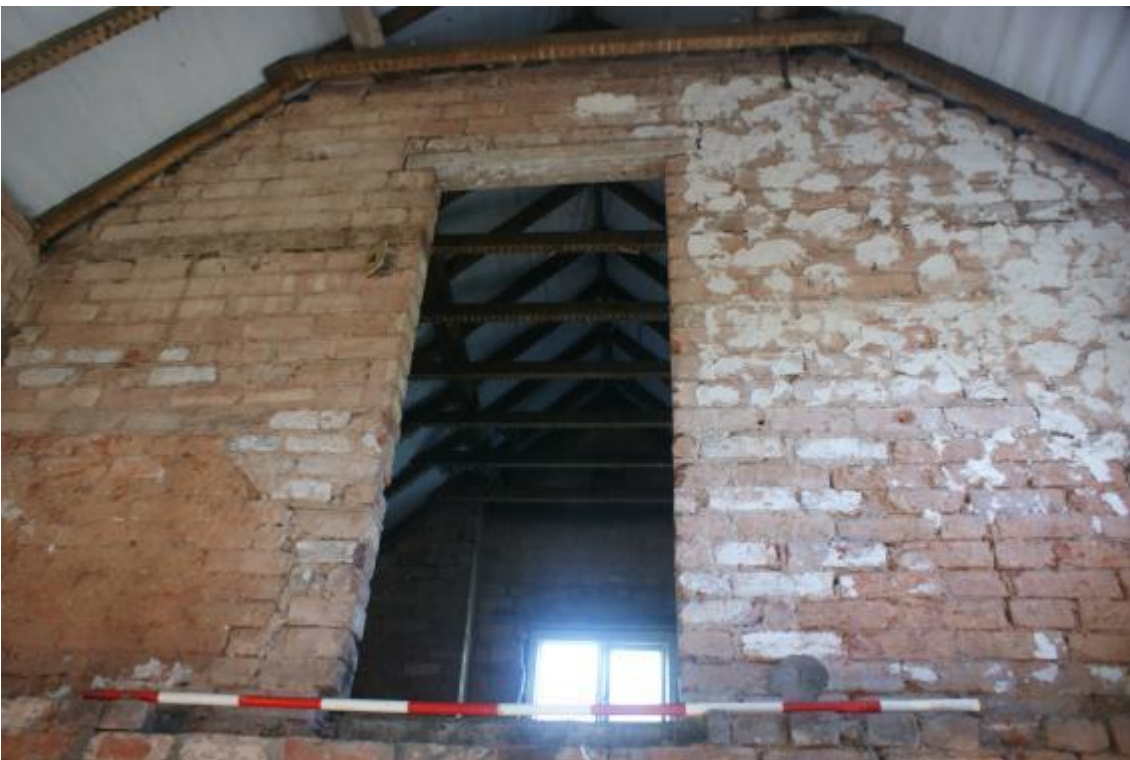
Plate 15 Phase 5 first floor doorway, looking north-west
