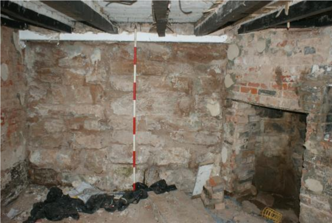
Plate 7 Phase 1 stonework with Phase 2 blocking stonework, looking south-west
