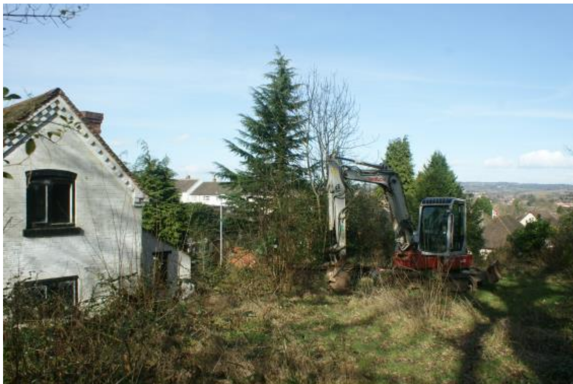
Plate 3 The building, looking north-east
