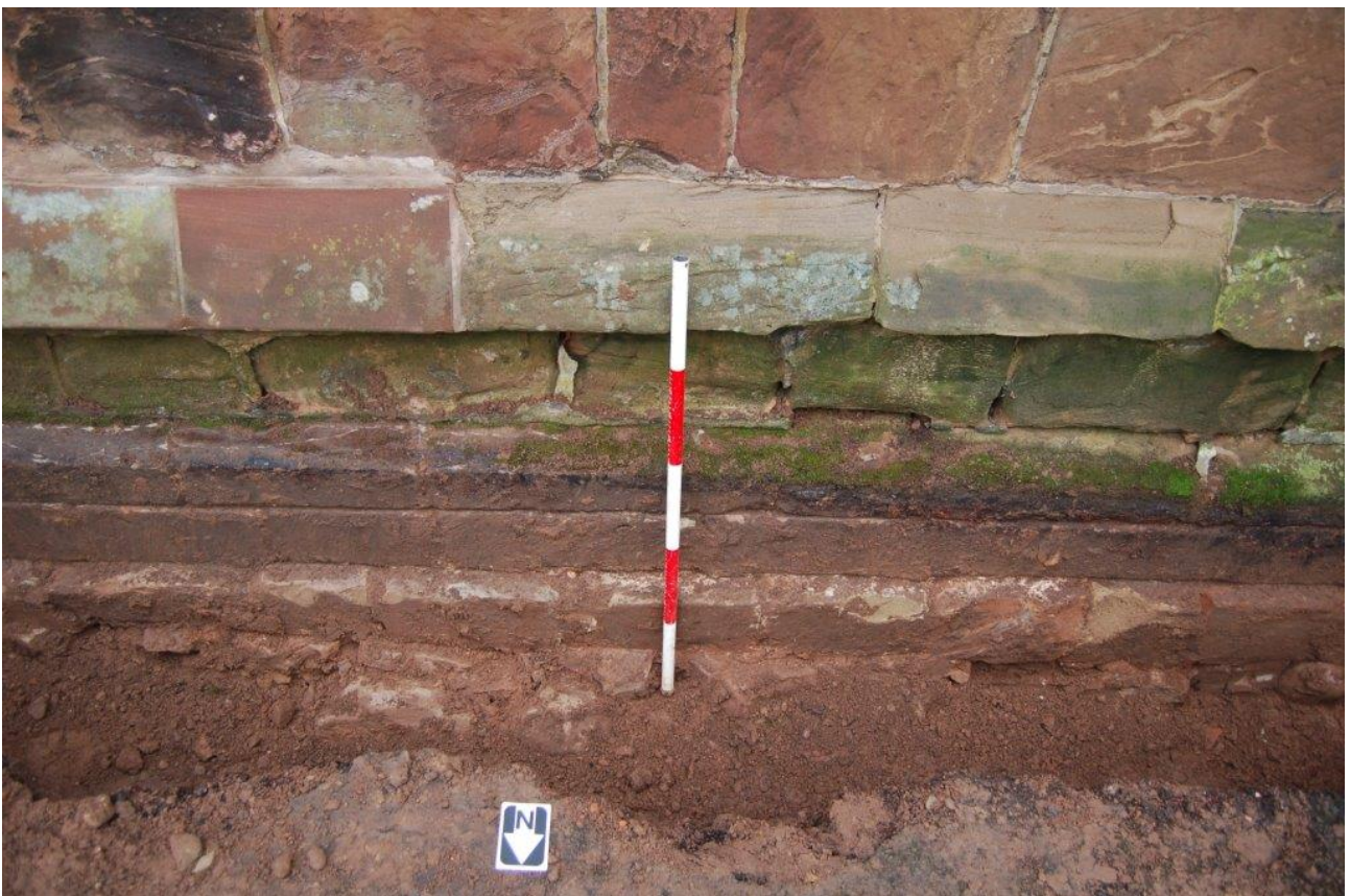
Plate 3: Wall (107) and foundation rubble (108) in bay 4, 1m scale
