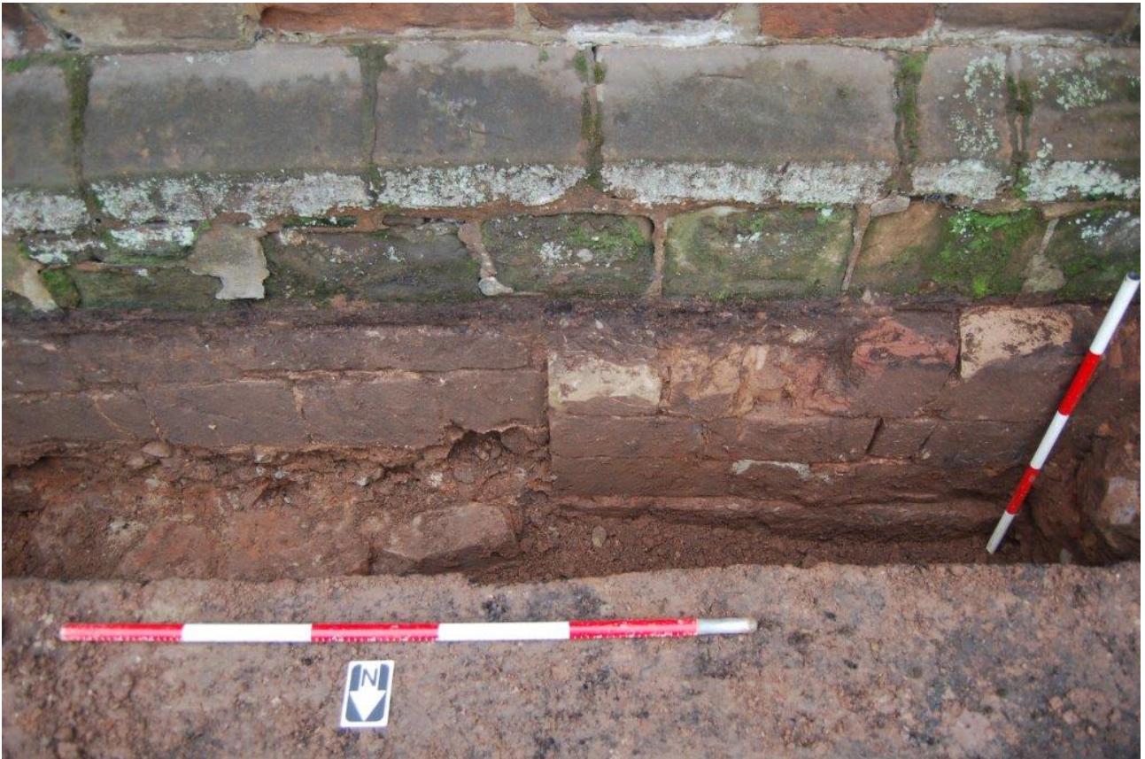
Plate 2: Northern transept wall (110) in the western side of bay 2, 2x1m scales
