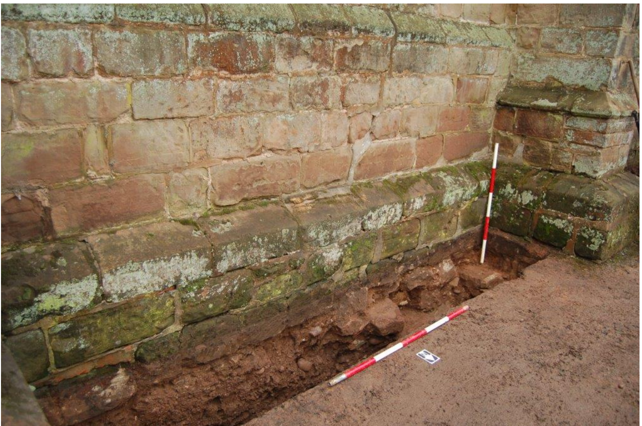
Plate 5: Wall (106) and foundation rubble (109) in bay 1, 2x1m scale
