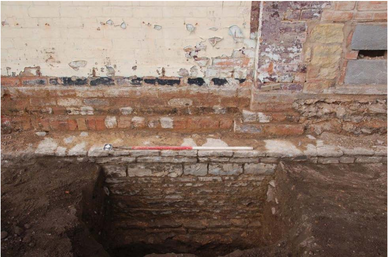
Plate 13, Abbot Chryton's wall with boundary wall of No.44 Merstow Green built above, view north, 1m scale
