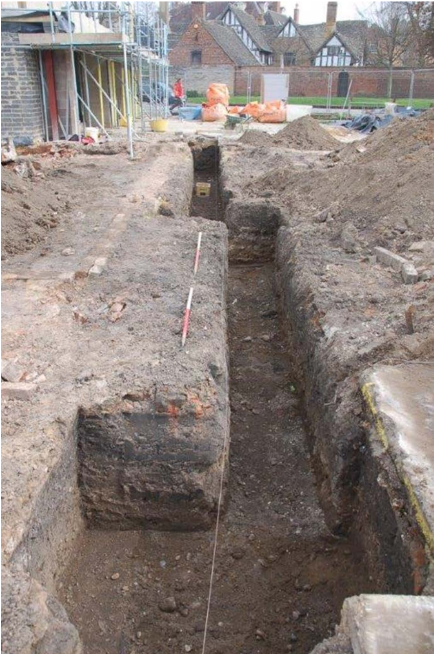
Plate 5, Strip foundation trench, view east, 2x 1m scales
