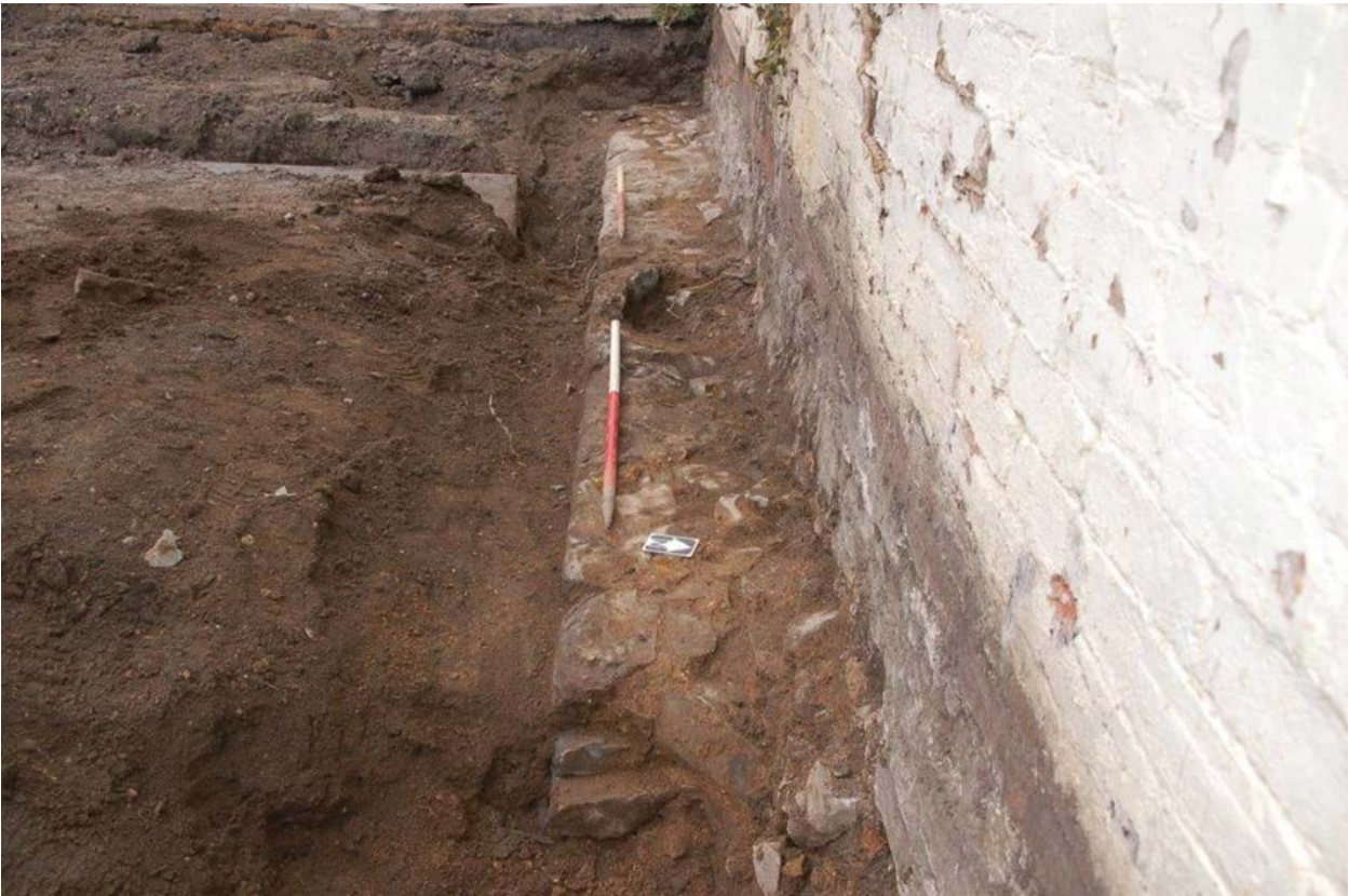
Plate 17, Abbot Chryton's wall at west of site, view west, 2x 1m scales
