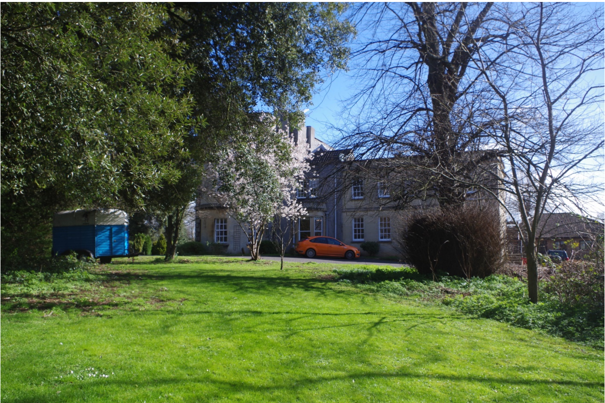
Plate 2: Warmley House (SGHER 1432) with screening vegetation to west – photograph facing east
