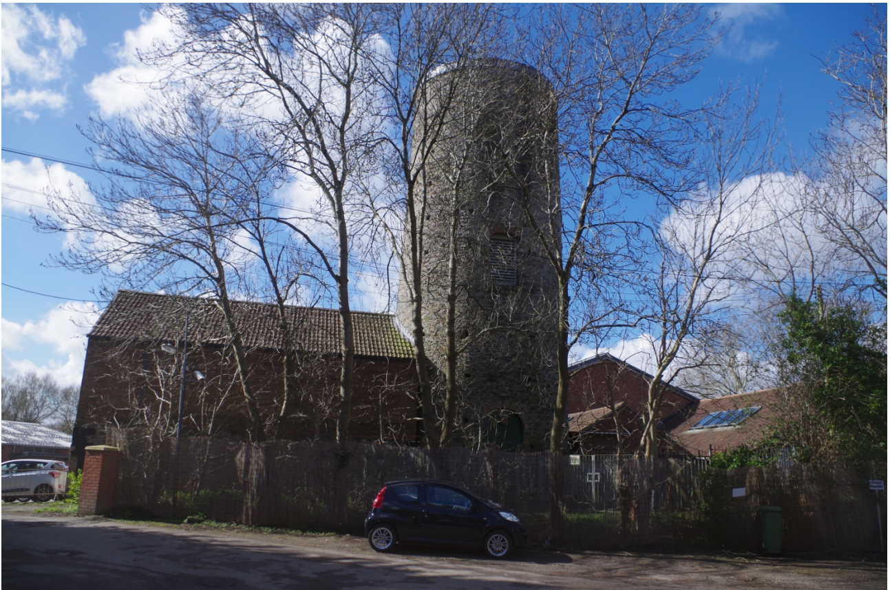
Plate 4: Windmill tower (SGHER 1430) as seen from site – photograph facing south-west
