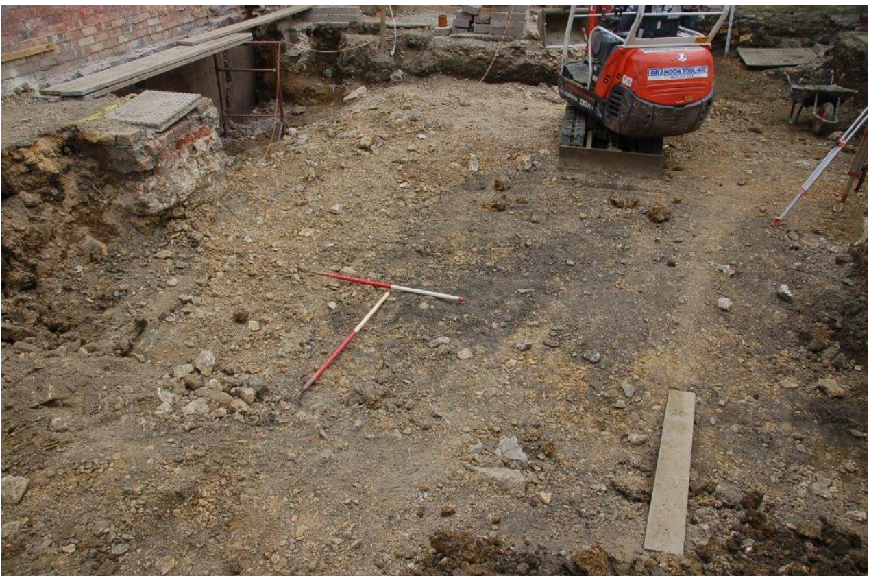
Plate 6 The excavated trench, natural 103 in base, view south-east, 2x 1m scales
