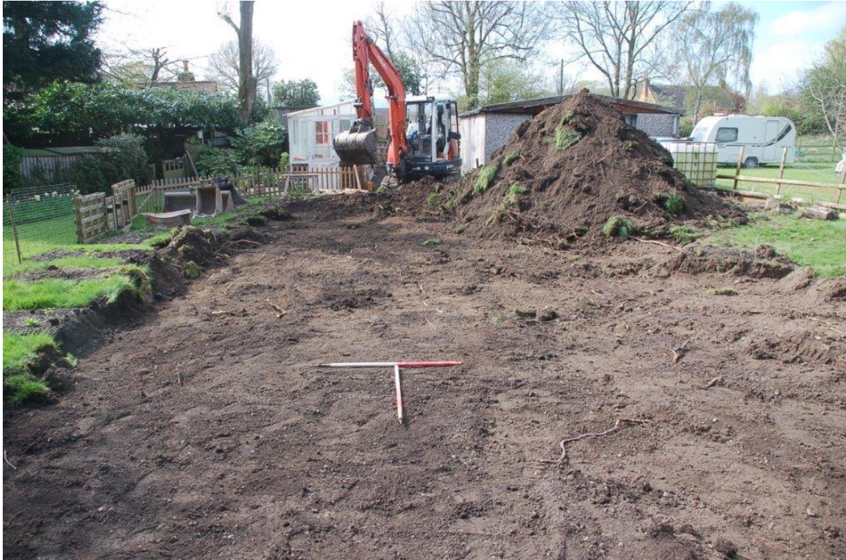
Plate 1. Topsoil strip of the development area. View west. Scales 1m.
