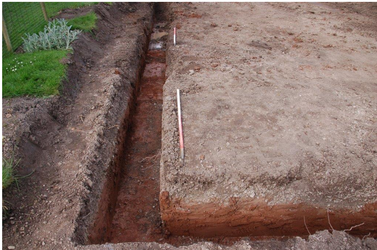
Plate 2. Strip foundation trench in south-east corner. View west. Scales 1m.
