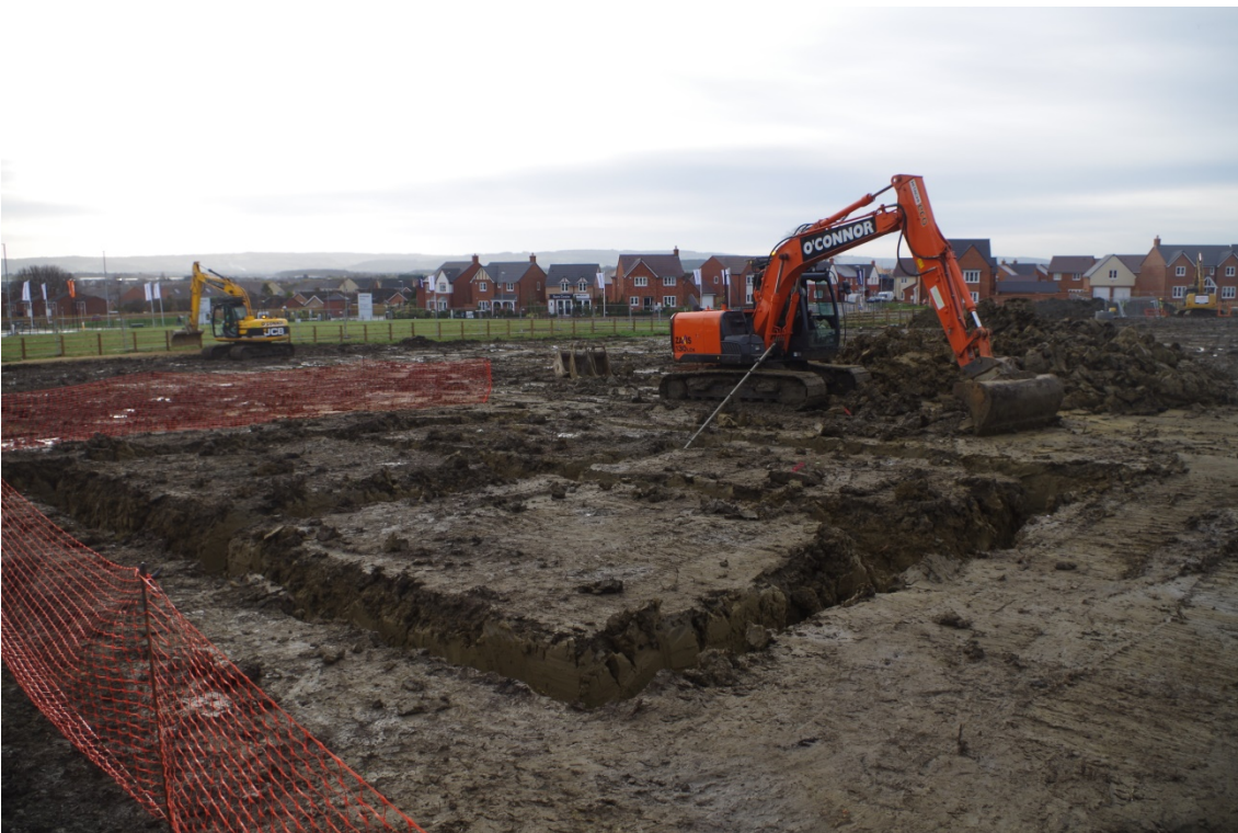
Plate 2 Trench 2 house foundations, looking south-east
