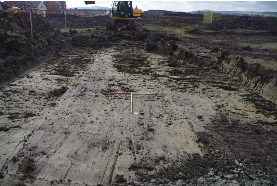
Plate 1 Trench 1 access strip, looking south
